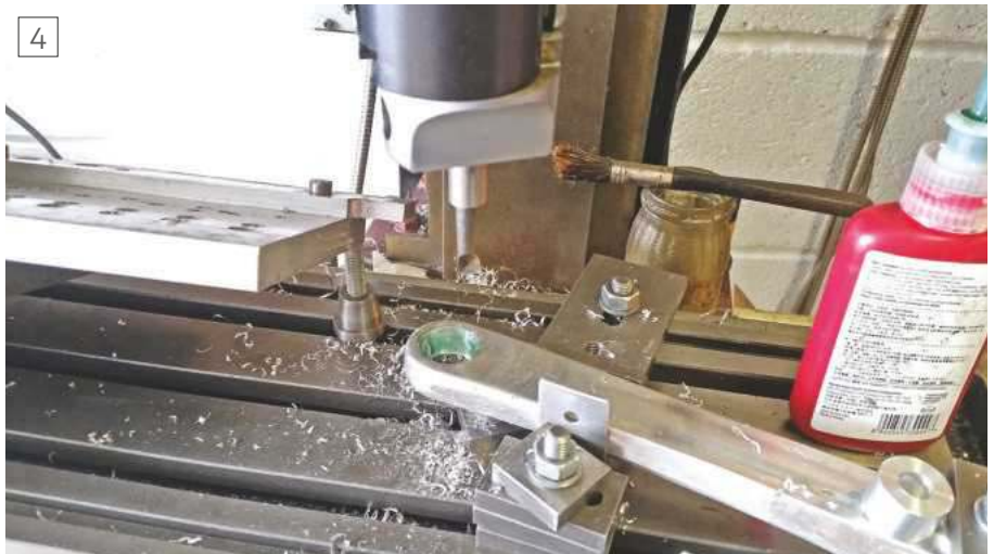
Applying the retaining compound to the bore.
