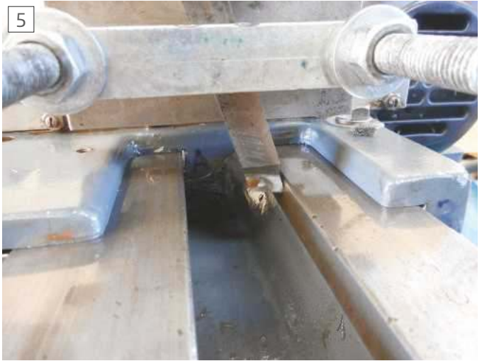
Sharpened tool bit is set on the most worn section of shear.
