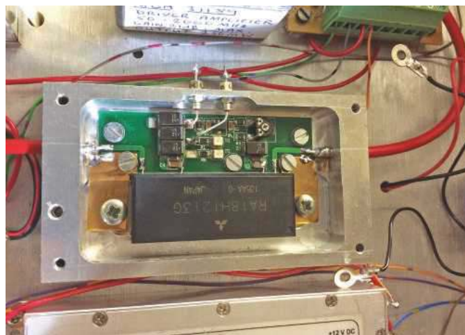
The finished enclosure with lid removed showing final radio frequency and power connections and the use of some brass shim to earth bond the module fixing screws to the co-axial cable and circuit board.
