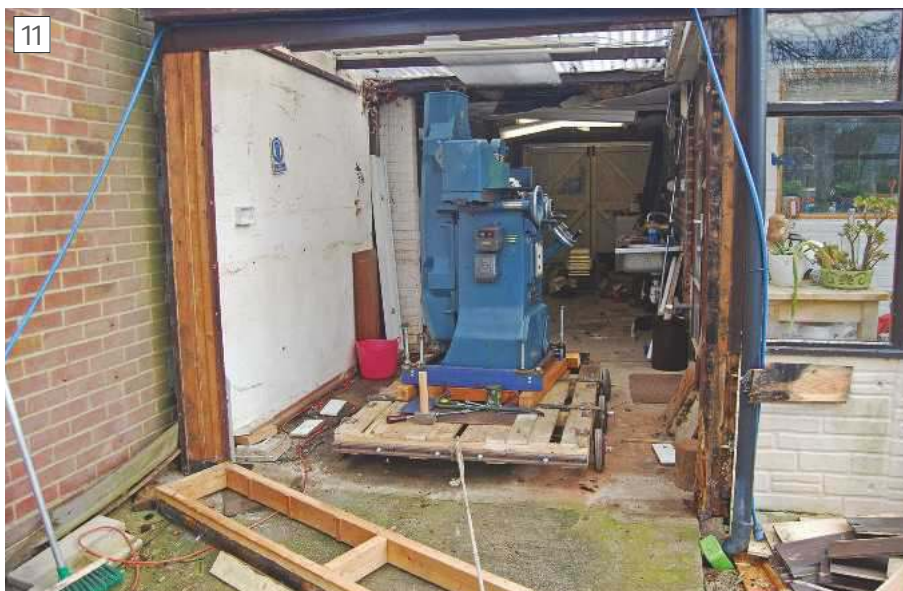
Rear of Garage Removed
