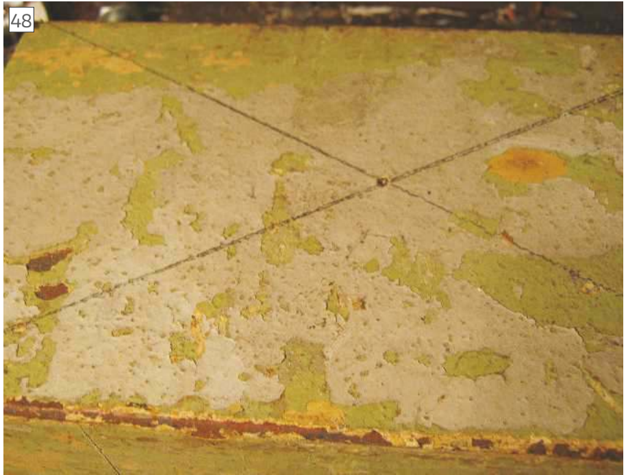
Ready to start drilling
