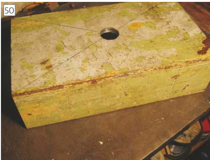
Marking out on large channel
