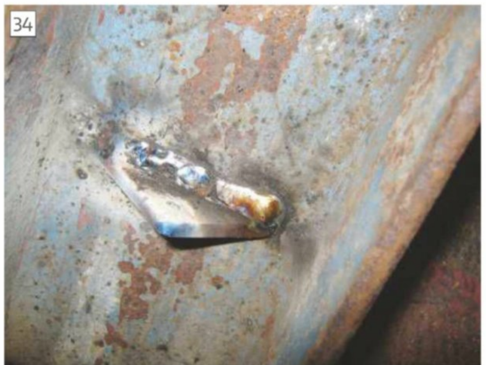
Spring supports welded in position
