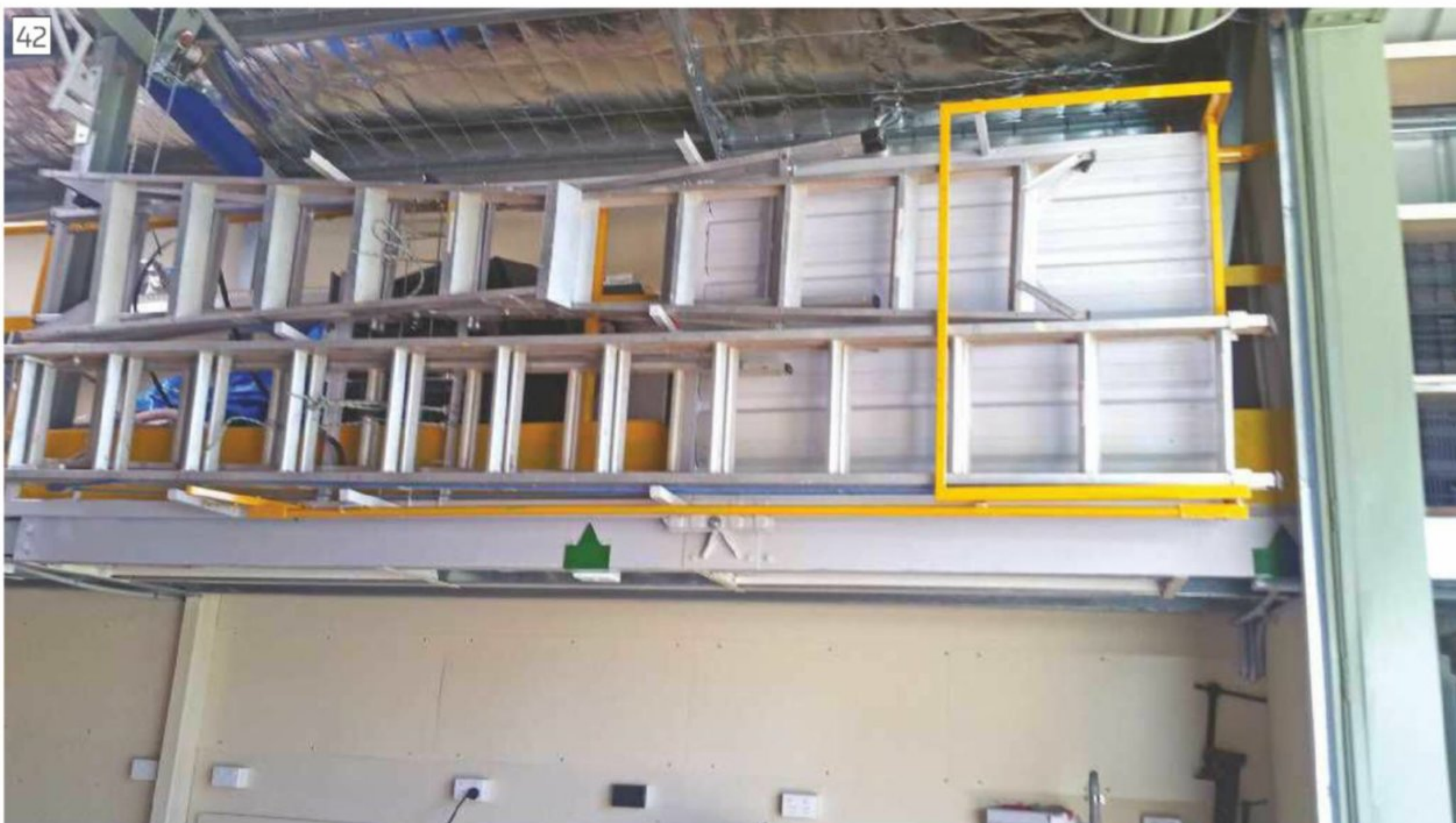
Ladders pivoted up out of the way
