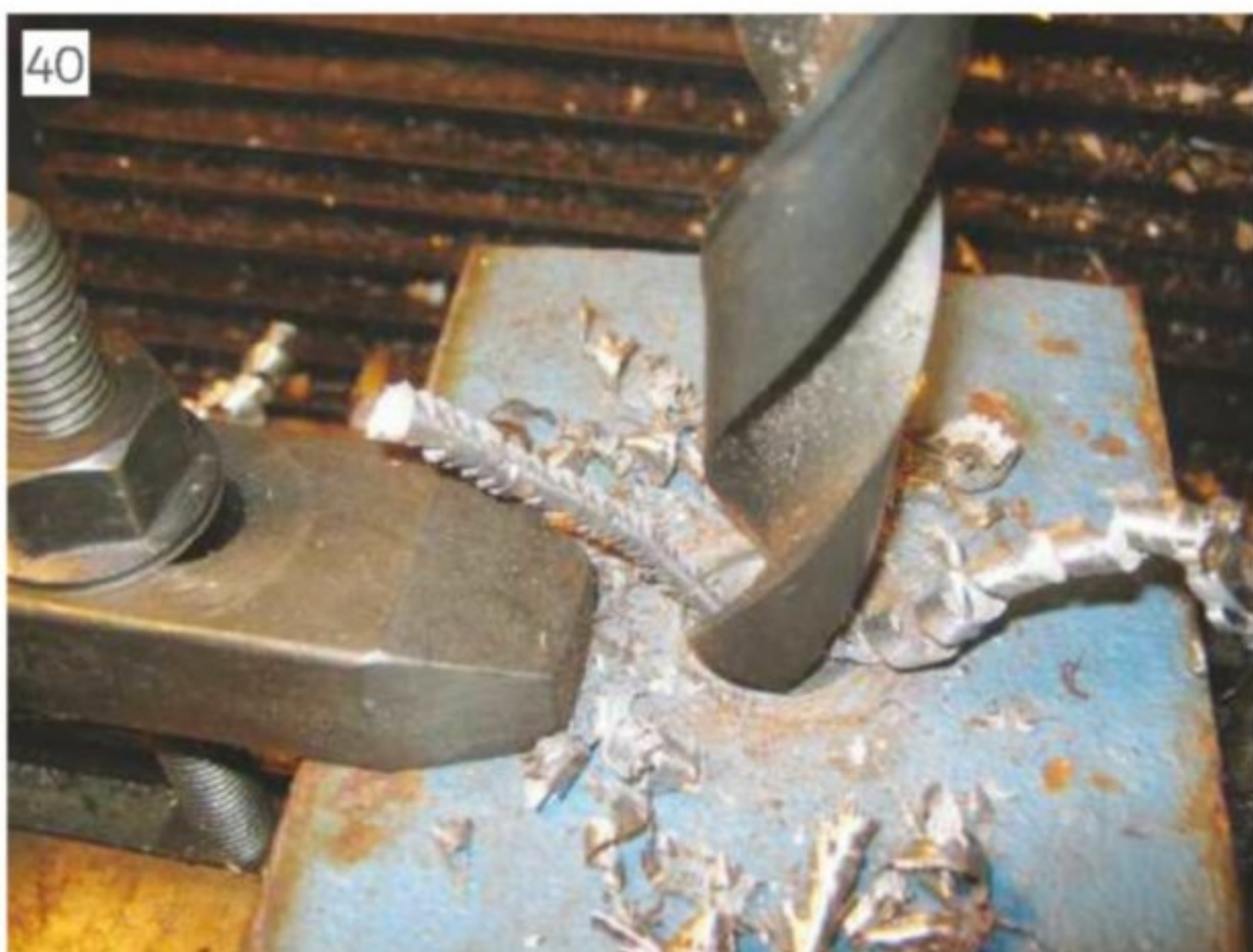
Drilling first 21mm hole base frame
