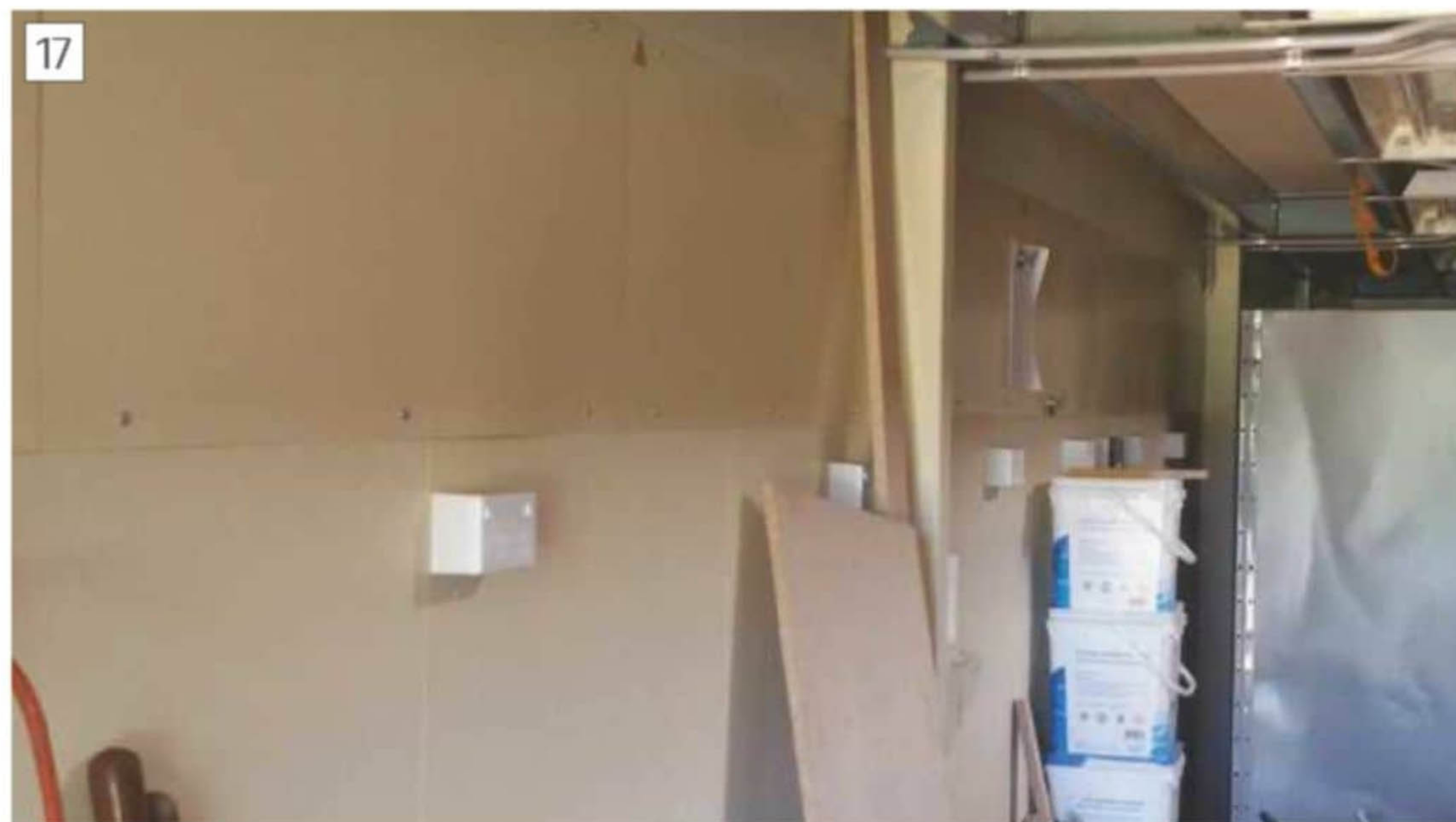
Cover in place
