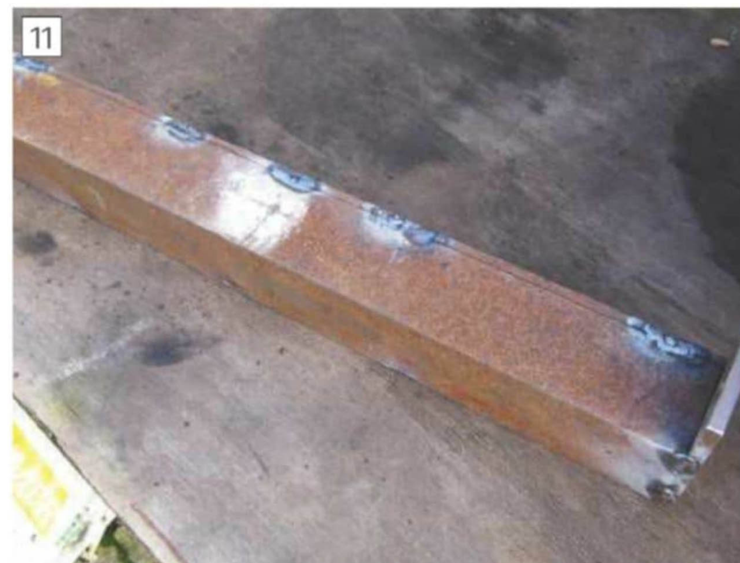
Ram guide tack welded
