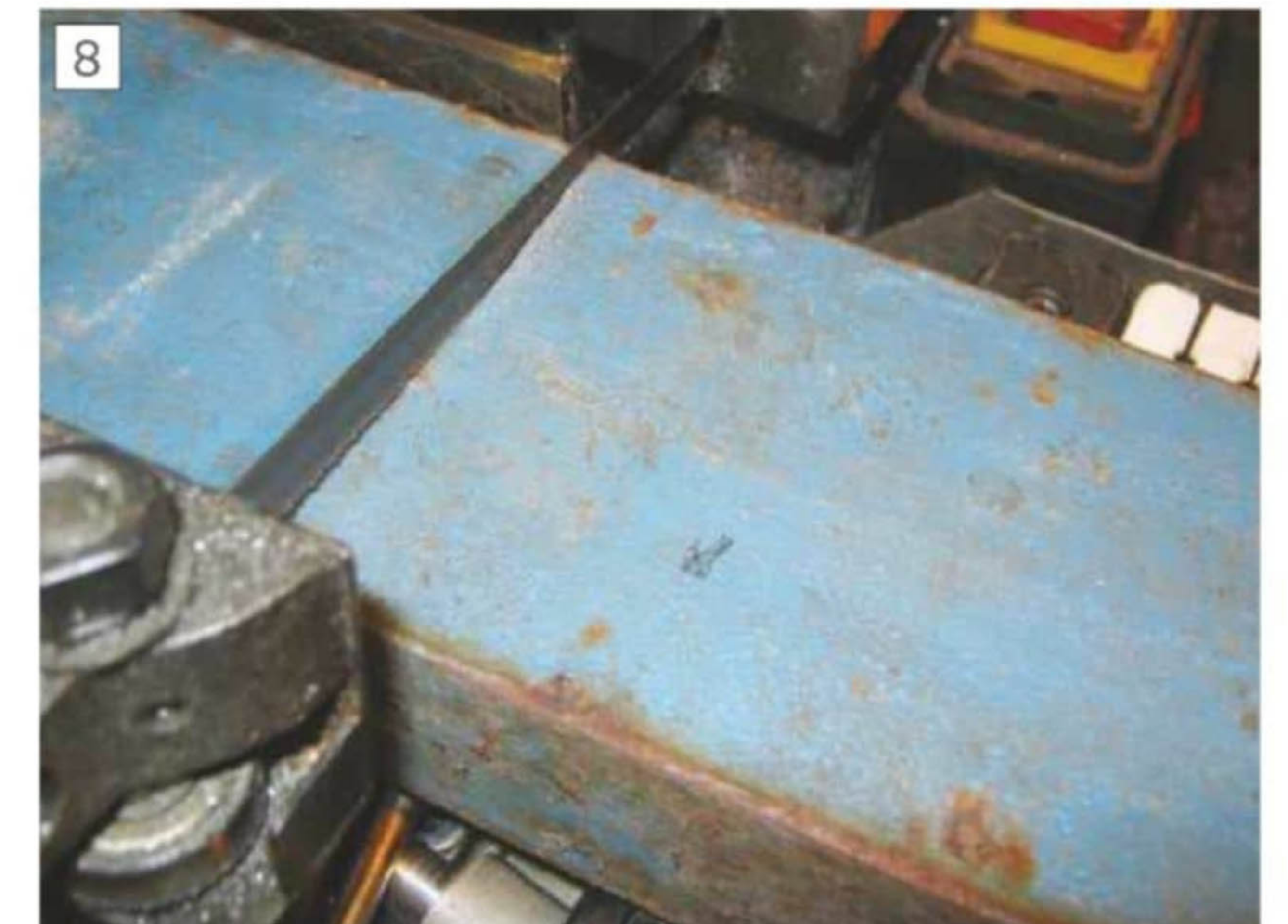
First channel cut
