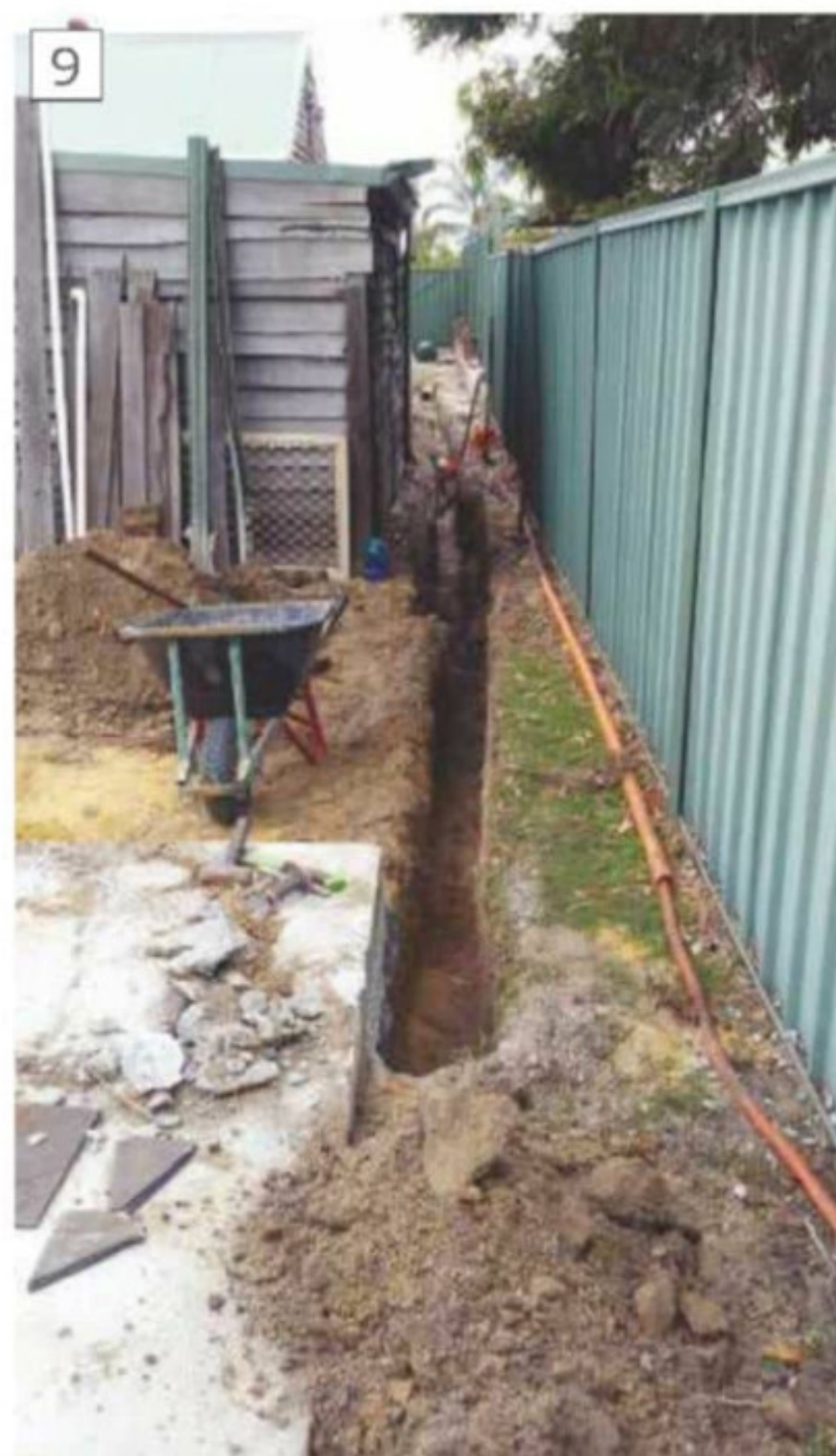
Trench for power supply
