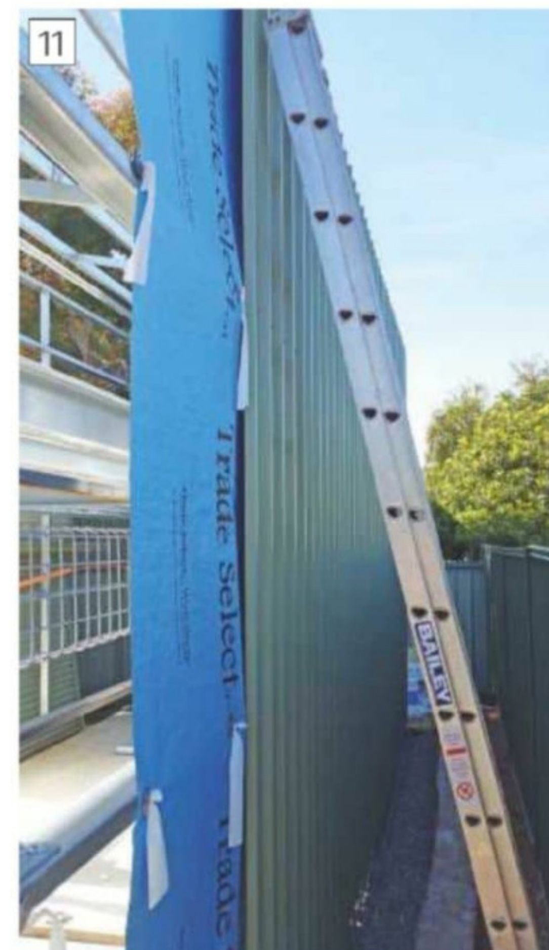
Fixing cladding
