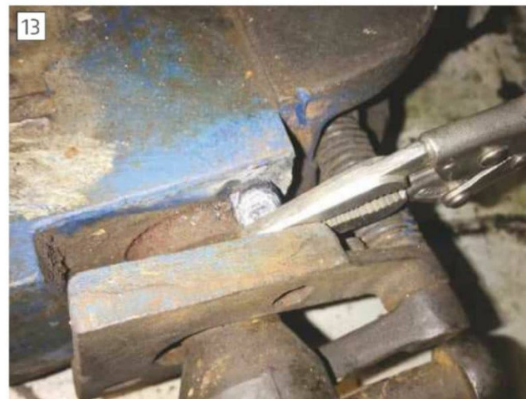
Removing screw with welded on head using grips
