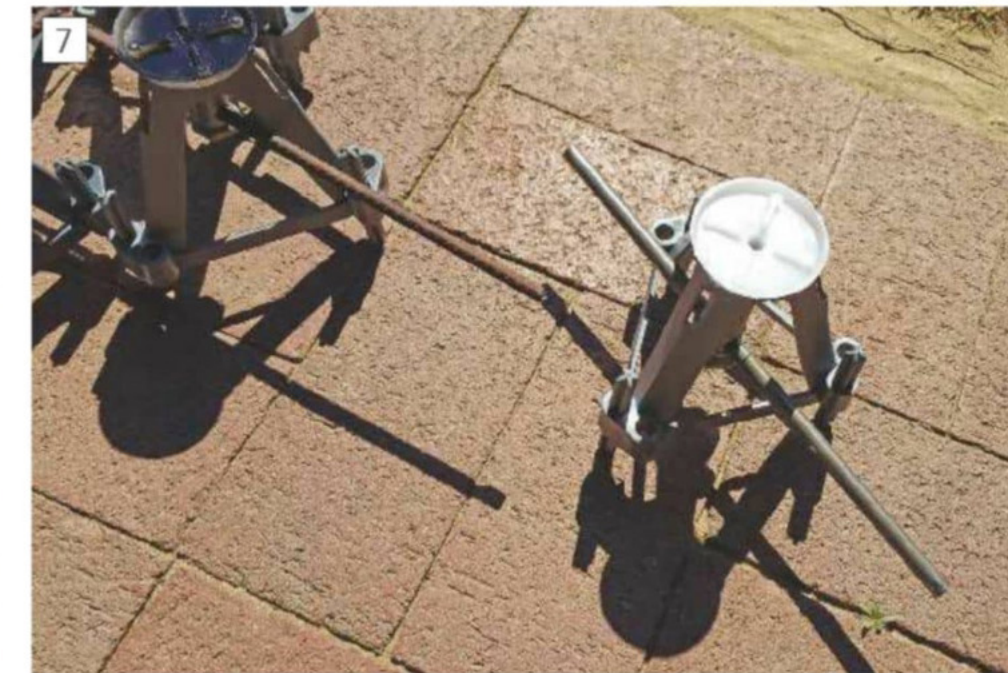
With reinforcing bar and cap
