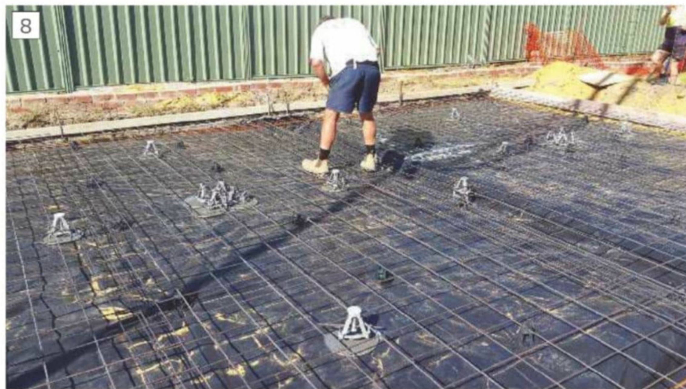
Almost ready to pour.
