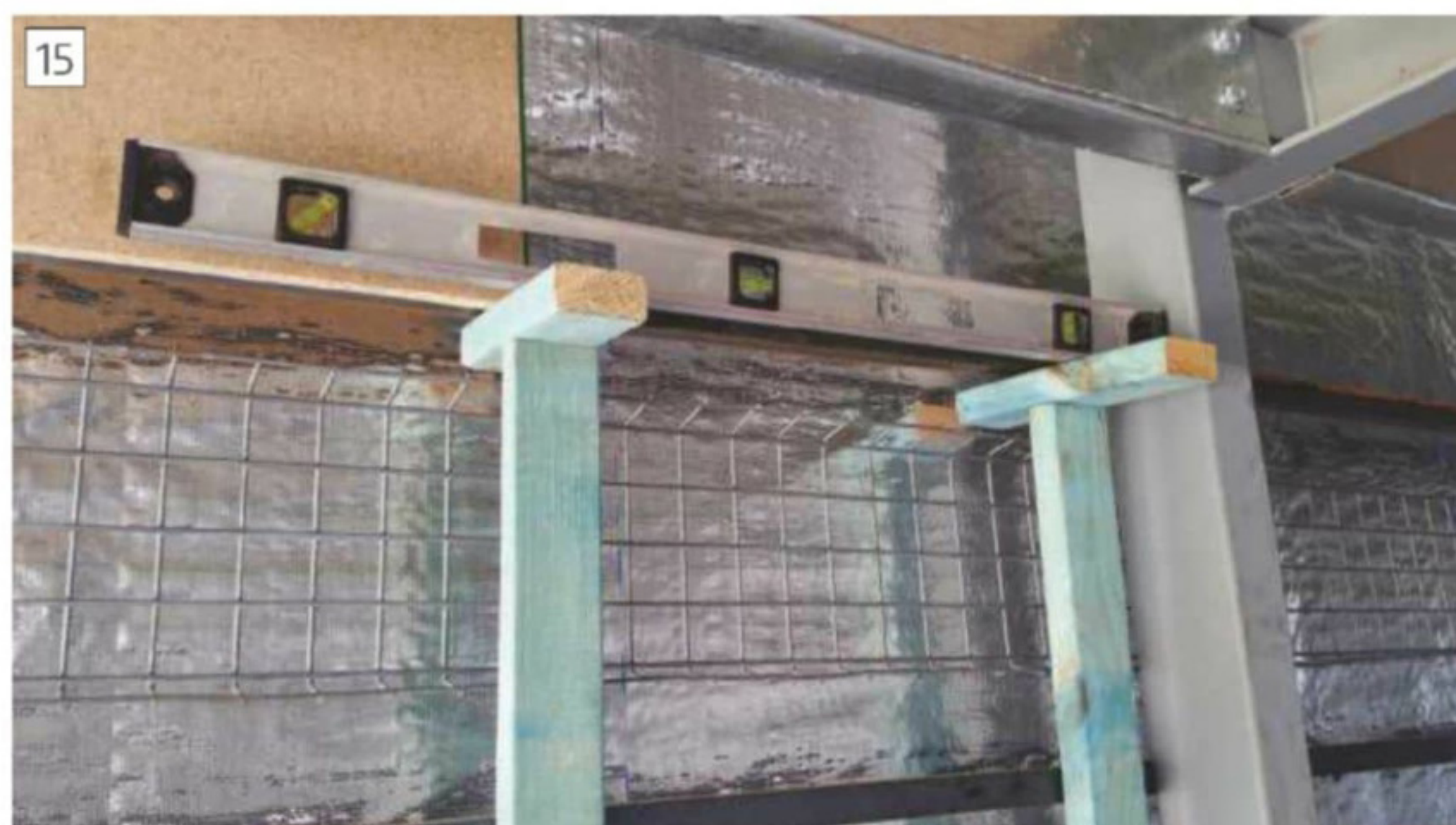
Installing wall lining
