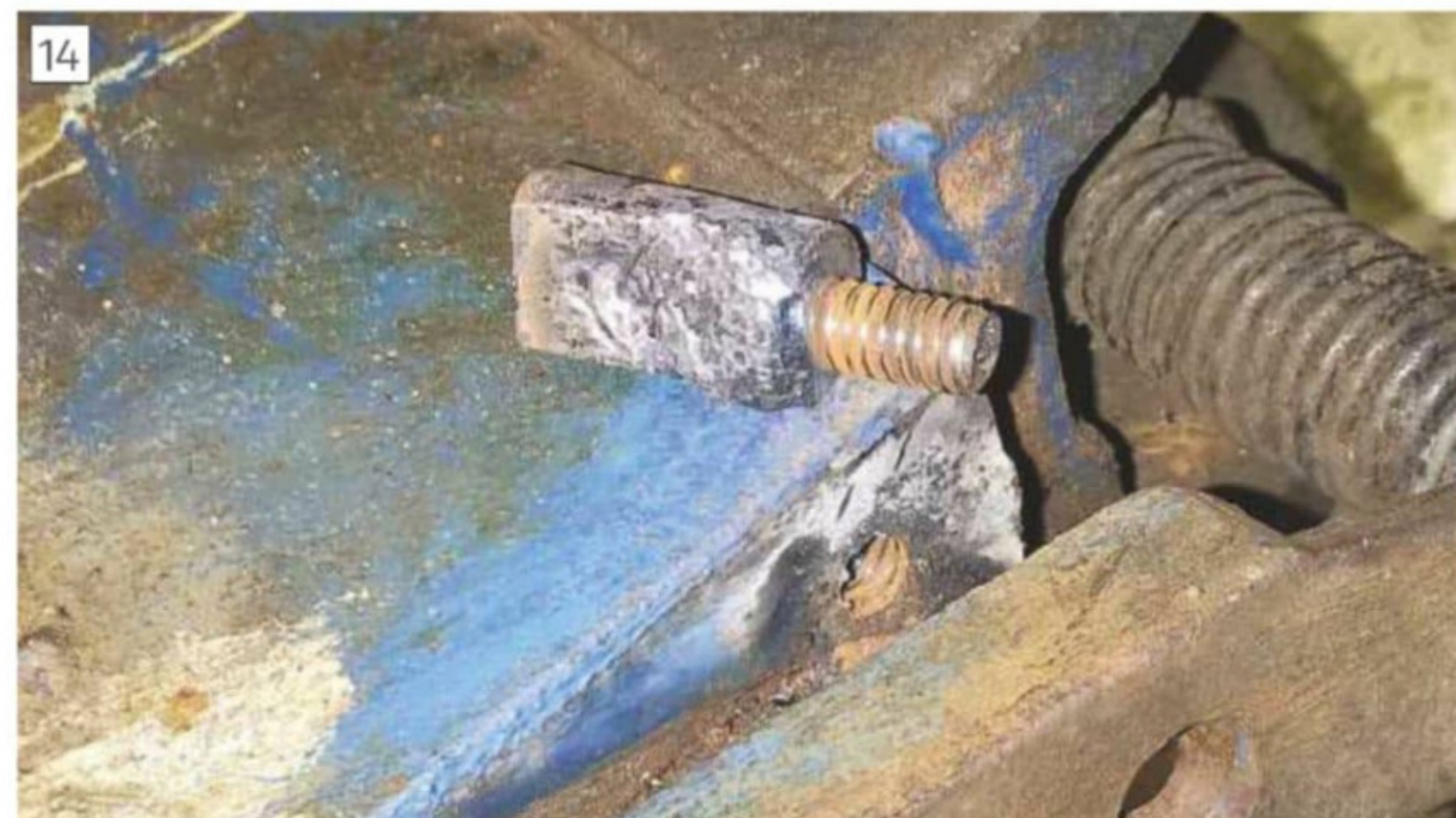
Screw removed and on its way to the scrap bin
