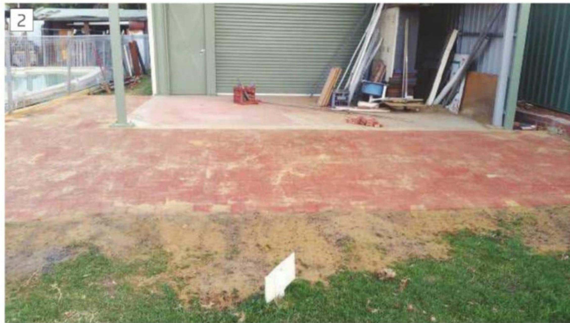
Paved area for hot work
