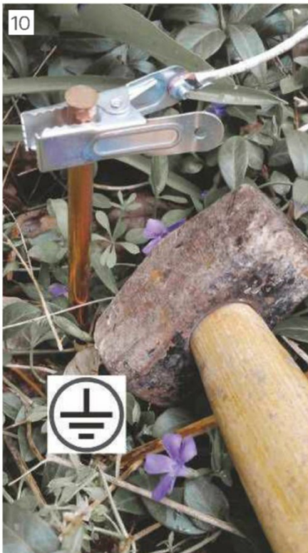
Earth grounding rod and cable connection.
