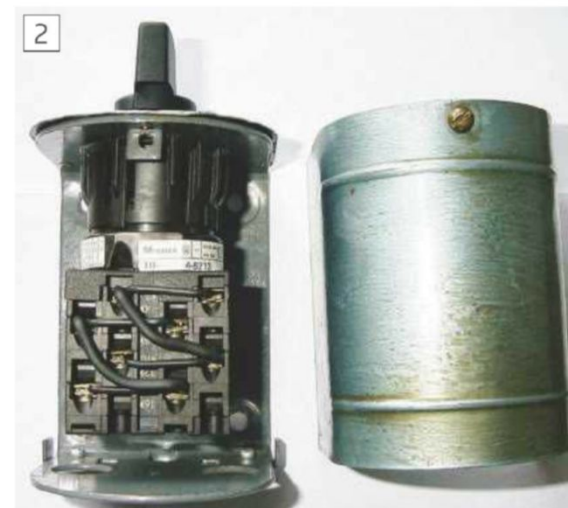
New switch fitted inside old casing
