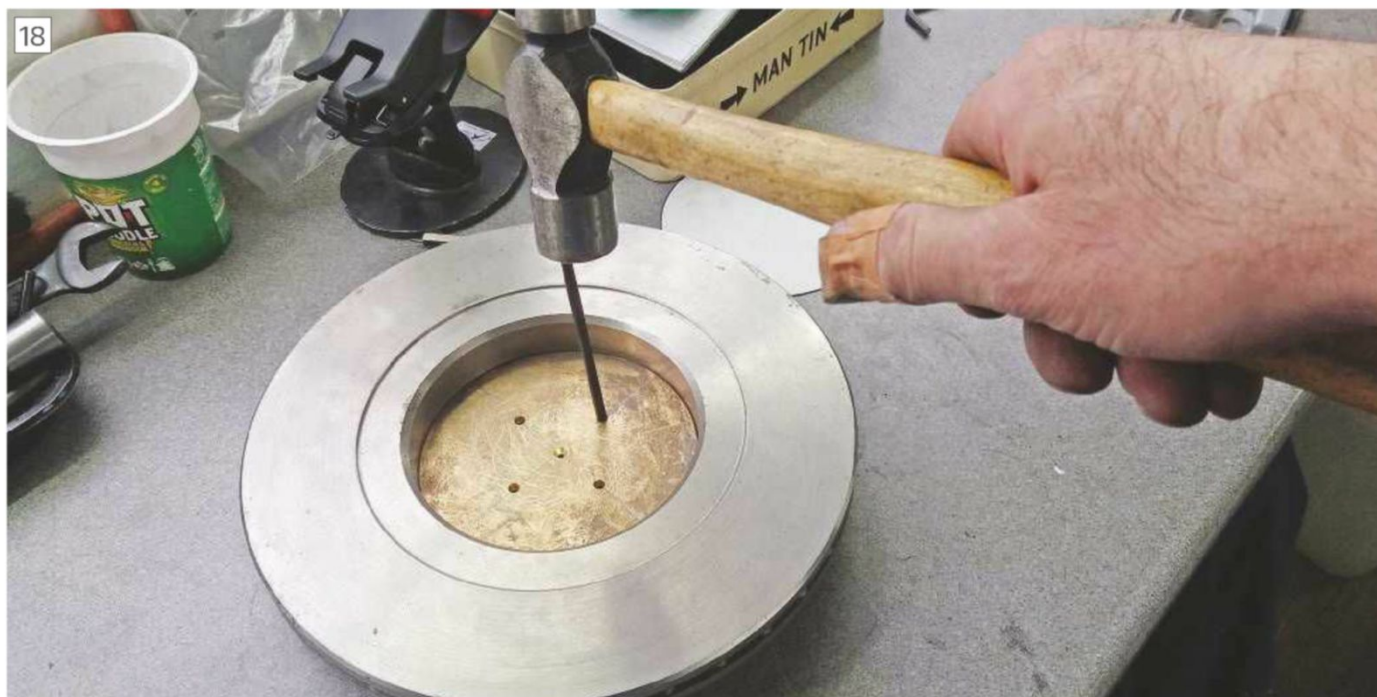
Using a transfer punch to mark the steel plate
