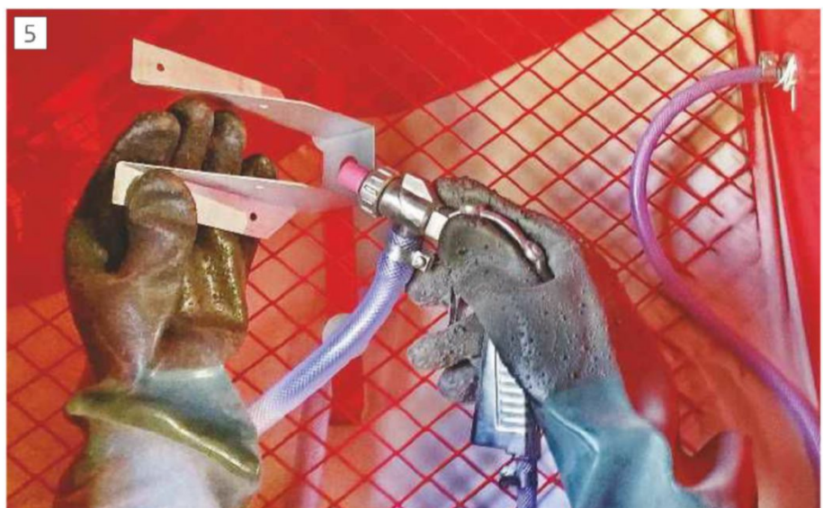
Sand-blasting is the ideal preparation.
