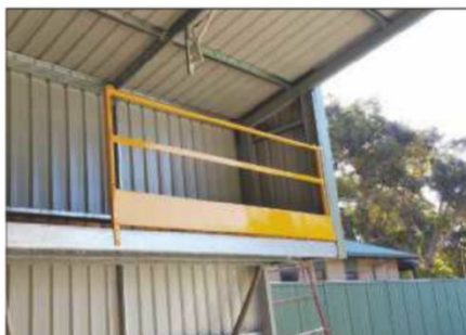
The Story of a Shed - Des Bromilow builds his dream workshop
