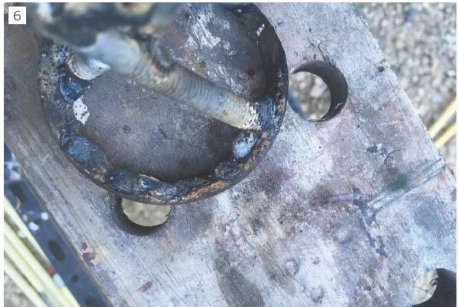
Crude and roughly applied but with maximum current for deep penetration
