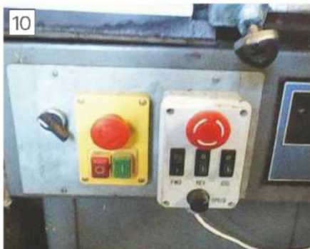
Electrical controls. From the left, suds pump switch, main on/off switch, inverter controls.
