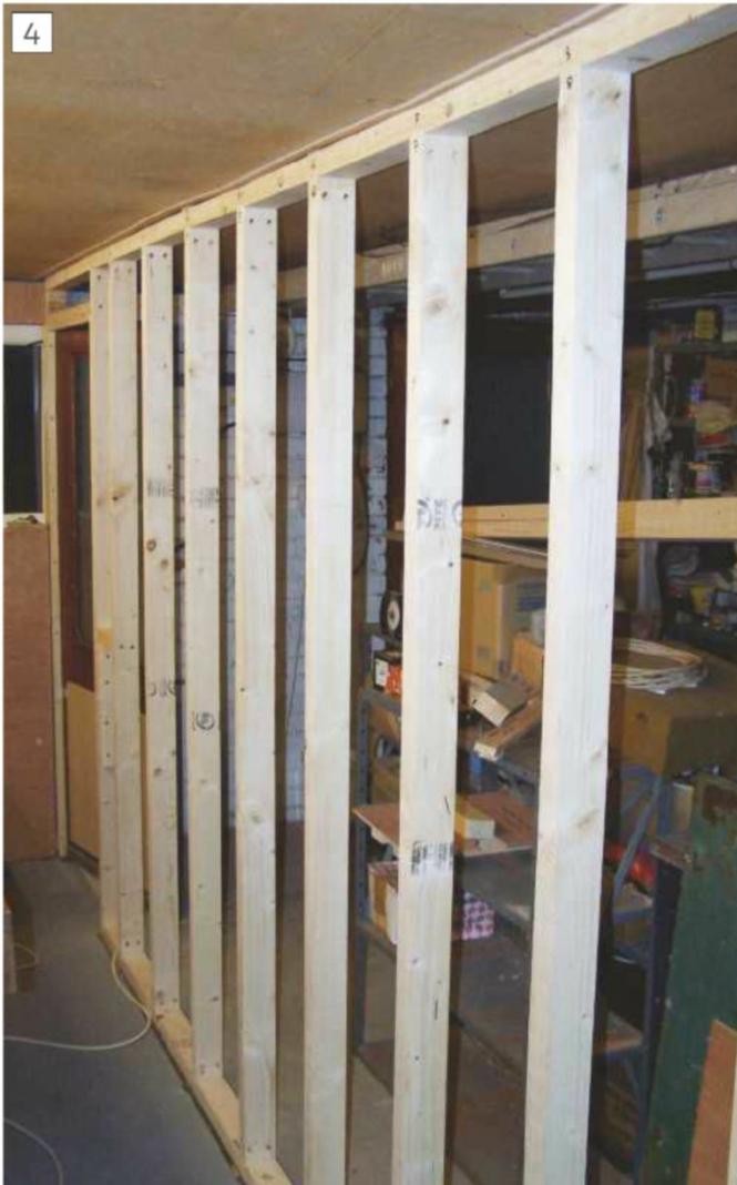
The timber uprights for the wall
