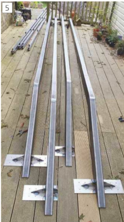
Supports almost ready for the attic
