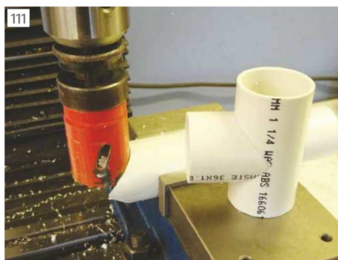
Cope cutting end of pipe with hole saw
