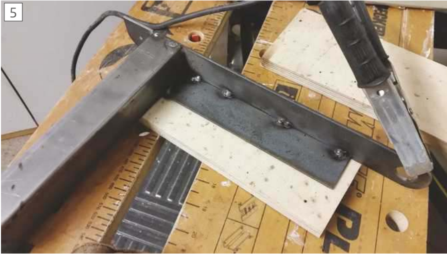
Welding the stiffener using intermittent welds. is complete.
