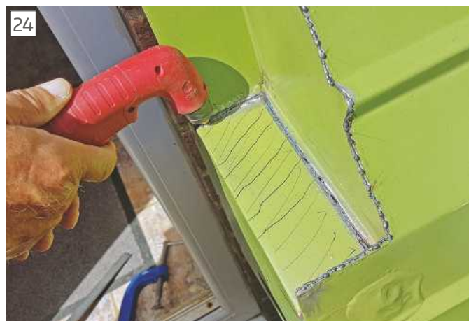
Part way through 2nd cutting operation – first panel removed
