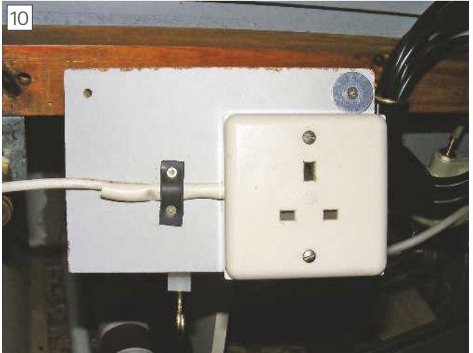
The back of the electric board showing the compressor socket.
