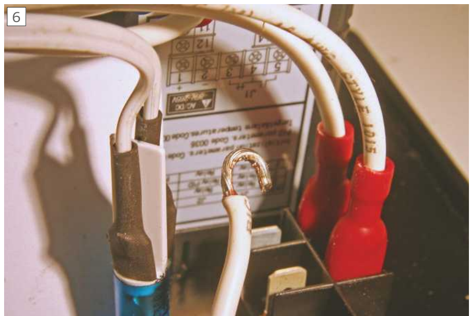
Quality connections on all mains work
