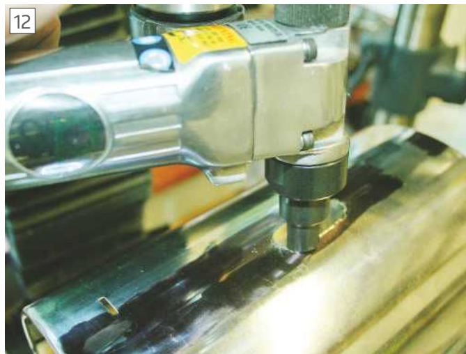
Using a nibbler to cut the top hole.
