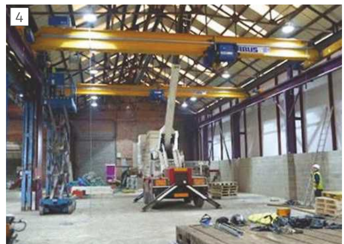
An Ideal place to build a steam loco. Just needs the pit
