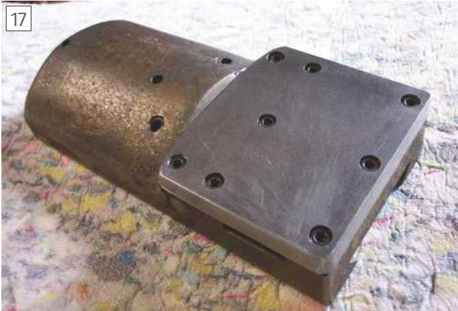
First fit of the new steel plate
