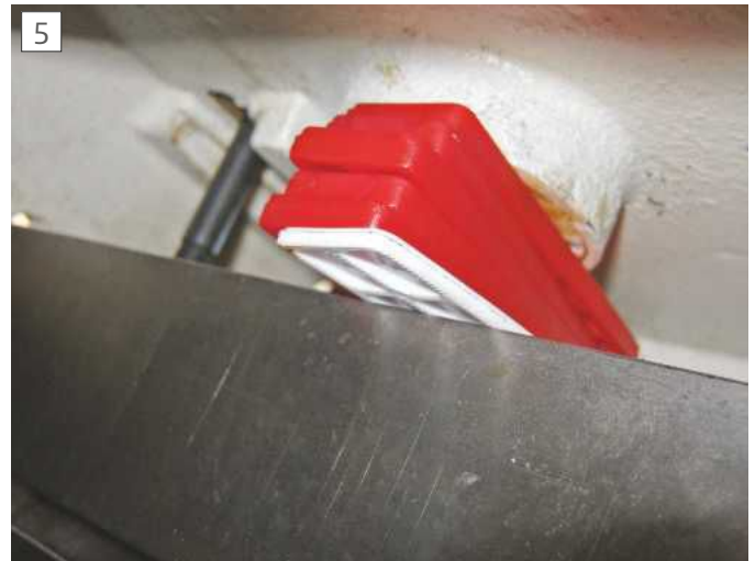
Packers under casting boss
