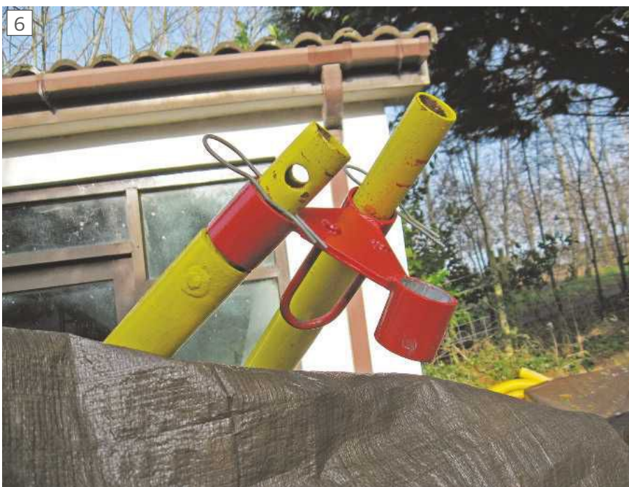
This view clearly shows the eye for the hoist
