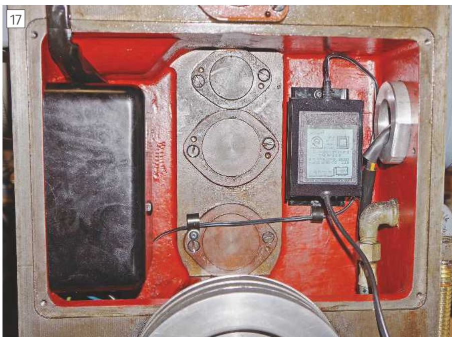
DC supply fitted
