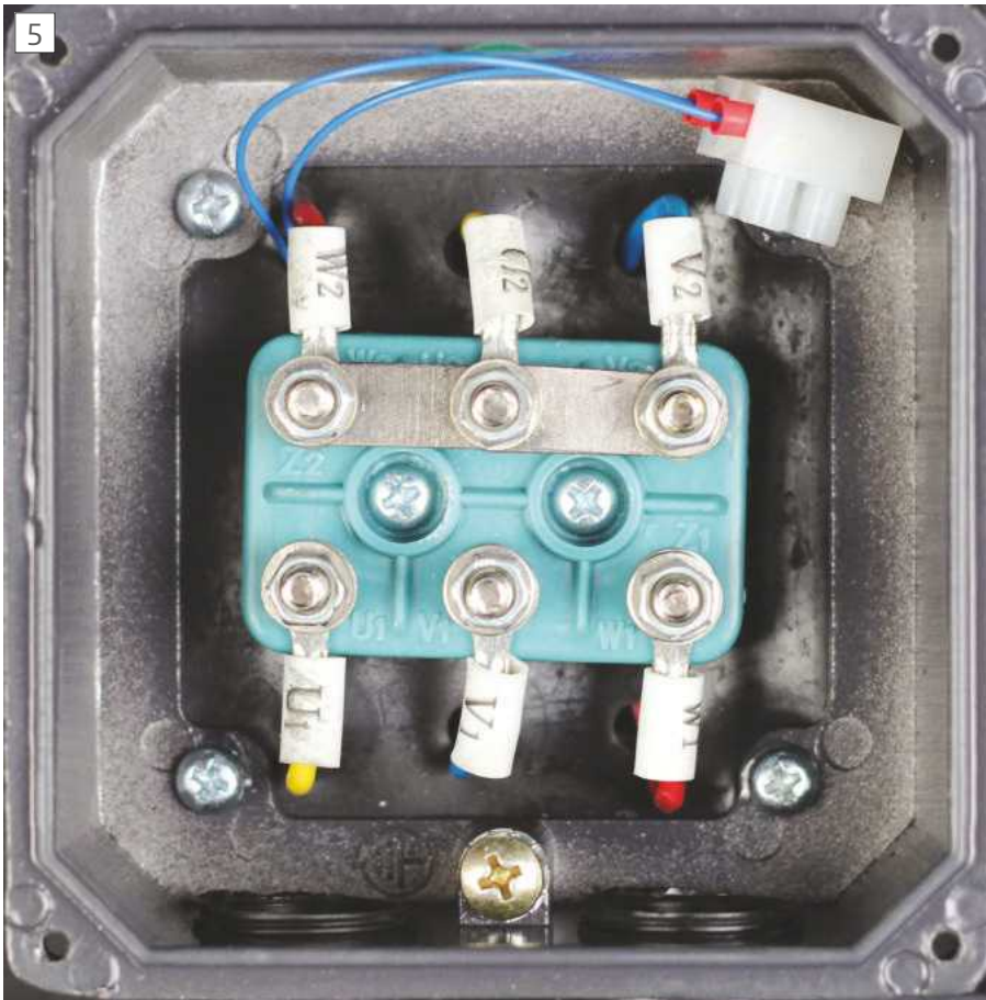
Motor in star configuration.
