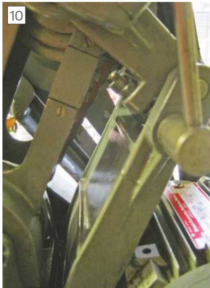
Replaced missing drive guard component
