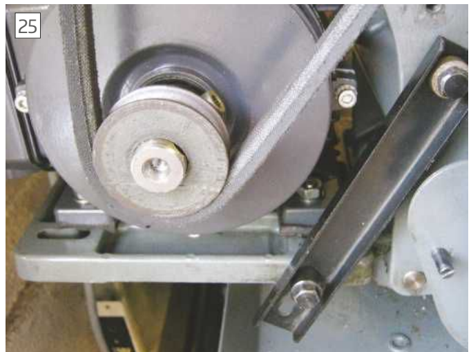
New motor mounted on the inverted platform
