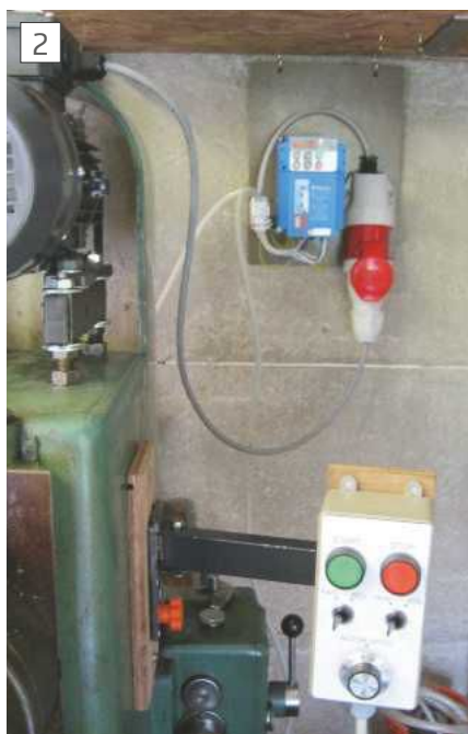
Control Panel mounted for use on the mill
