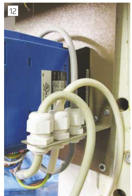
Control box cable support glands
