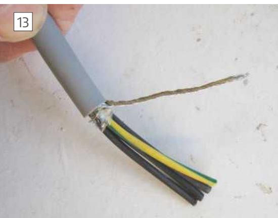
13 Screen braid prepared for sleeving and connection to earth
