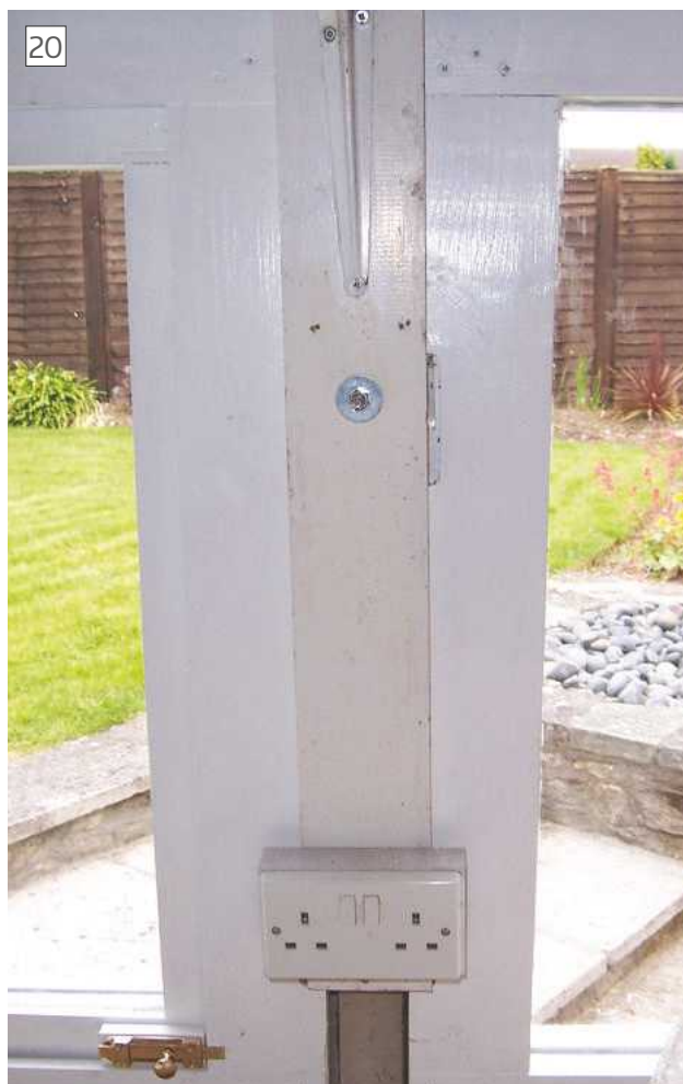
Use of structural bolts to attach wooden shelf supports
