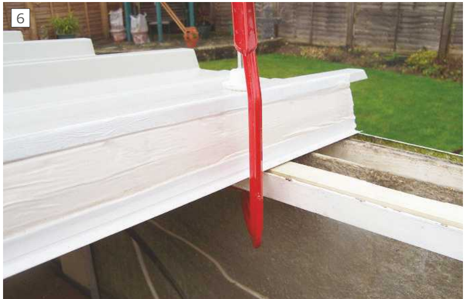
Roofing sheet clamped prior to bolting.
