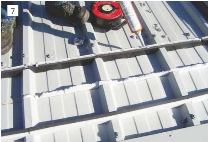
Gap in ridge filled with polystyrene. Applying the gunned mastic.
