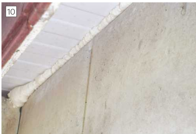
Use of builders' foam to seal between roof sheets and walls
