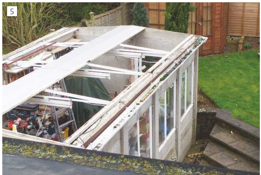
Internal ridge sheet sitting on the wooden battens which in turn are sitting on the 1° angle
