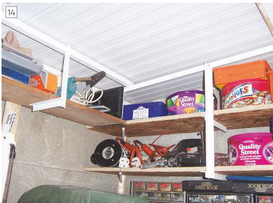
Finished area of new shelves showing additional angle supports
