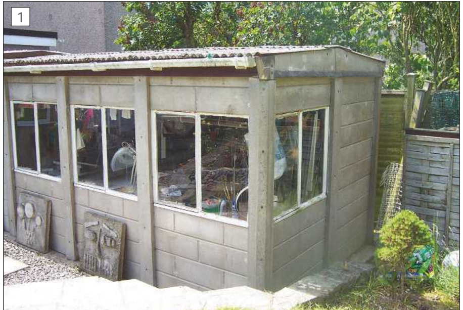
General view of workshop before work commenced
