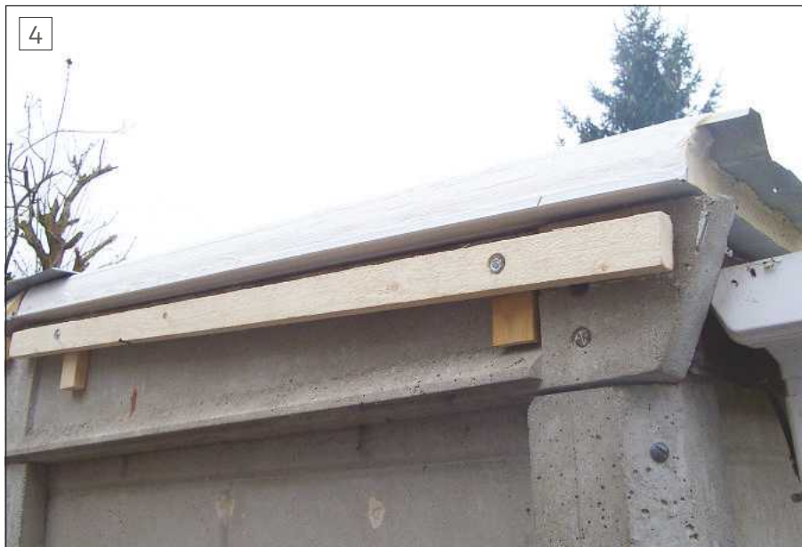
Roof sheet cut back for gutter drip and arrangement to support end caps/barge boards
