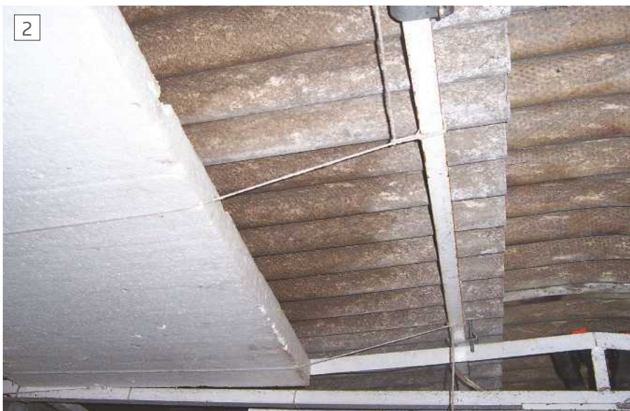
Trial insulation with polystyrene
