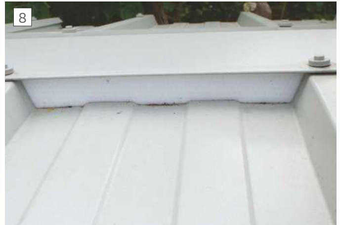
Ridge filler work completed
