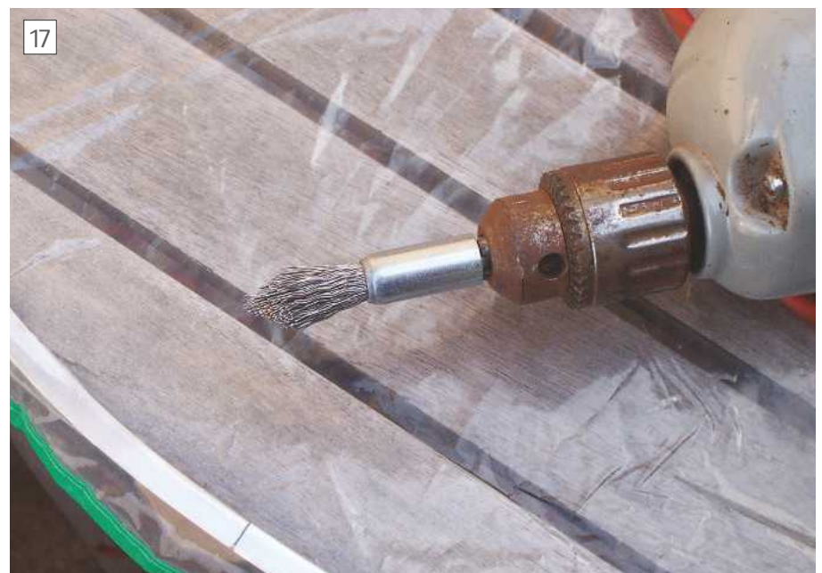
Pencil wire brush used to clean rusty re-bar
