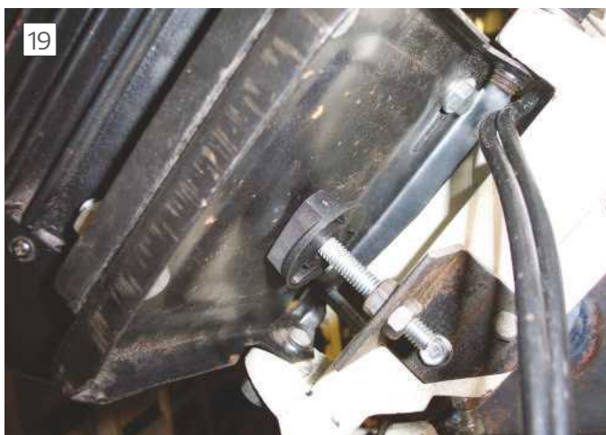
New support screw below motor platform
