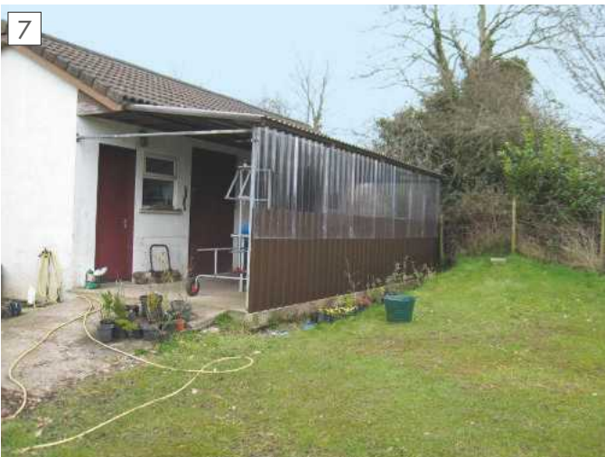
The sheeting almost complete.
