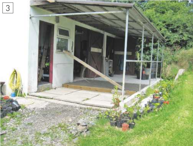
Laying the concrete floor.
