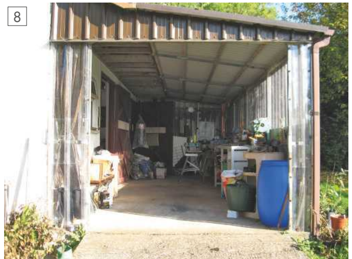
The gap to be filled by the doors.
