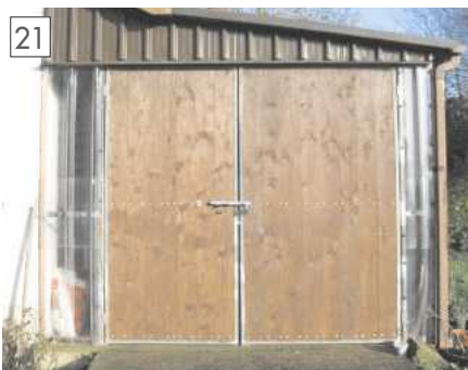
Both doors installed.
