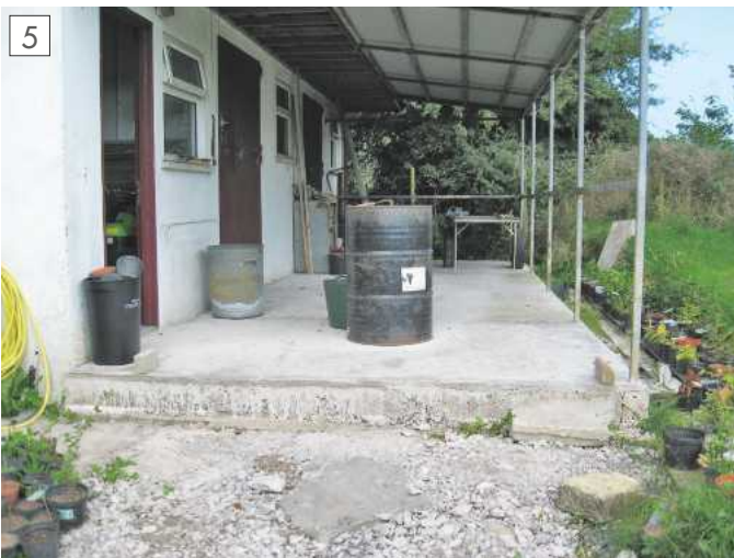
Concrete floor complete.
