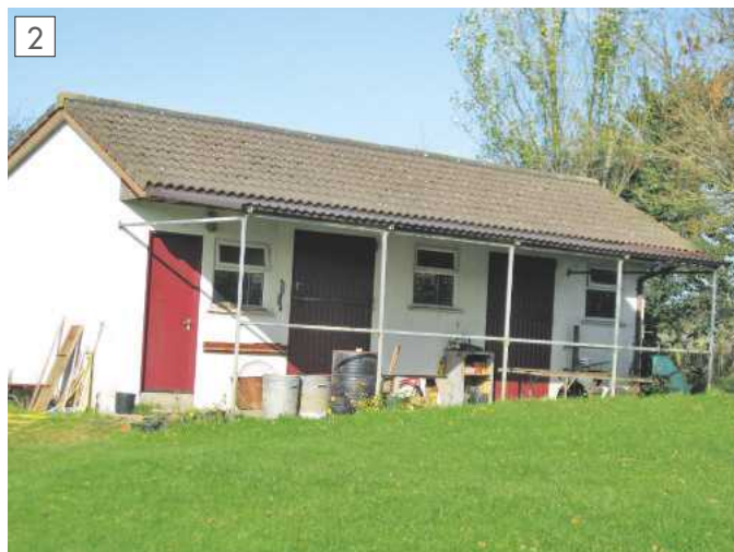
The roof 'tin' went on first!
