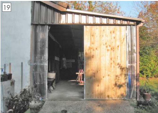
First door installed.
