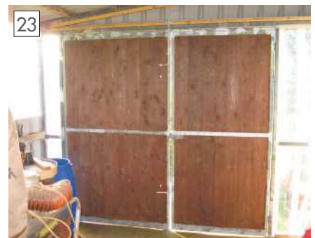
Internal view of the new extension.
