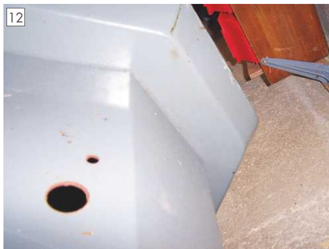
Underside of tray showing area available to fit new drain.
