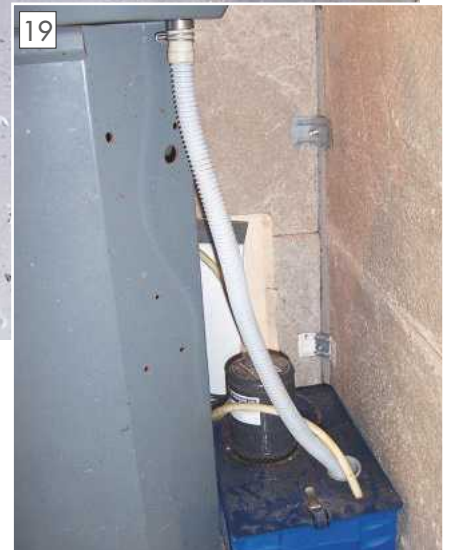
The completed drain system.
