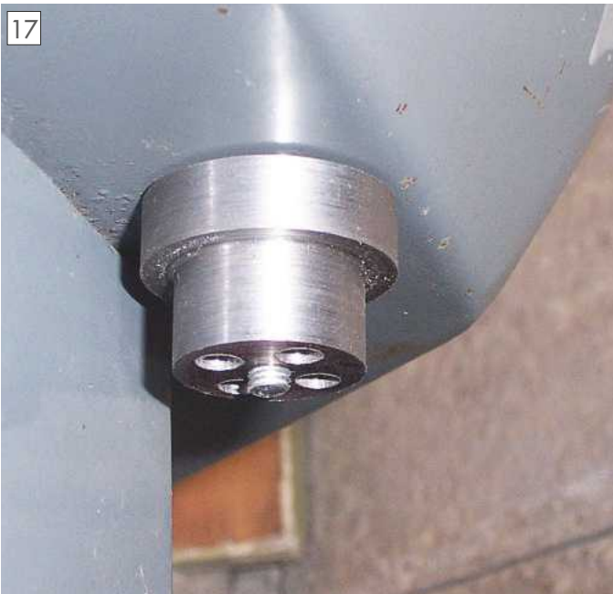
Underside view of tray with new drain branch fitted.
