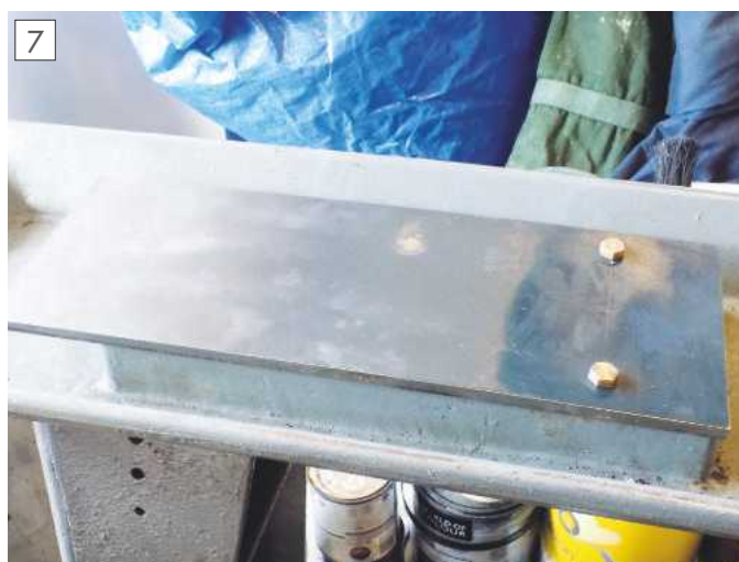
Plate bolted in position.
