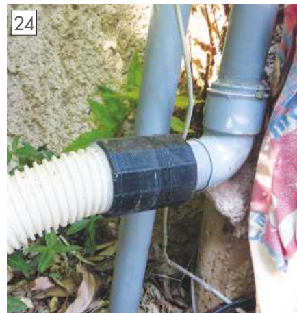
Printed version in place showing the bead of silicon ensuring a seal.
