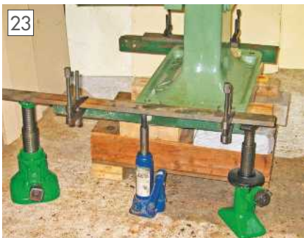
Jacking up the mill to enable trolley to slid underneath.
