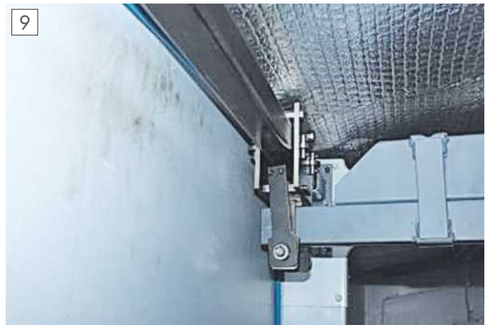
A front view of the UJ.
