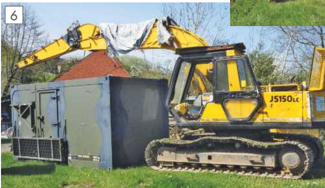
6 Ready for rigging the load.
