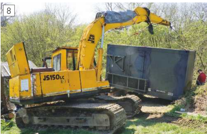
8 Positioning on foundations.
