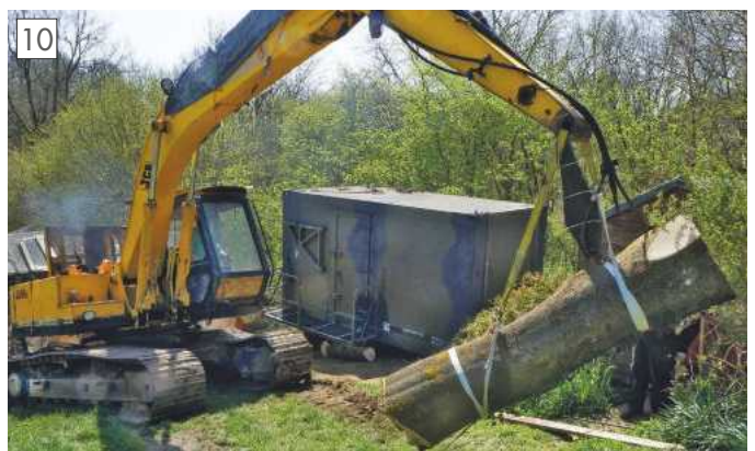
10 Removing the Ash Tree.
