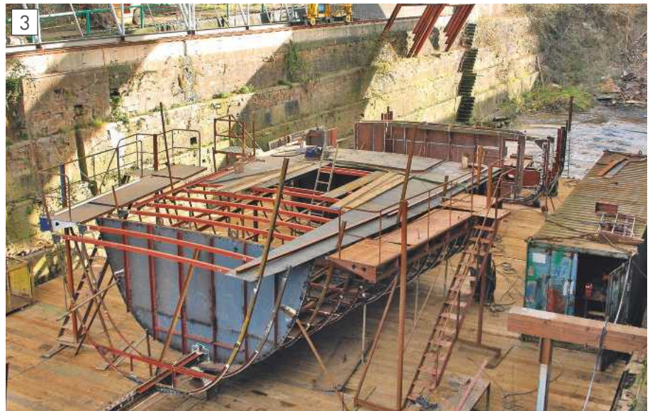
An early stage in the hull build (D. Abels).
