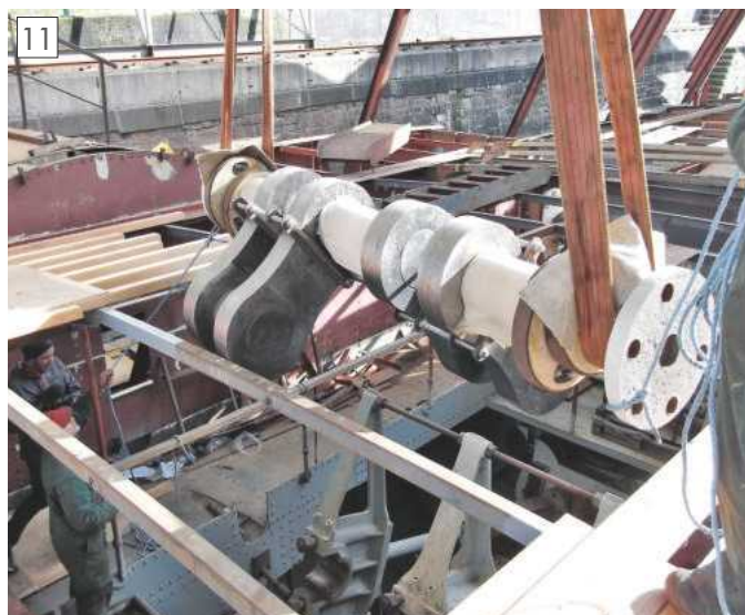
The crankshaft is lowered into position (MQPS).
