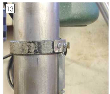
The repaired ring.
