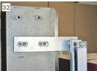
32 The upper Z axis bracket with scale and cover backing temporarily secured in place.
