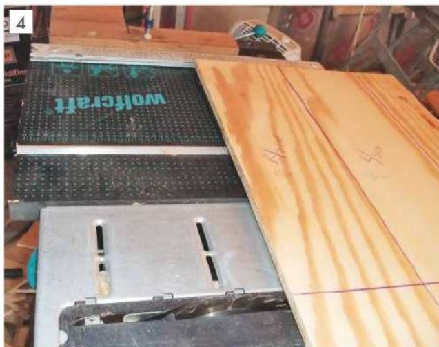
4 Improvised fence for cutting panels to size, safety guards removed for photos.
