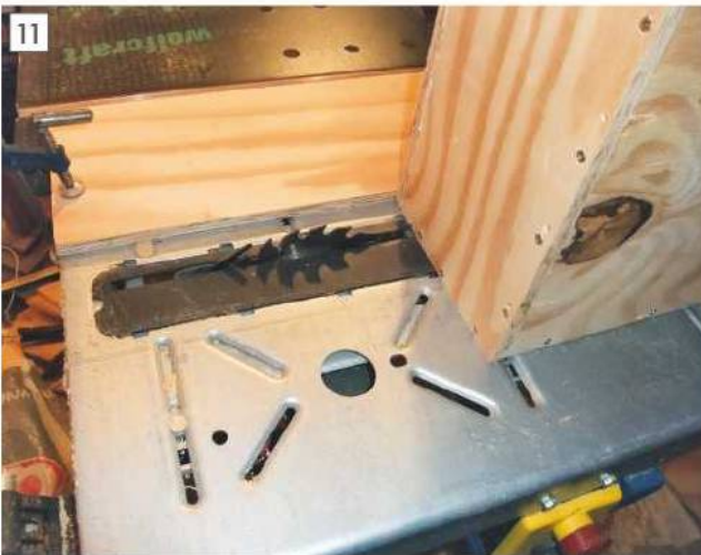
About to make the first cut to remove the front.
