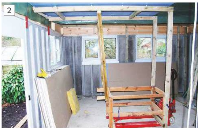
Plaster board raised ready to fix.
