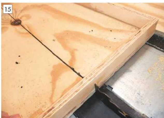
Lid face down, cutting half way through.
