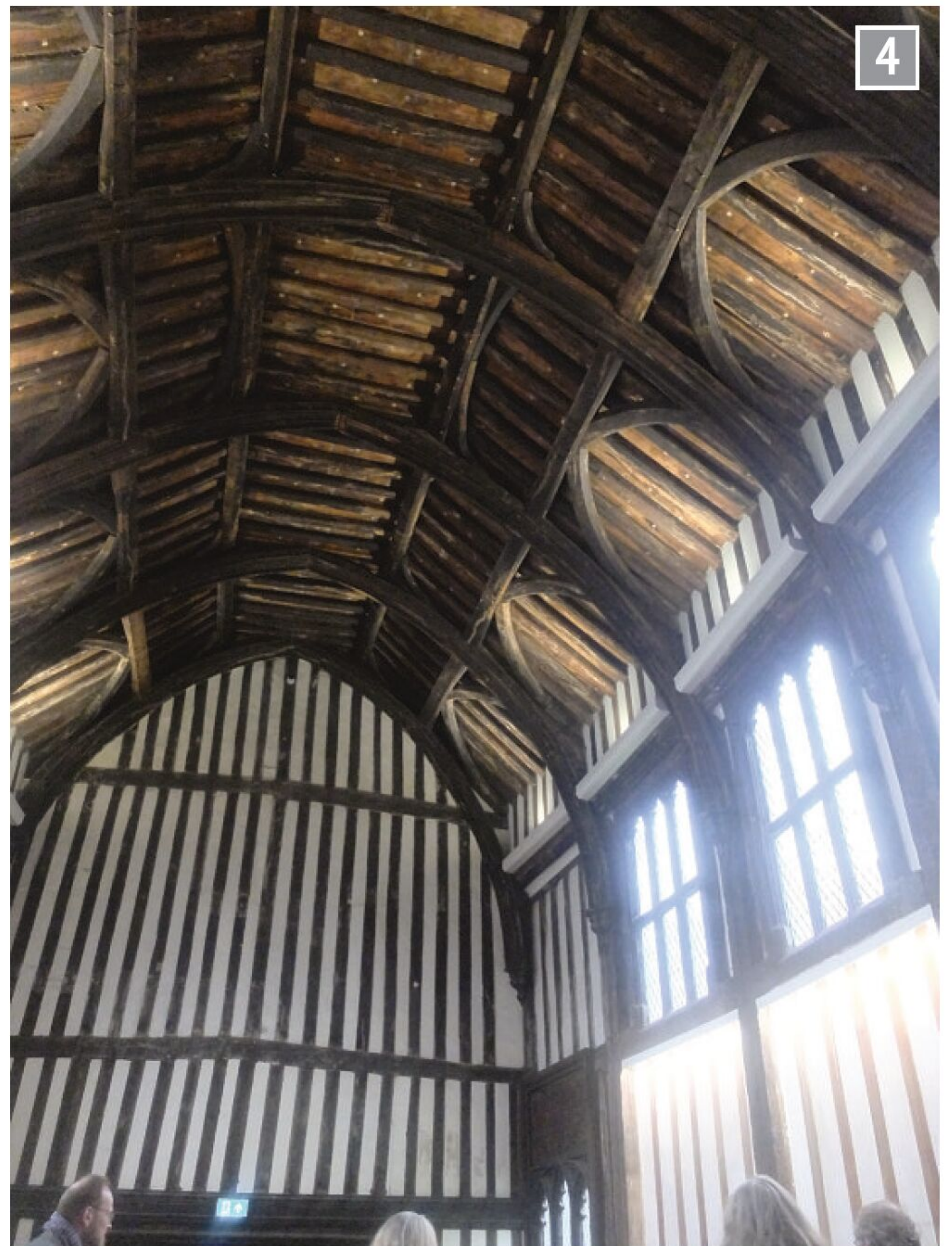
Gainsbrough Old Hall, roof.
