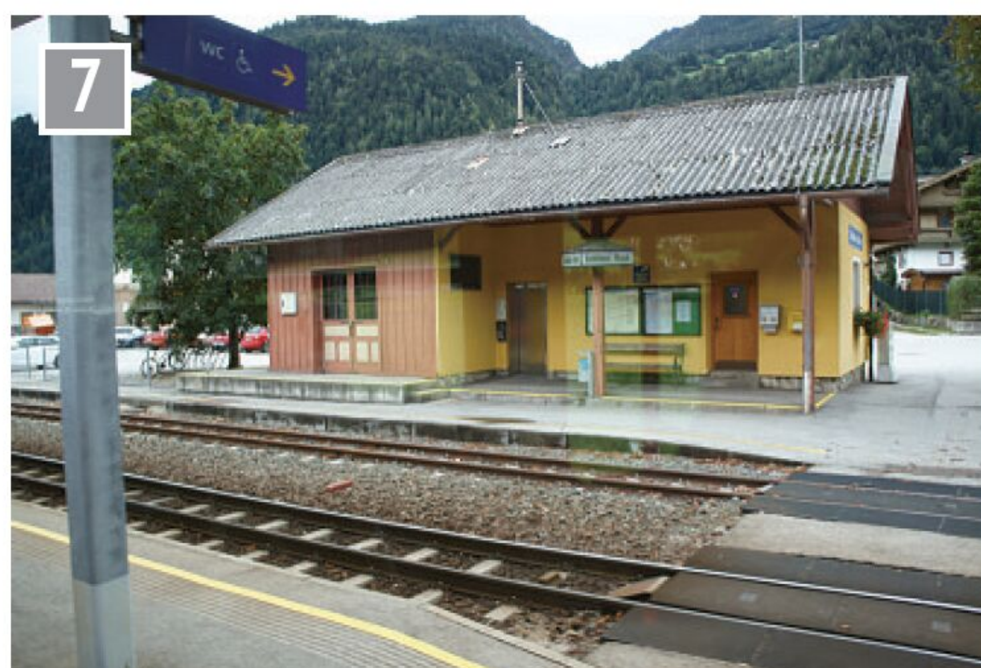
Stations like Schlitters Bruck are well built and maintained.
