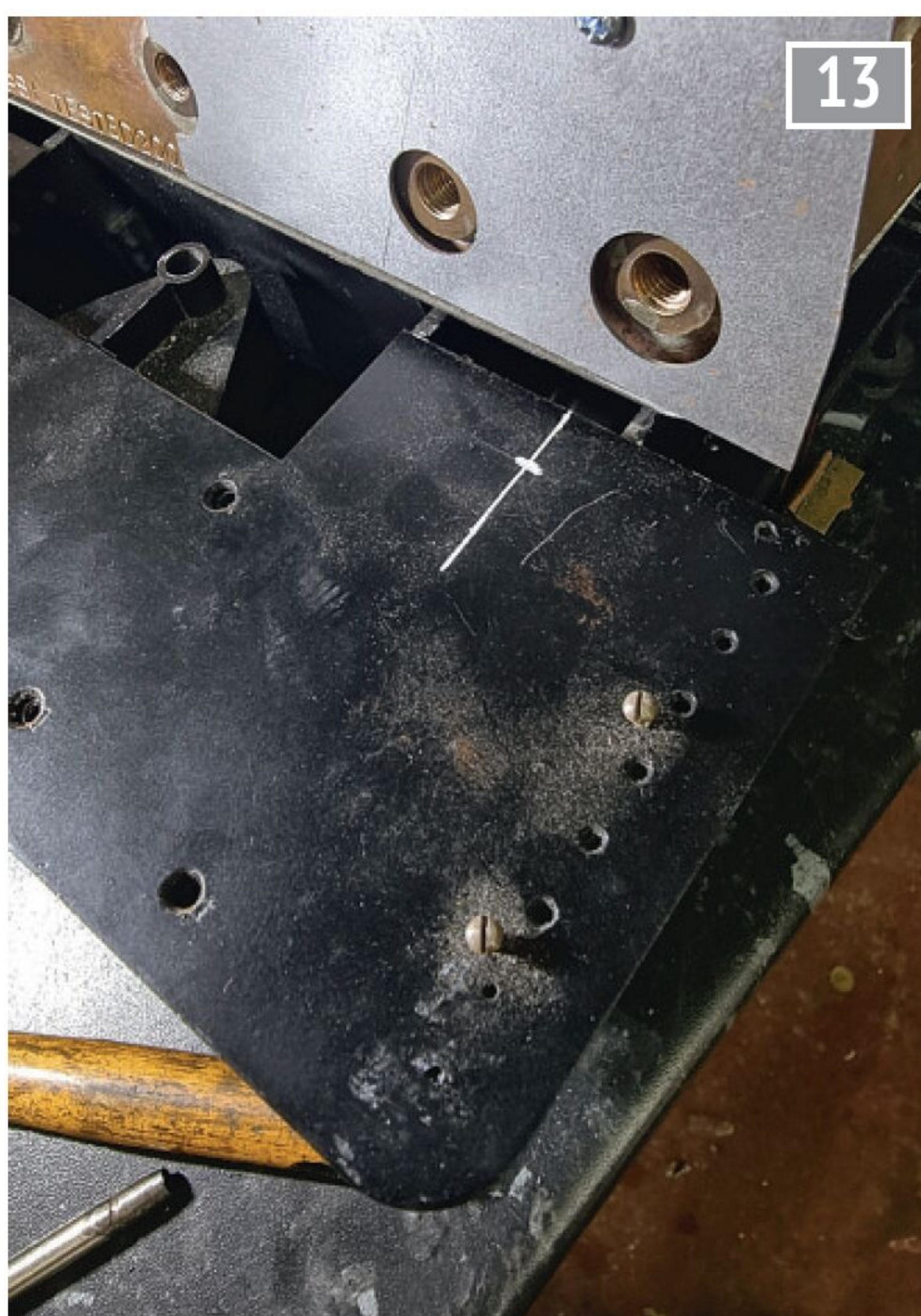
Initial mark for the cab floor cutout.
