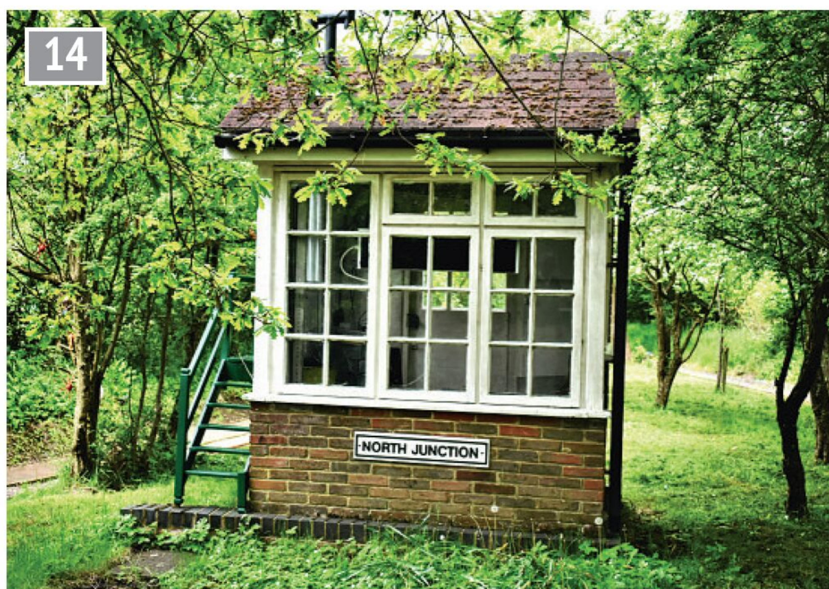
North Junction Signal Box.
