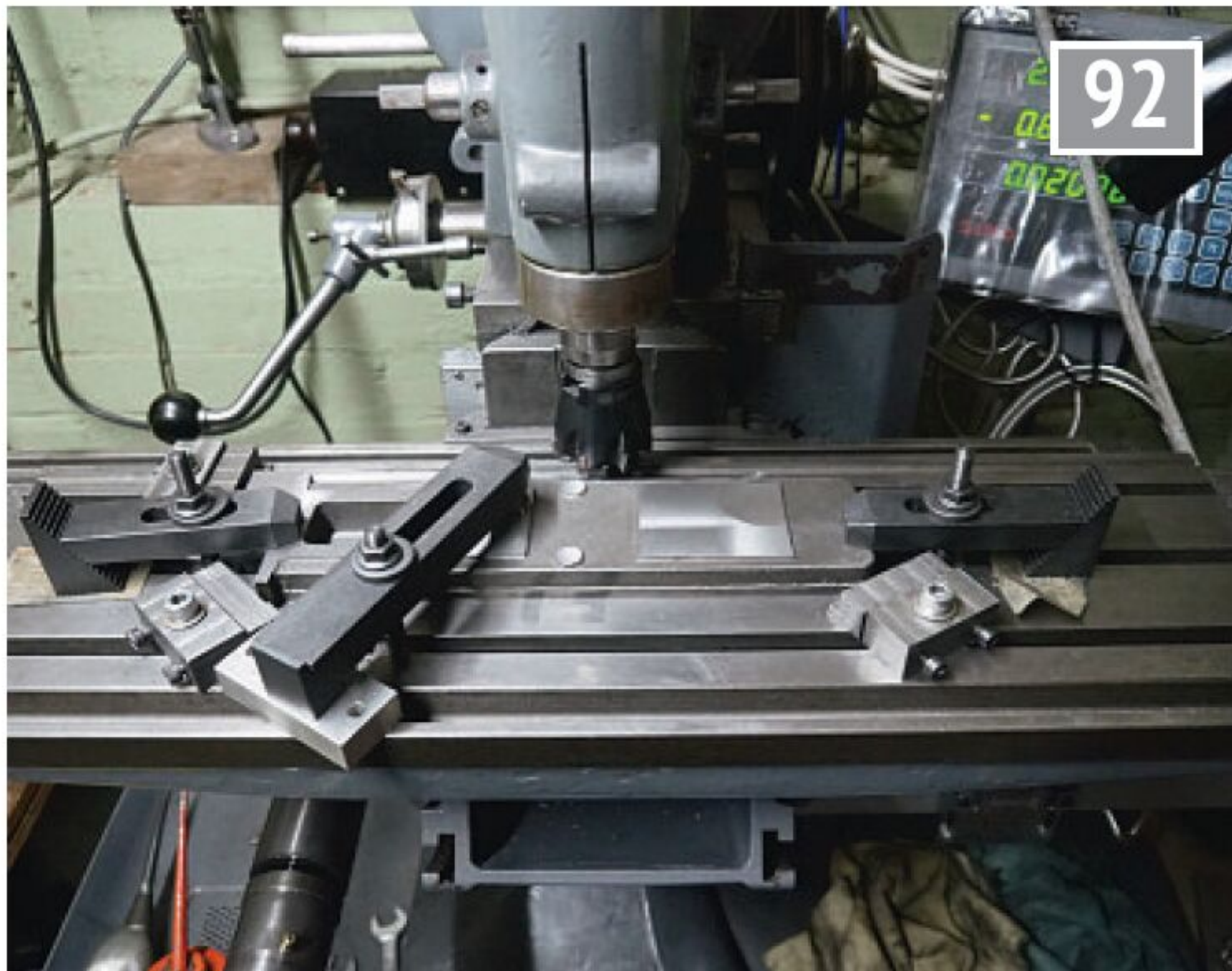
92 With the soleplate turned over the cylinder mounting pads are finished to height.
