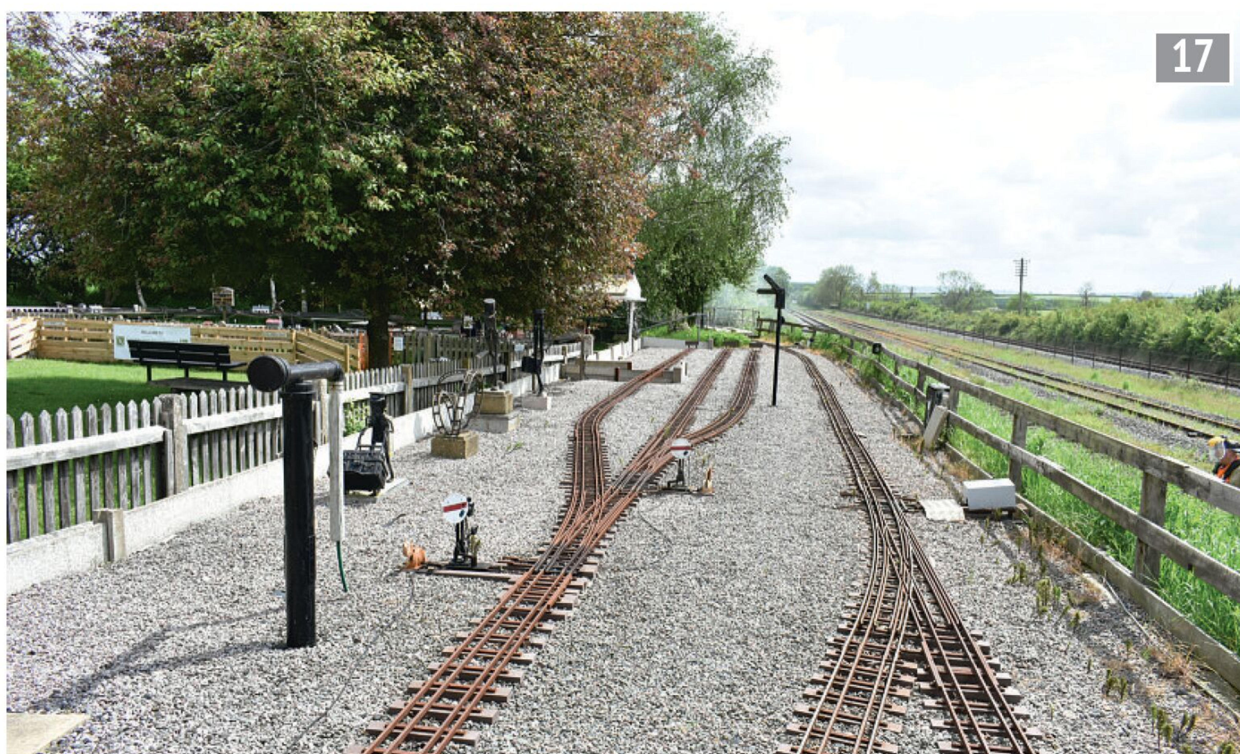
The arrival track work and lines to the storage sidings and the maintenance shed. Full size tracks on the right.
