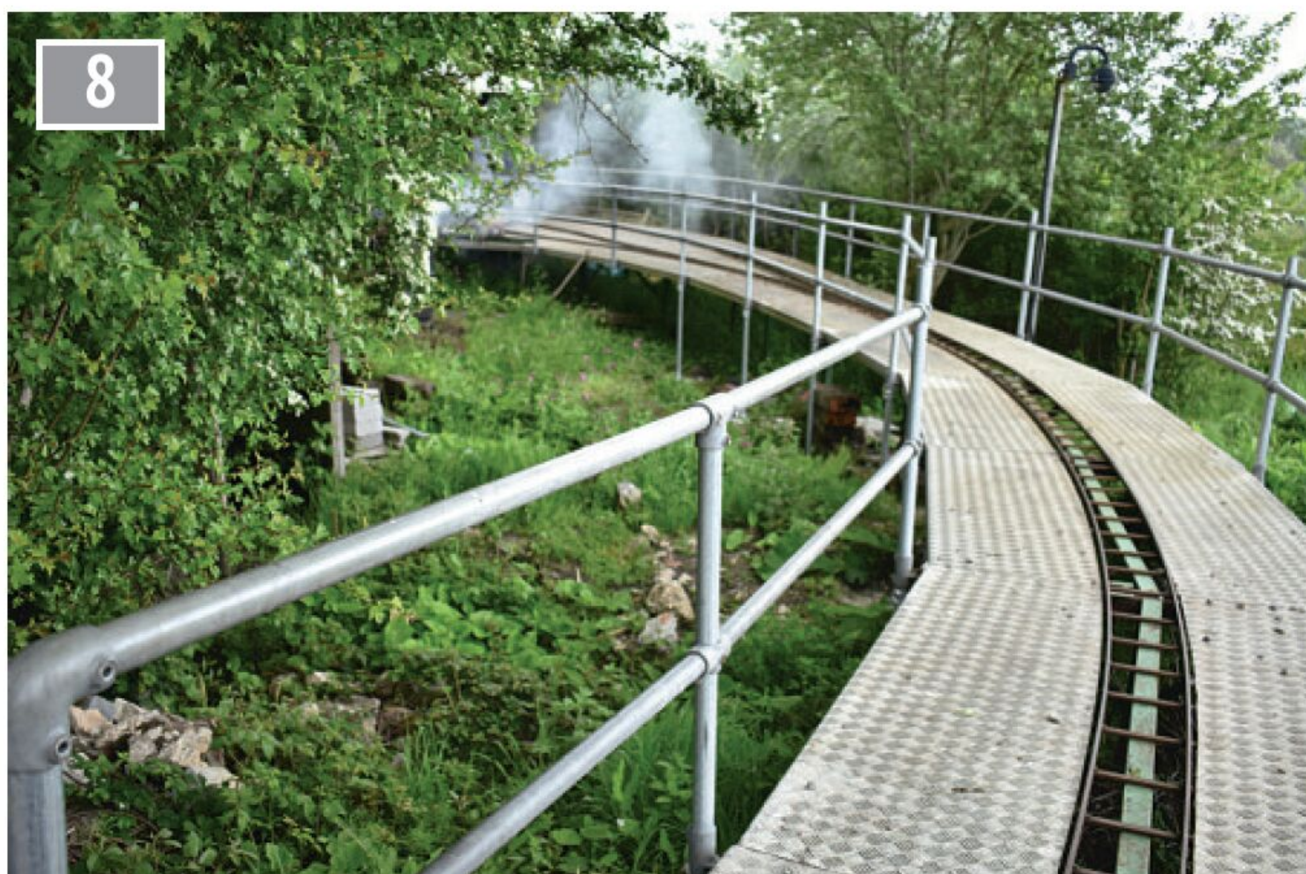
The well-built staging, supporting the track to the storage area. Gregg.
