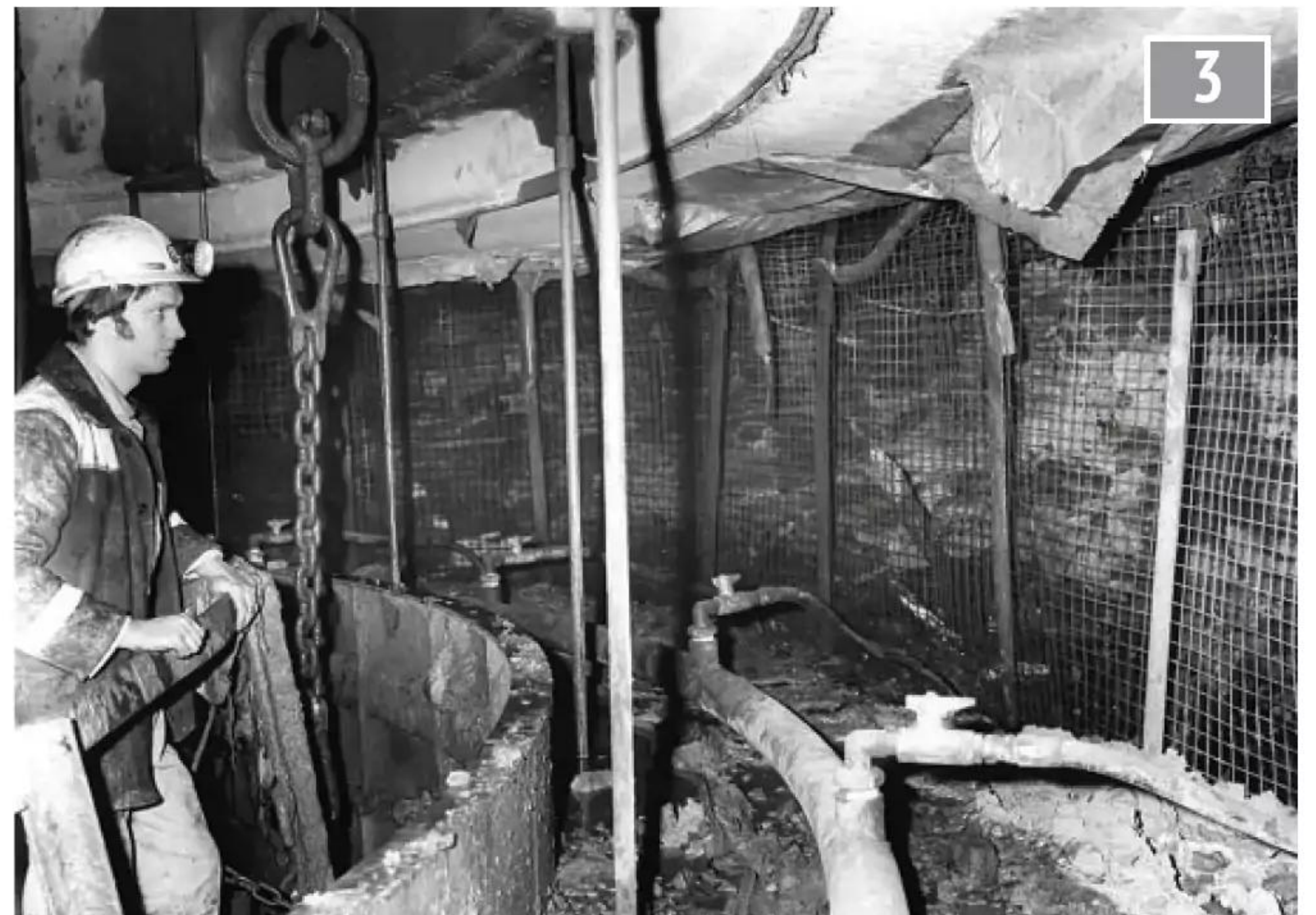
The shaft lining is 1m thick sulphate resisting concrete. Neil Rowley is standing on the top of the sinking stage.
