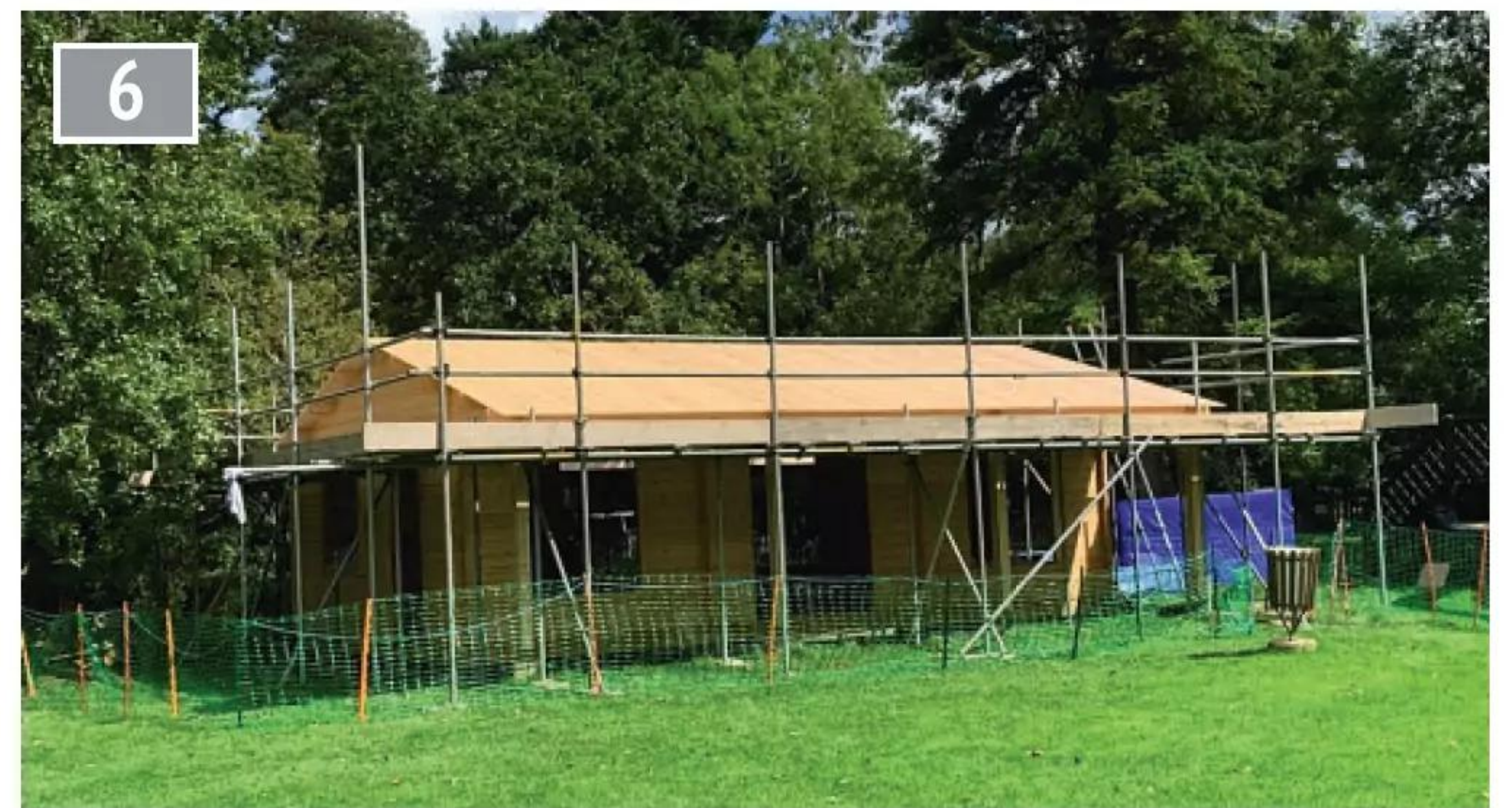
The roof goes on.
