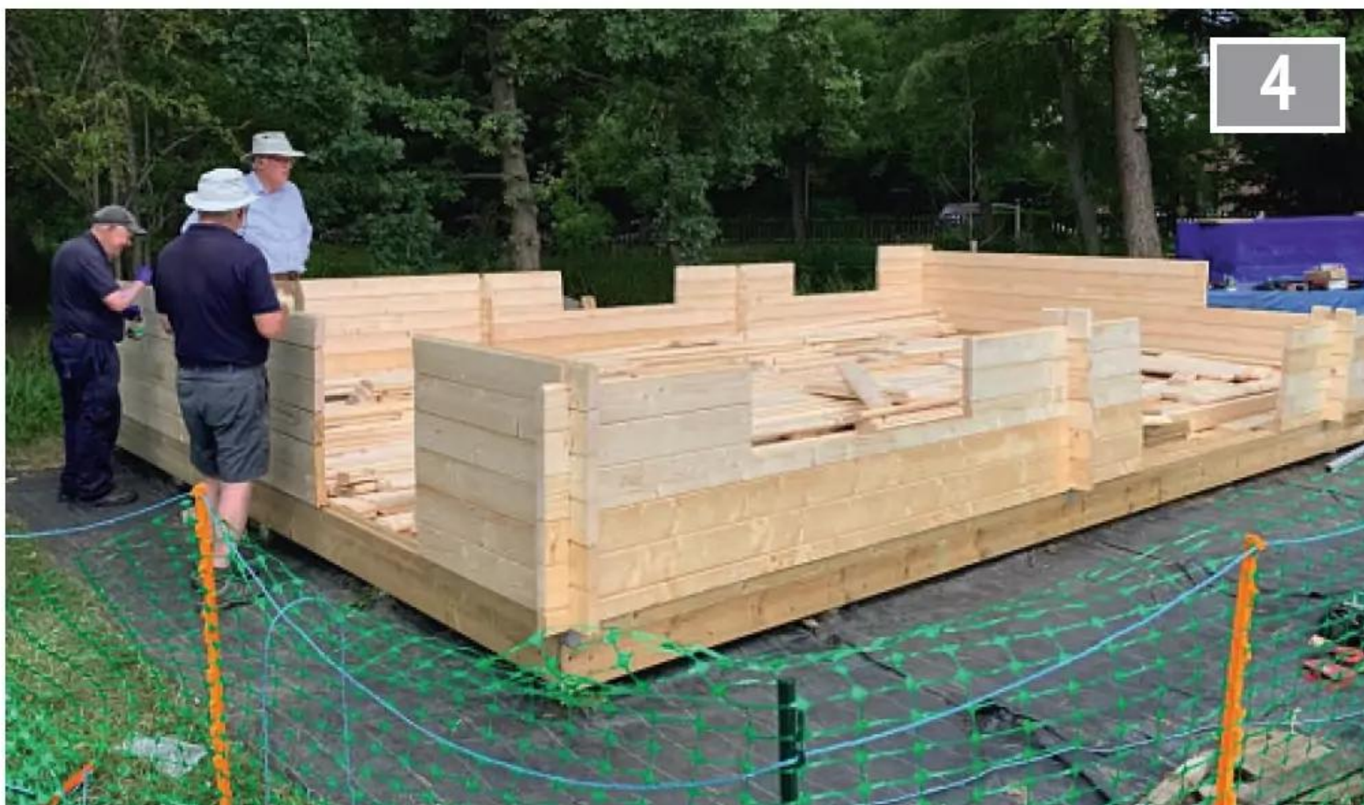
The new building rises from the ground.
