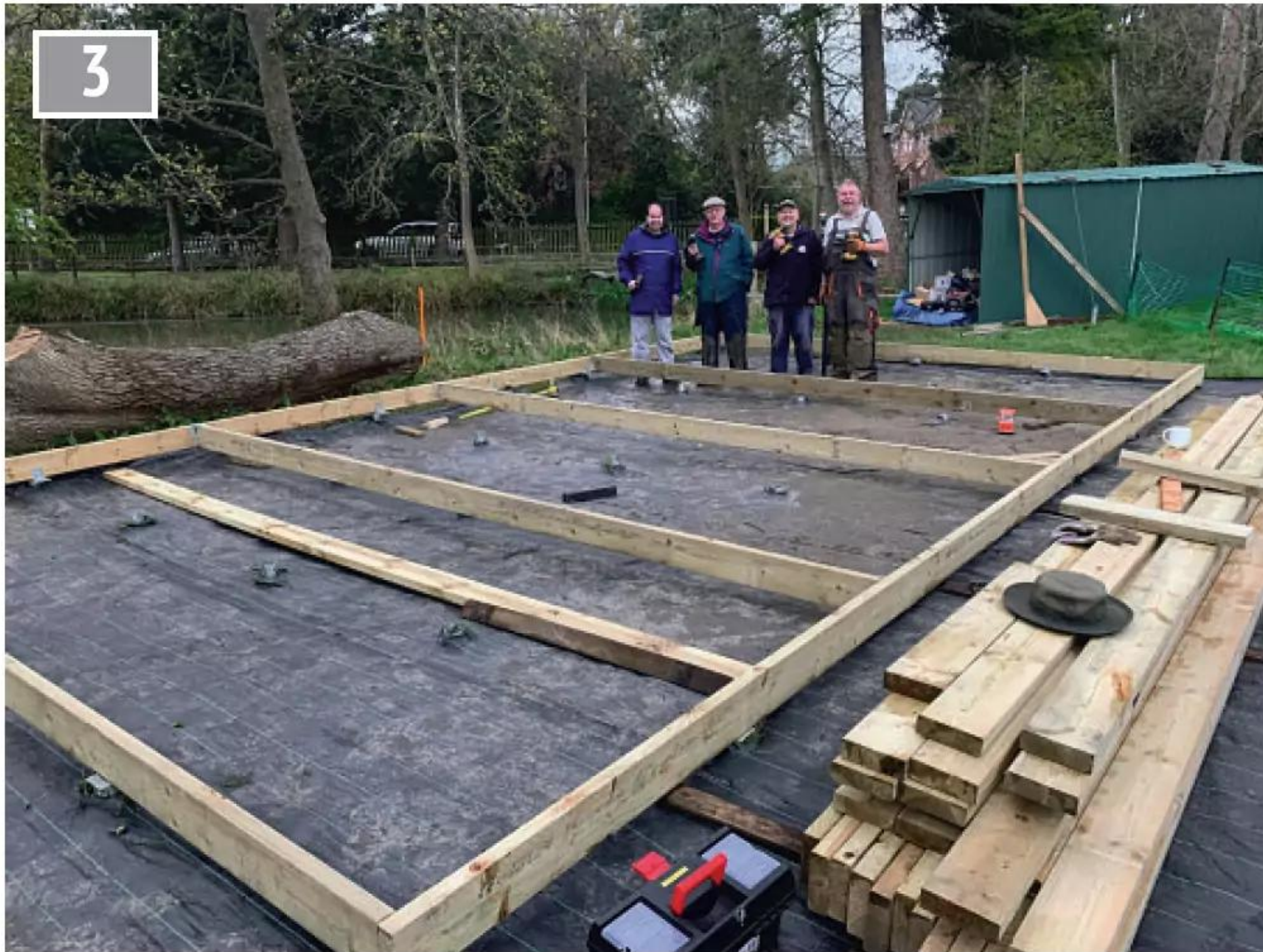
The frame under construction.
