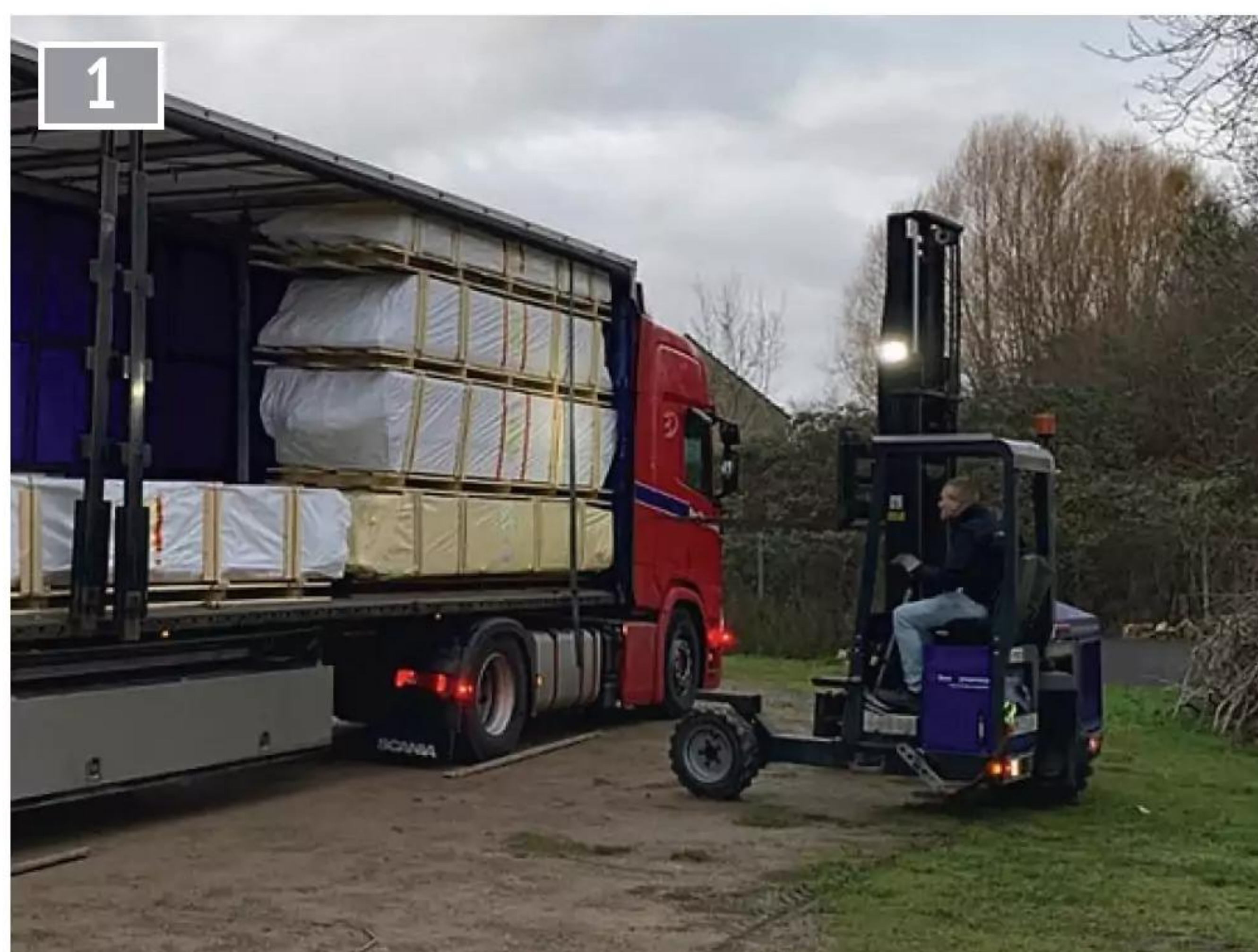
Unloading the new clubhouse.
