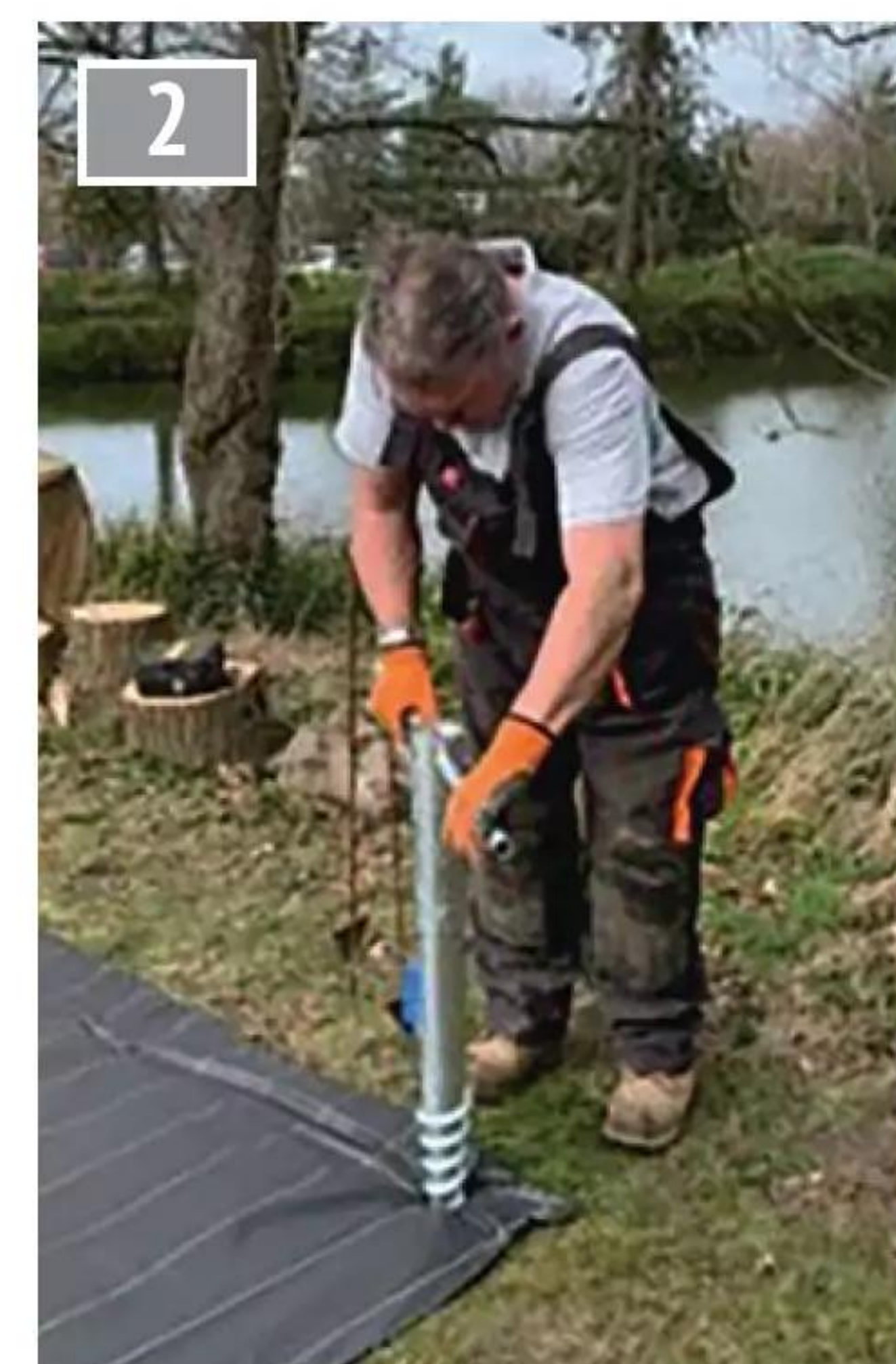
Putting in the first ground screw.
