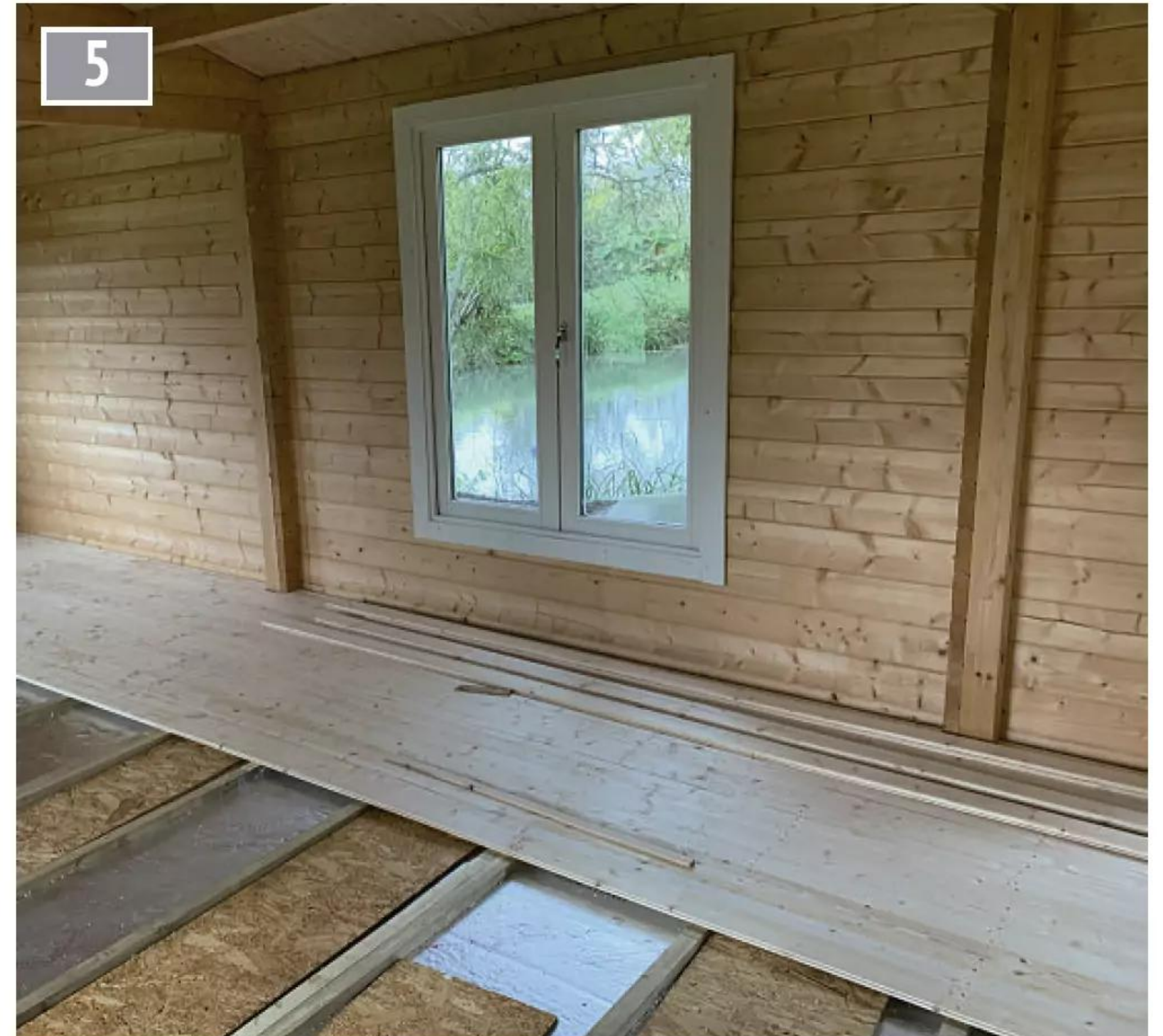
Putting in the floor.
