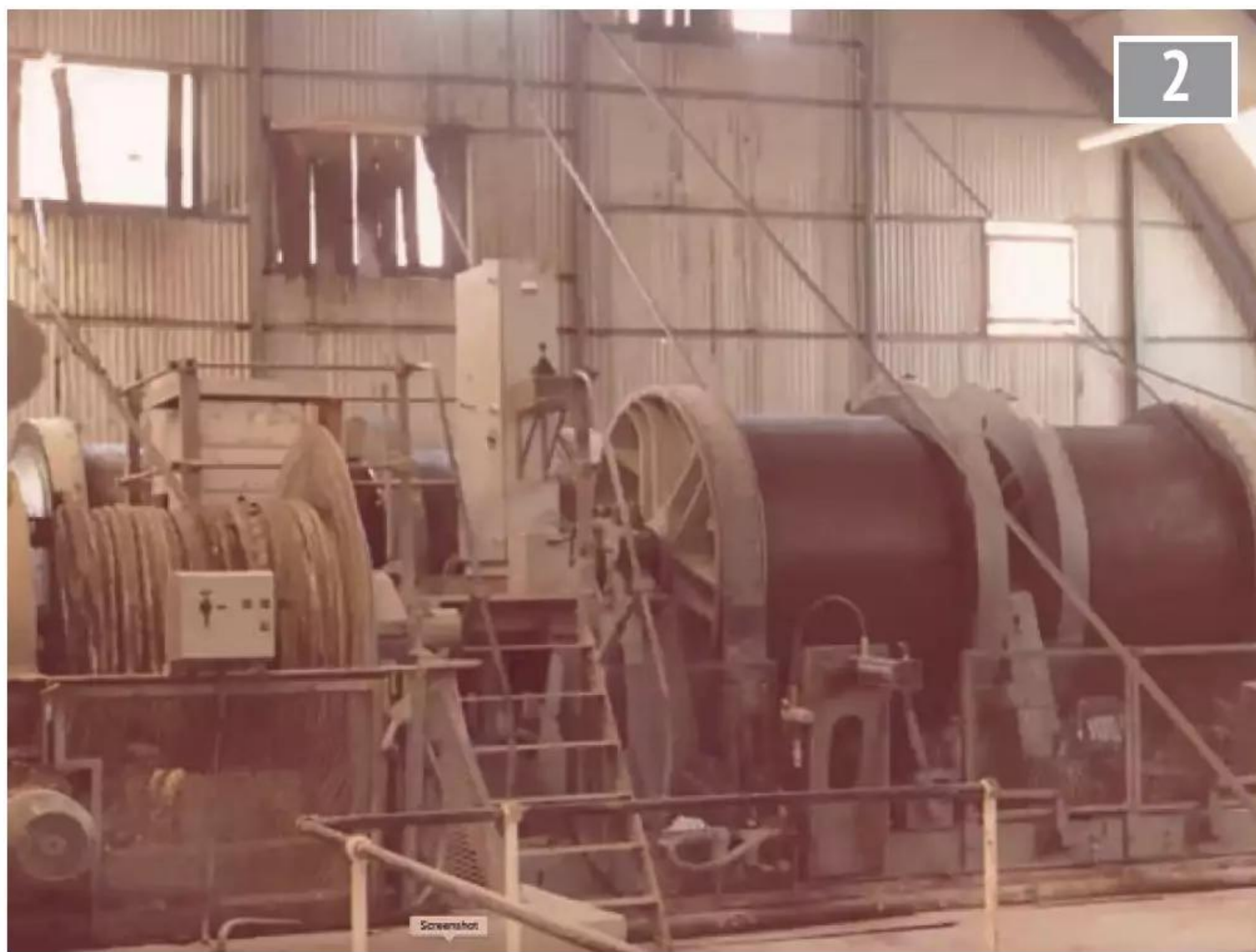
Power and telephone cable drums at the pithead and the normal winding engine.
