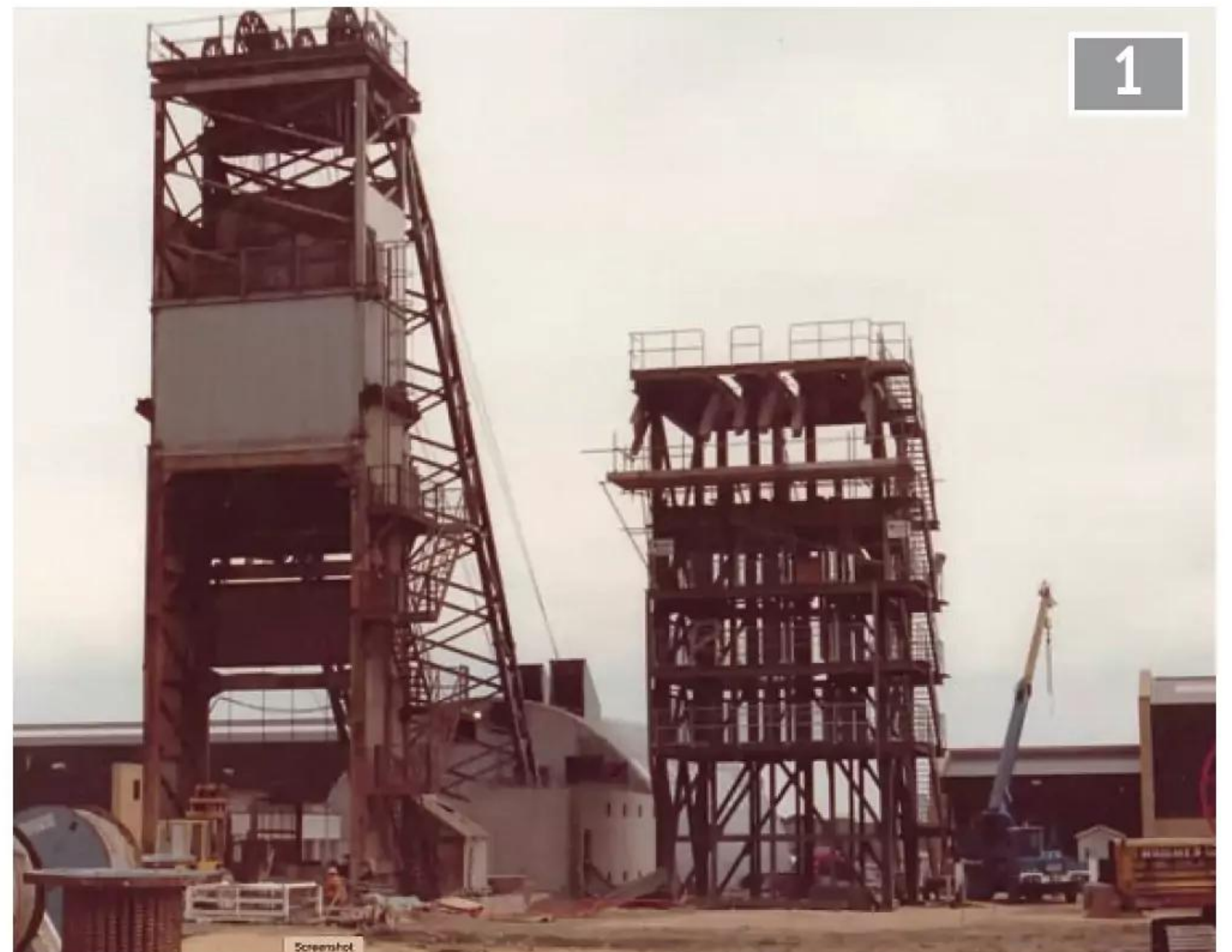
Four synchronised winches support the 5 deck sinking stage.
