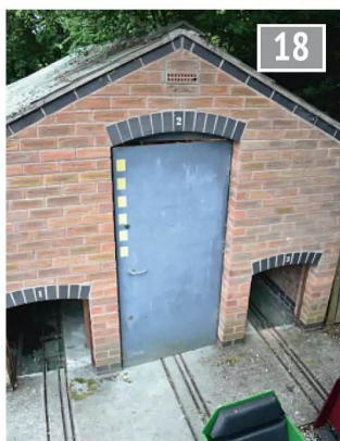
The front view of the substantial storage shed with ground level rail access.
