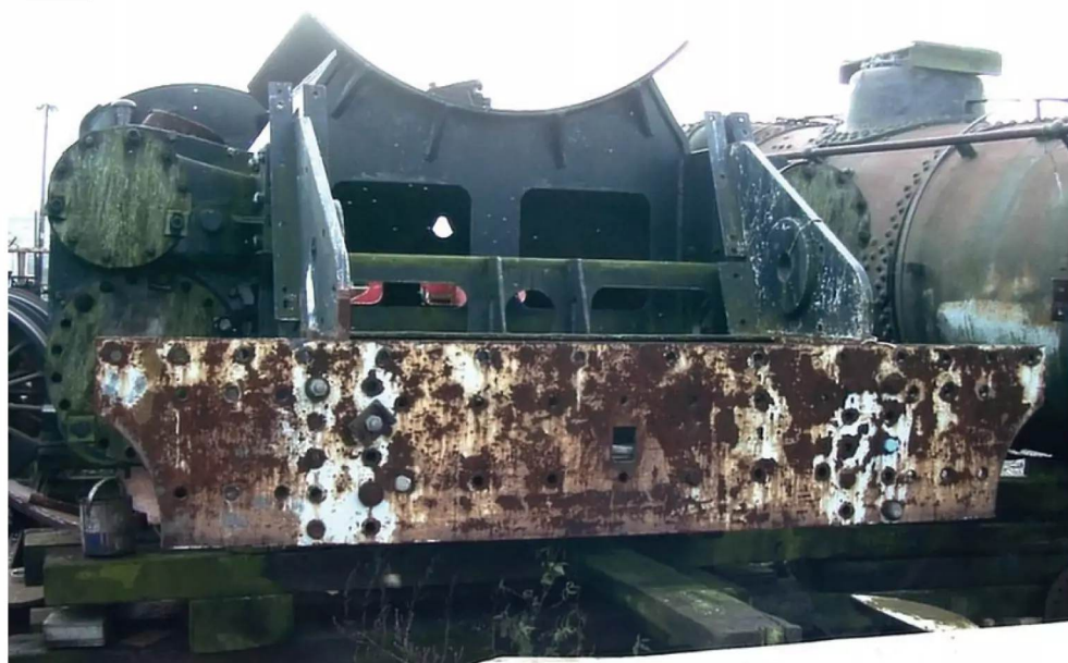
Front buffer beam and front plate of the saddle.
