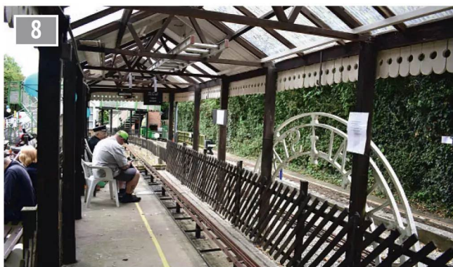
Inside the main station, looking towards the departure end.
