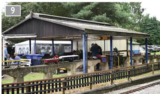
The large covered steaming bays for the elevated track.
