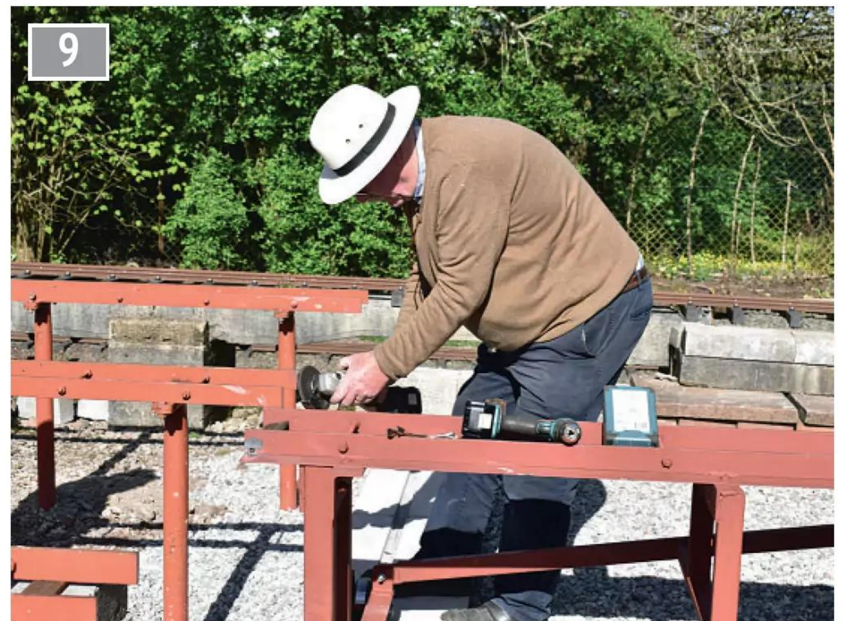
Eddie Attree working on the new carriage shed traverser.
