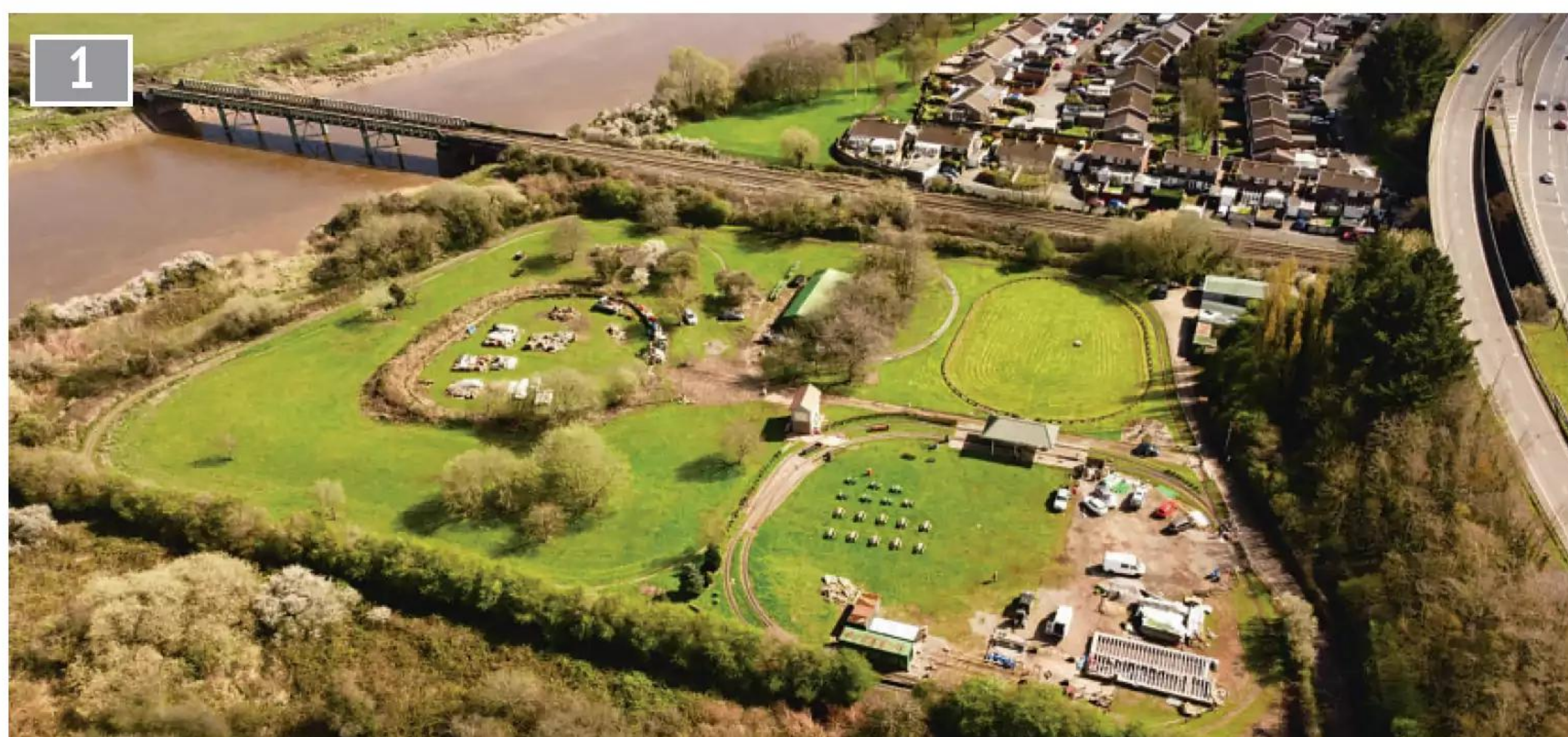
Aerial view of the current Glebelands site.
