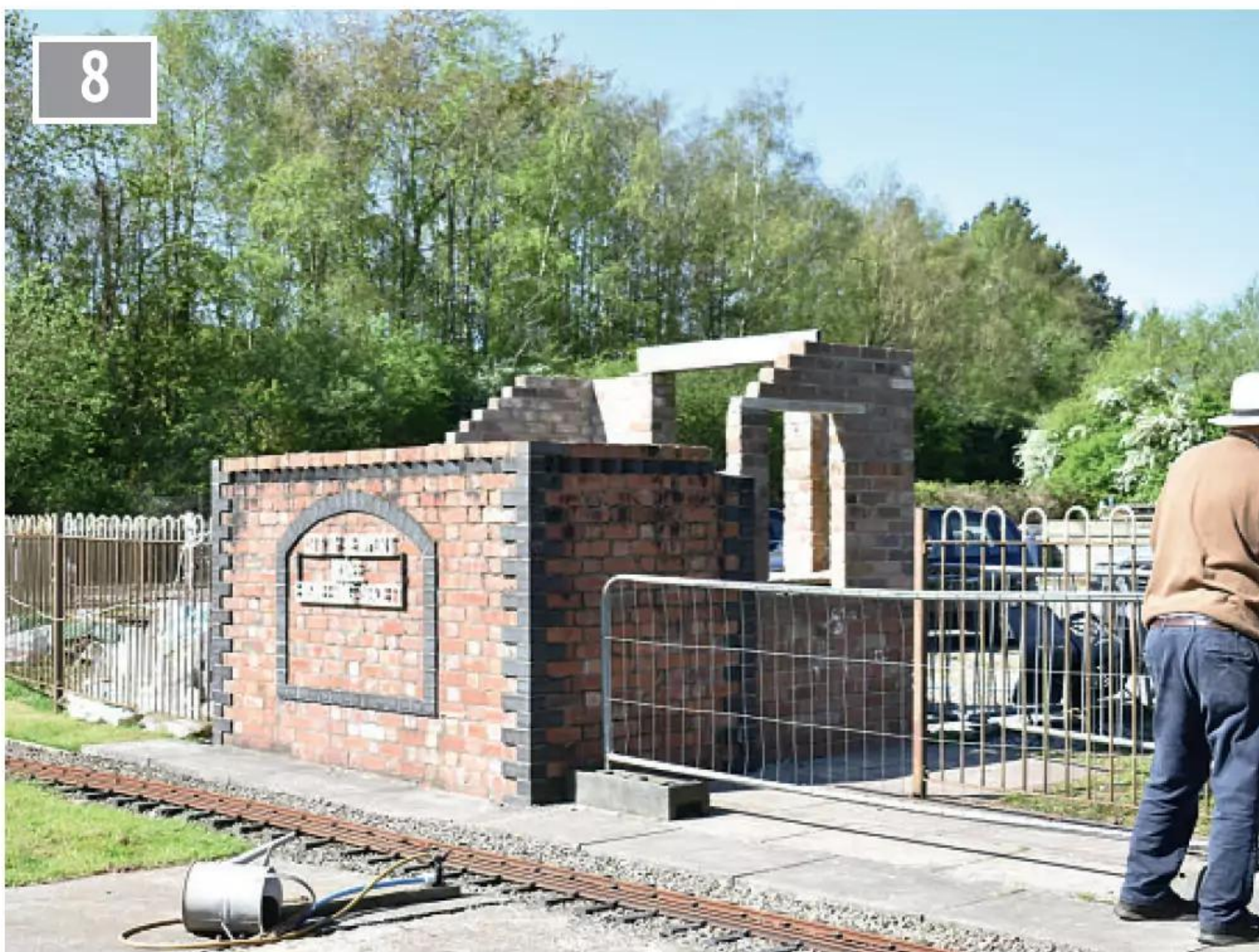
Work on re-building the old water tank support into a ticket office.
