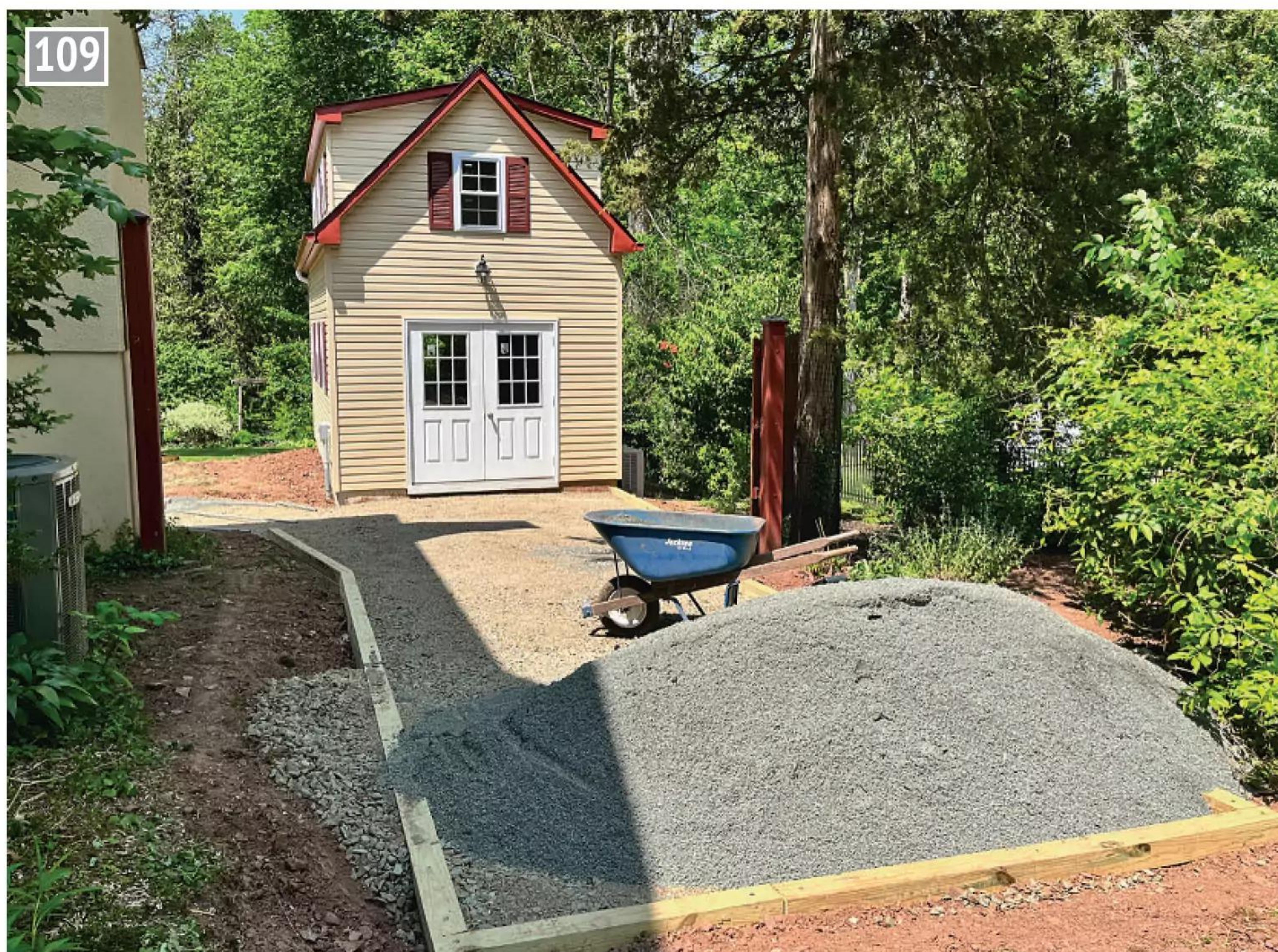
The patio base, completed by hand following a half-day of mechanical-digging terror.
