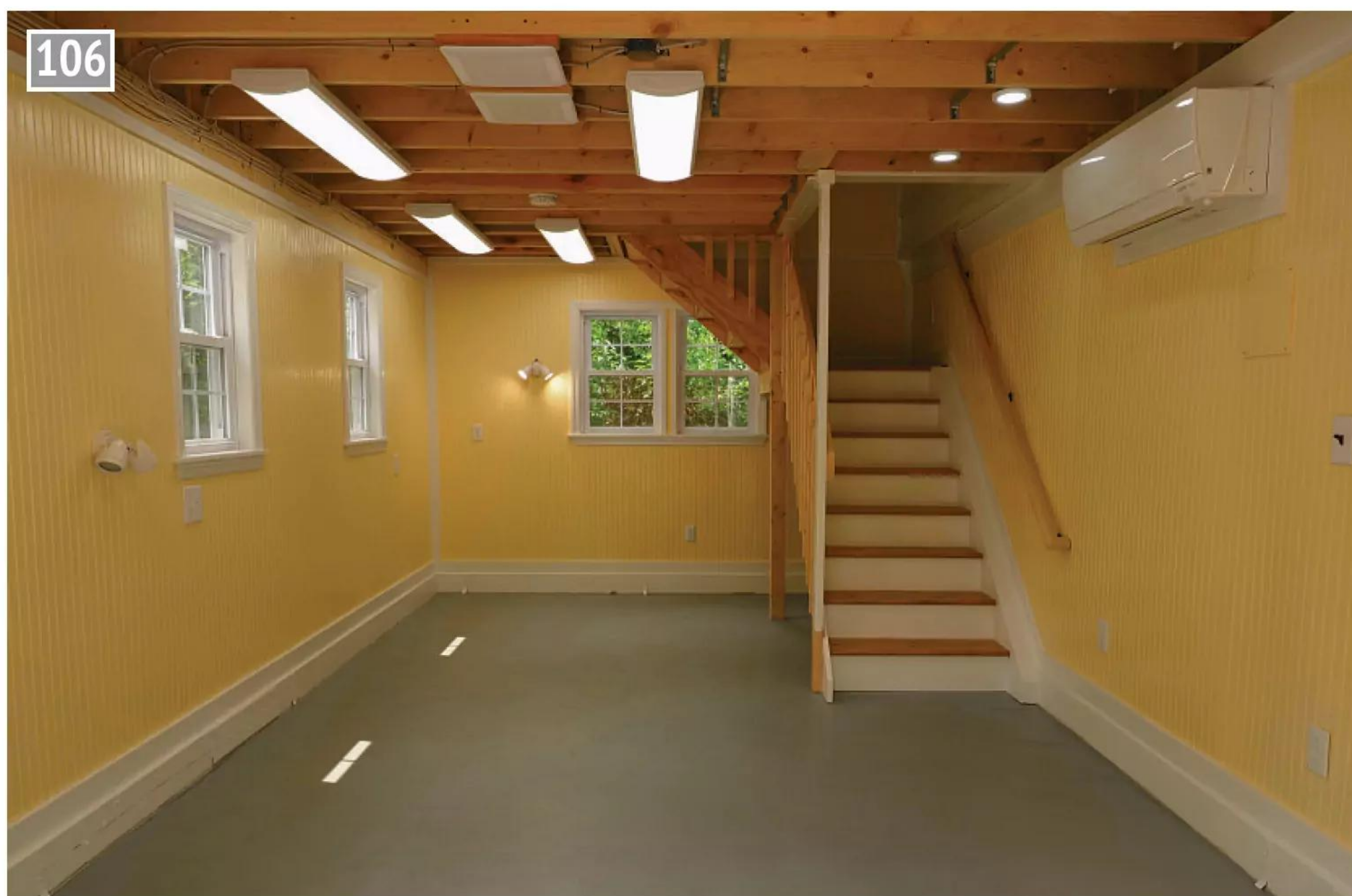
In the eventual workshop, plywood beadboard provides both a knock-resistant perimeter and a sturdy substrate for the shelving to come.
