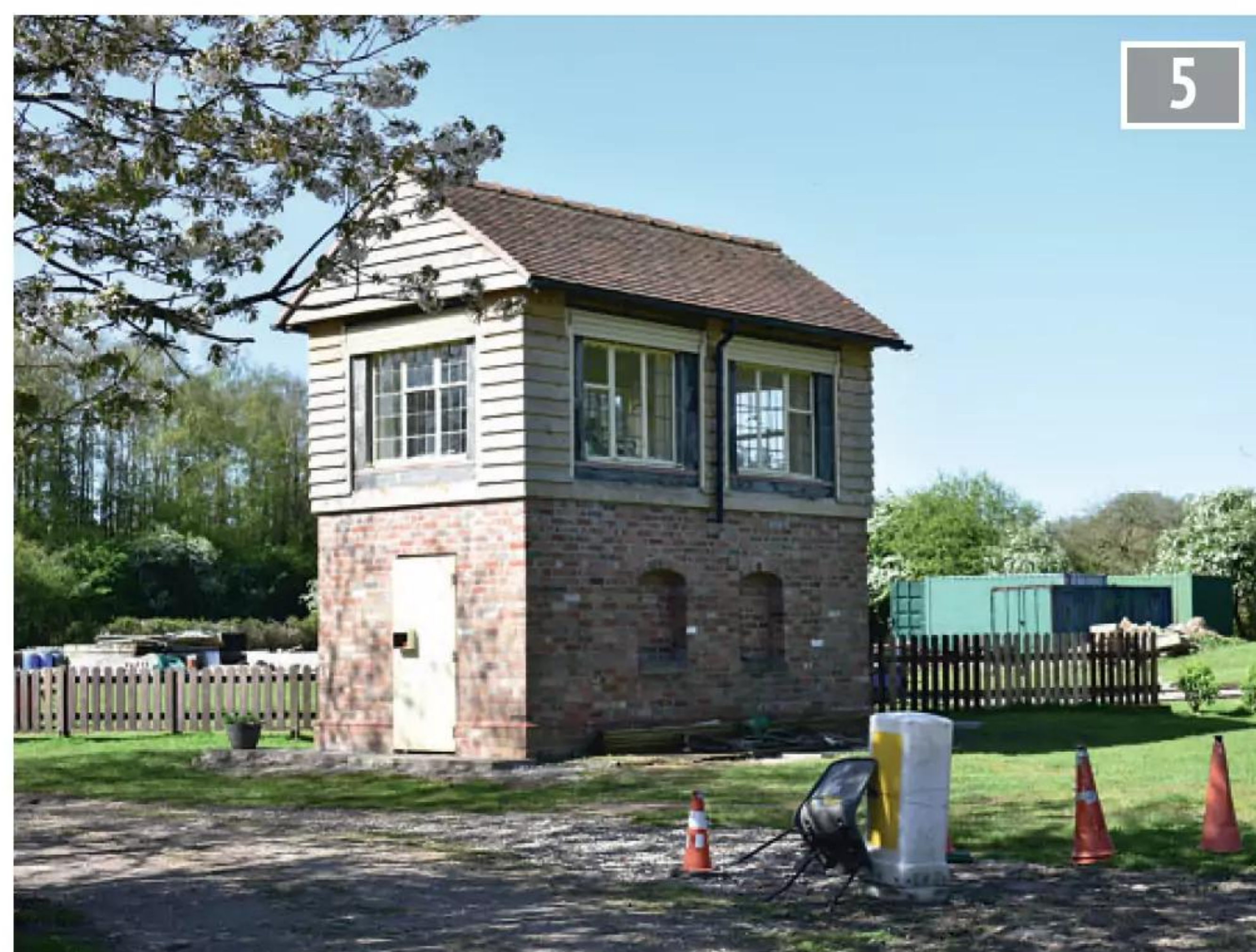
The new signal box with the protective roller shutters in the working position.
