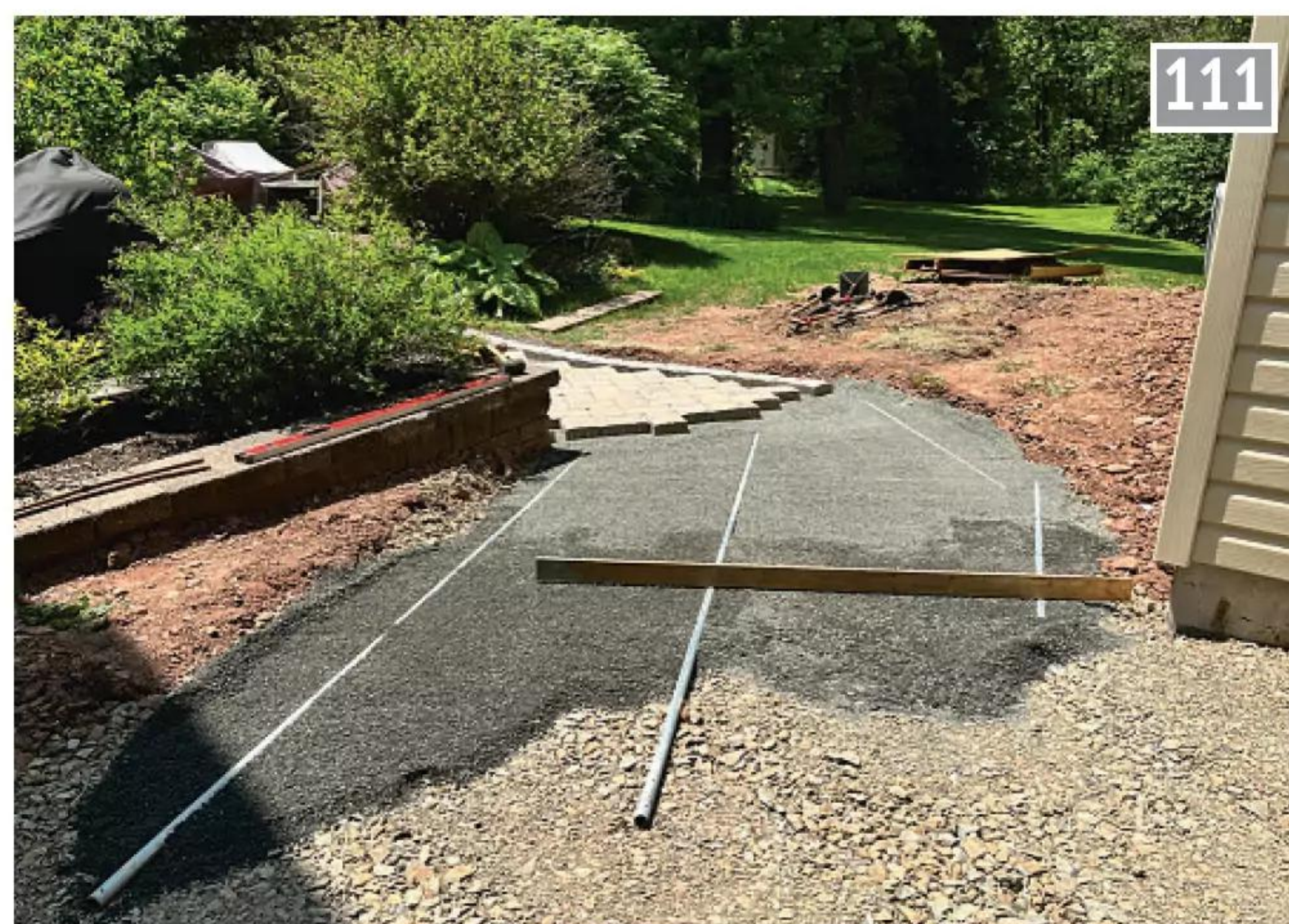
A few lengths of galvanised pipe and a straight-sided screed board help create a carefully contoured bed for the patio pavers.
