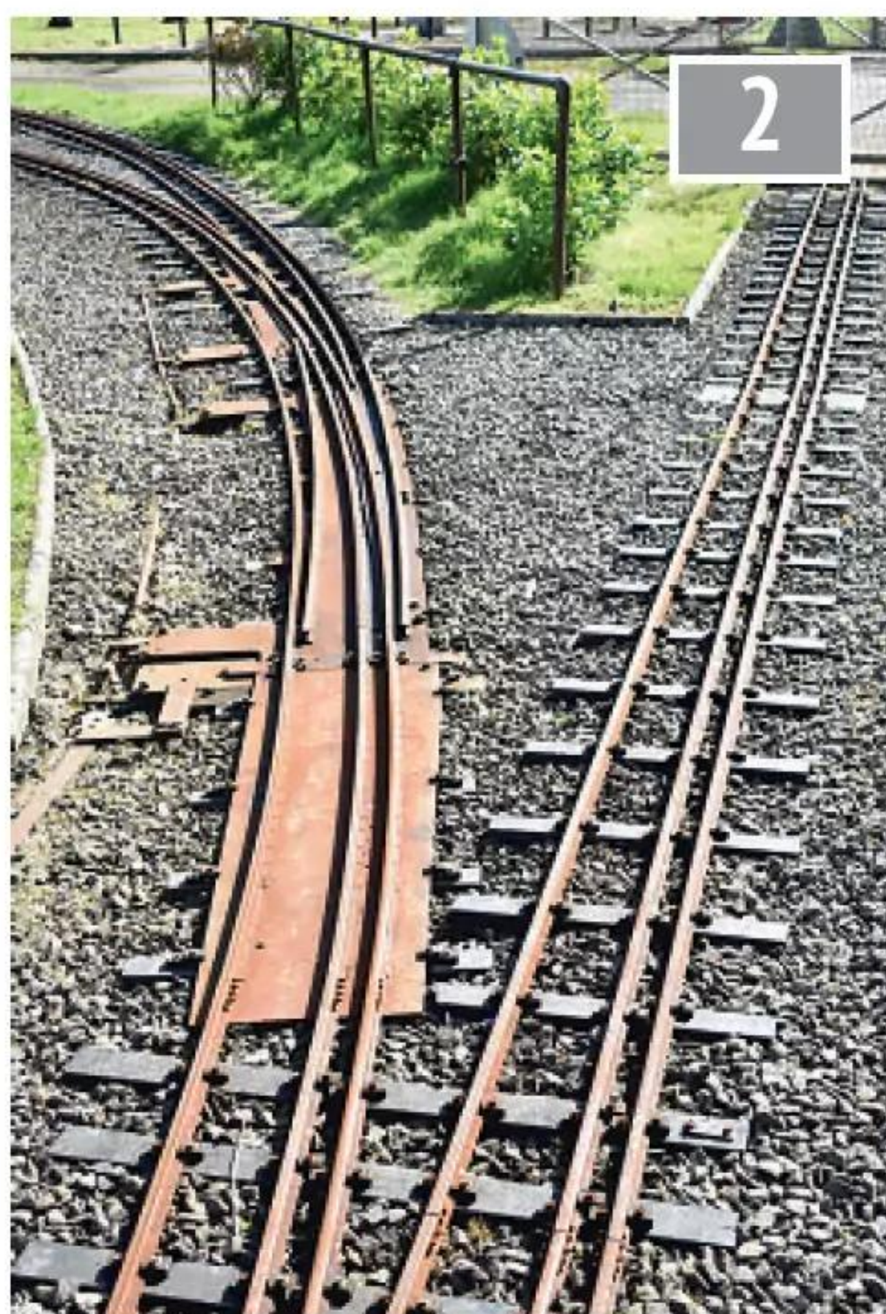
One of the new self gauge widening turnouts.
