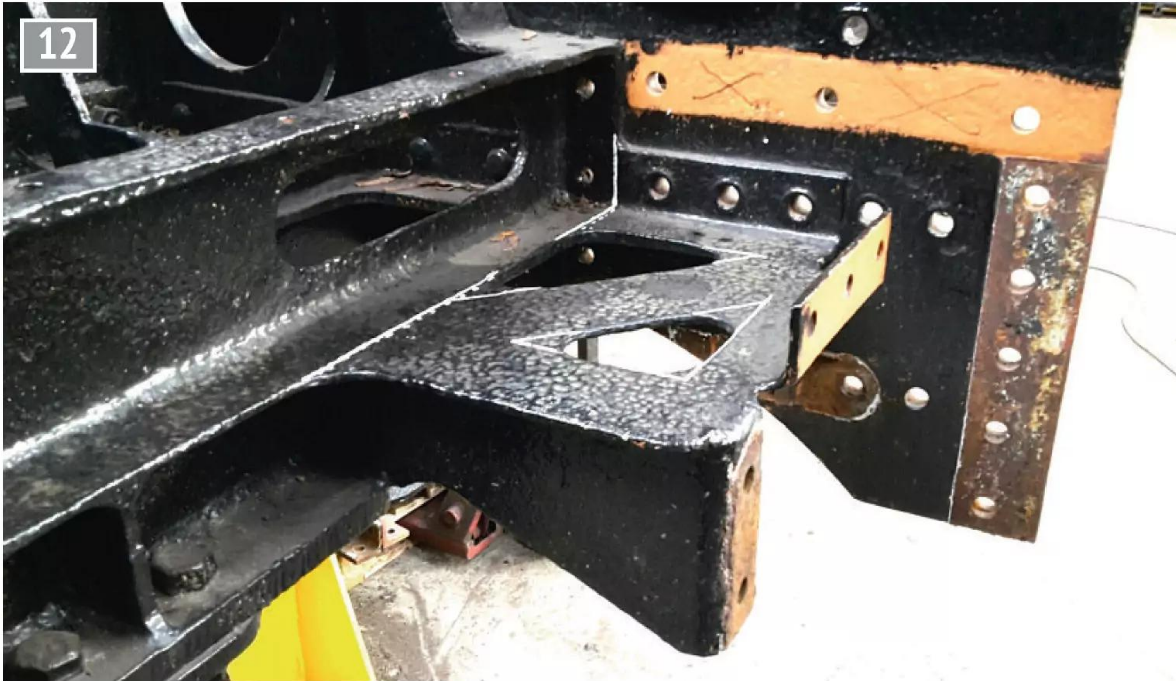
Frames – front left-hand corner. photo: Gloucestershire and Warwickshire Railway
