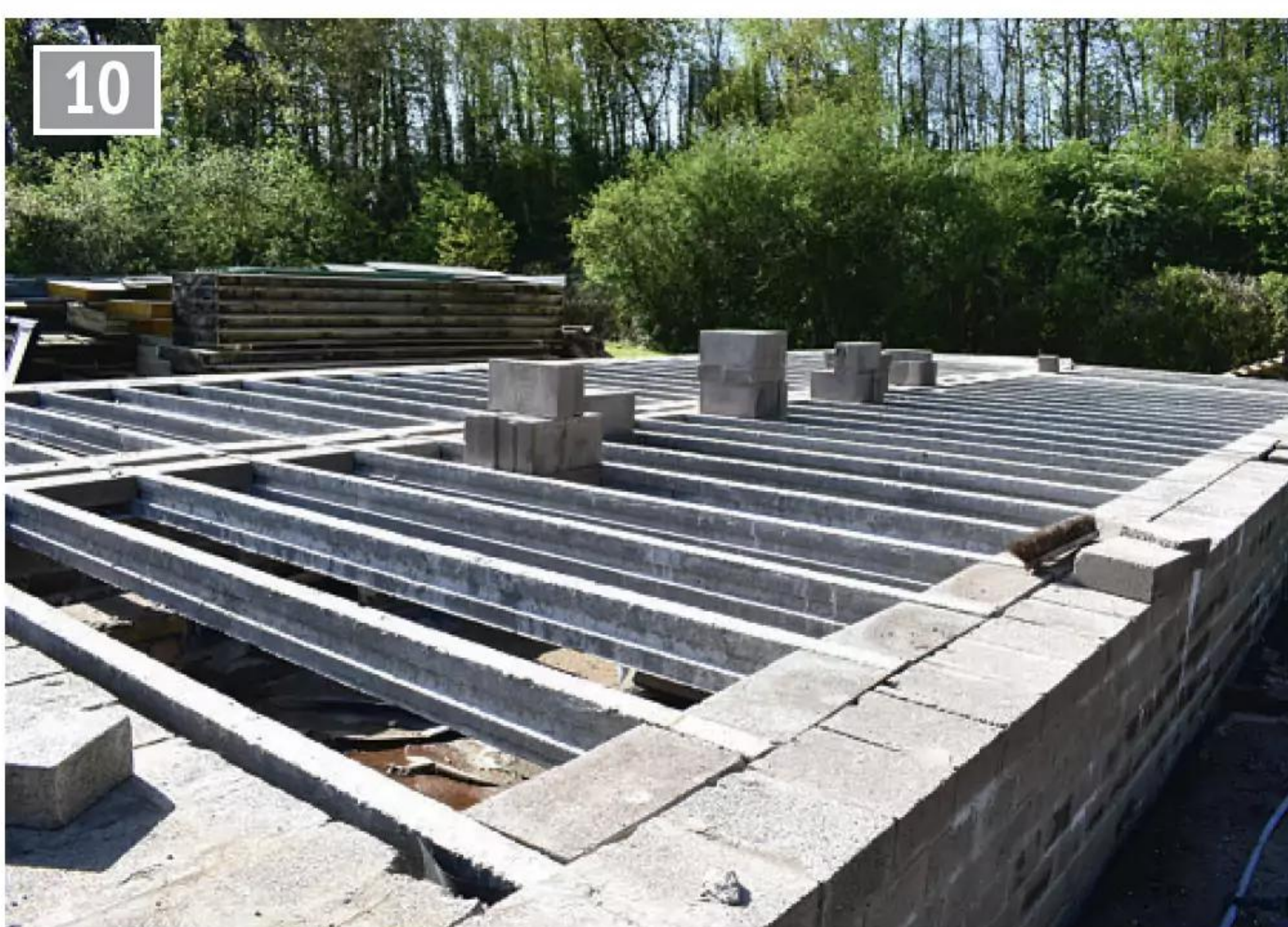
Substantial foundations for the new engine shed.
