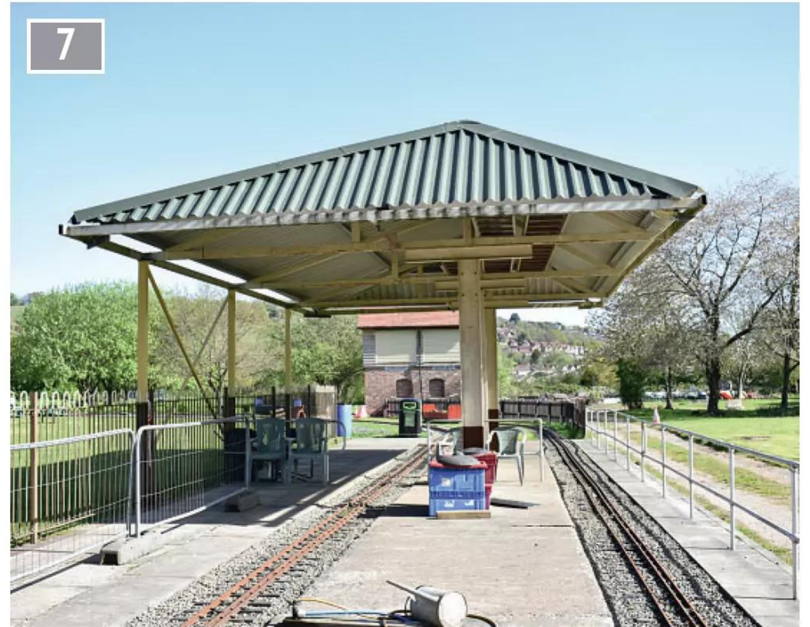
A view of the main station with its splendid new roof structure.
