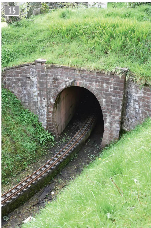
The entry portal for the inner tunnel.
