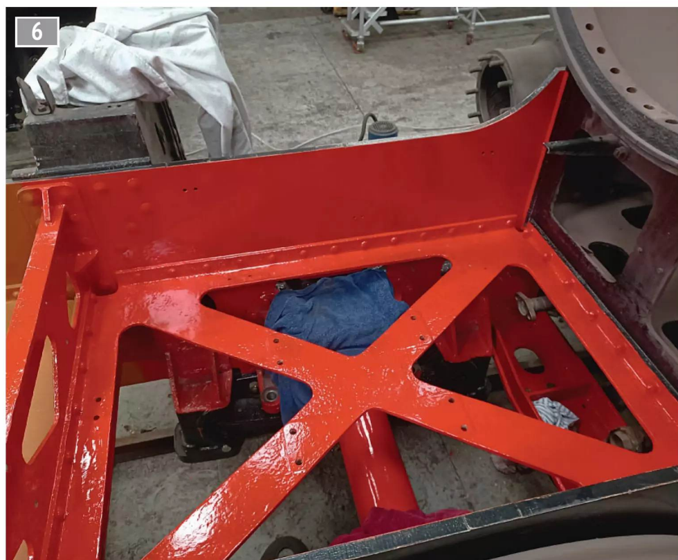
Frame stretcher on 76077, also freshly painted.
