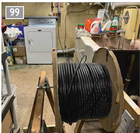
99 A hefty drum of wire rests on two sawhorses, the free end inserted into the grey conduit beyond, all ready for the first pull.
