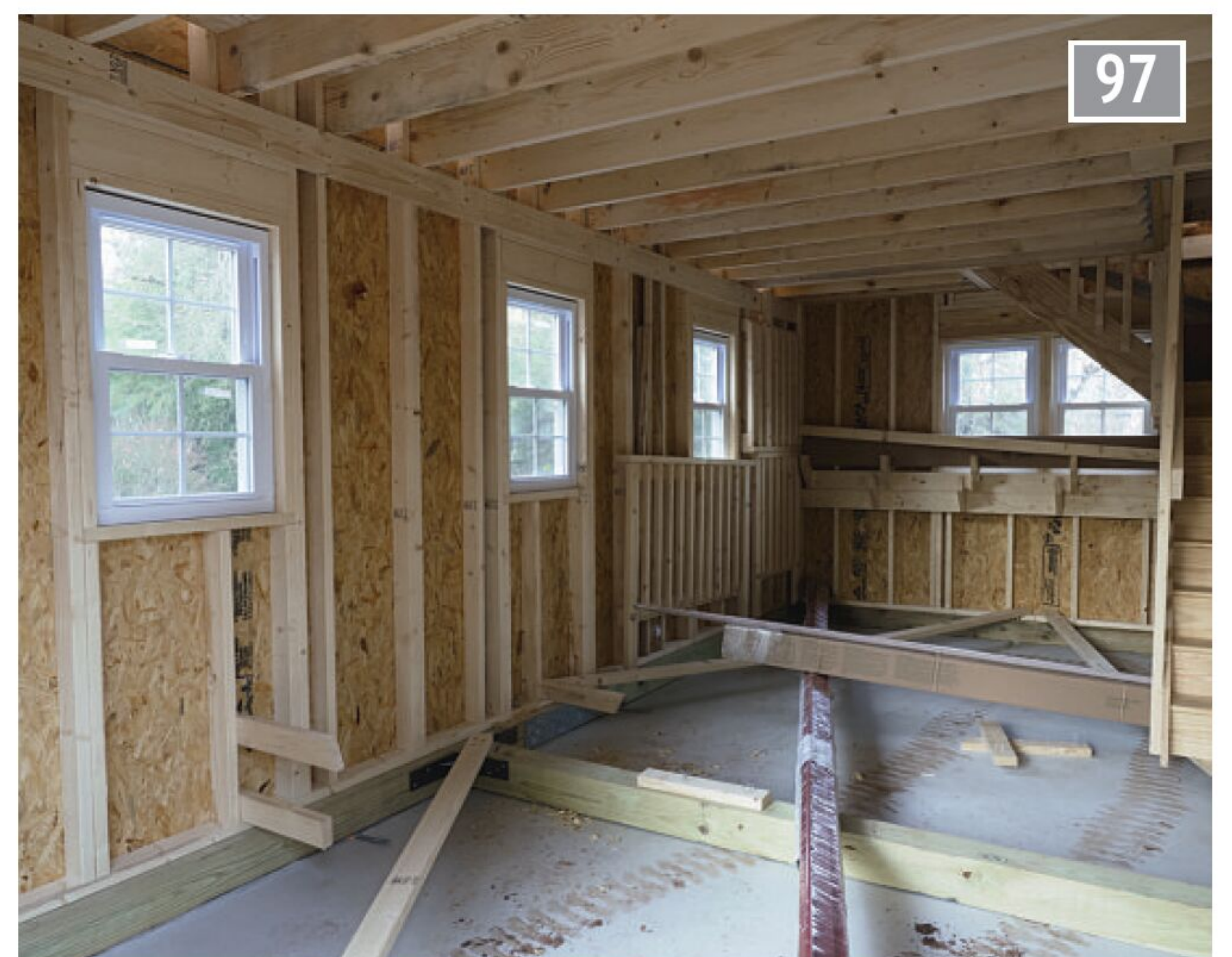
Within the shed, substantial cross-bracing kept everything ship-shape during the shed's long interstate journey and much shorter mule ride.
