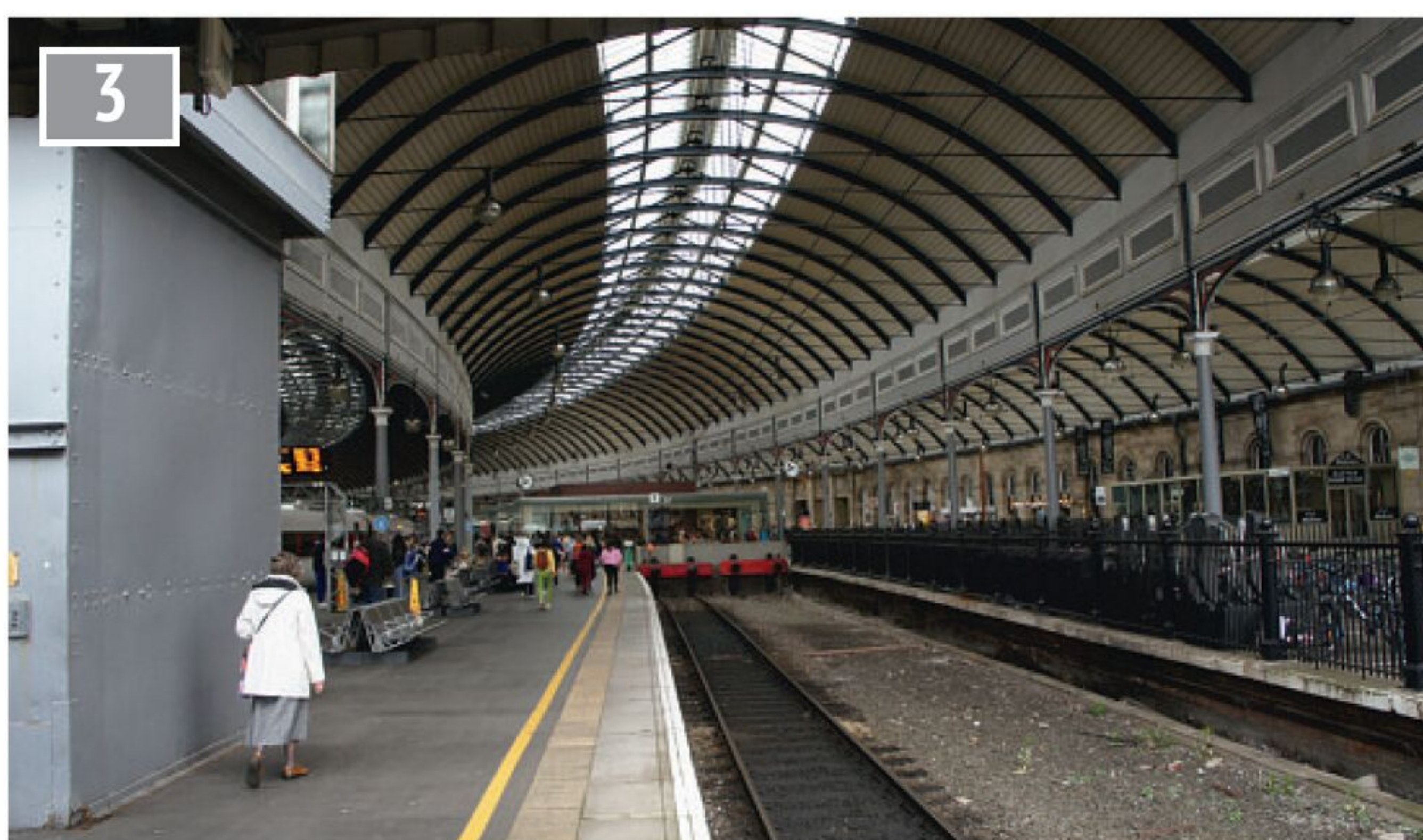
Newcastle Central Station has a magnificent overall roof.
