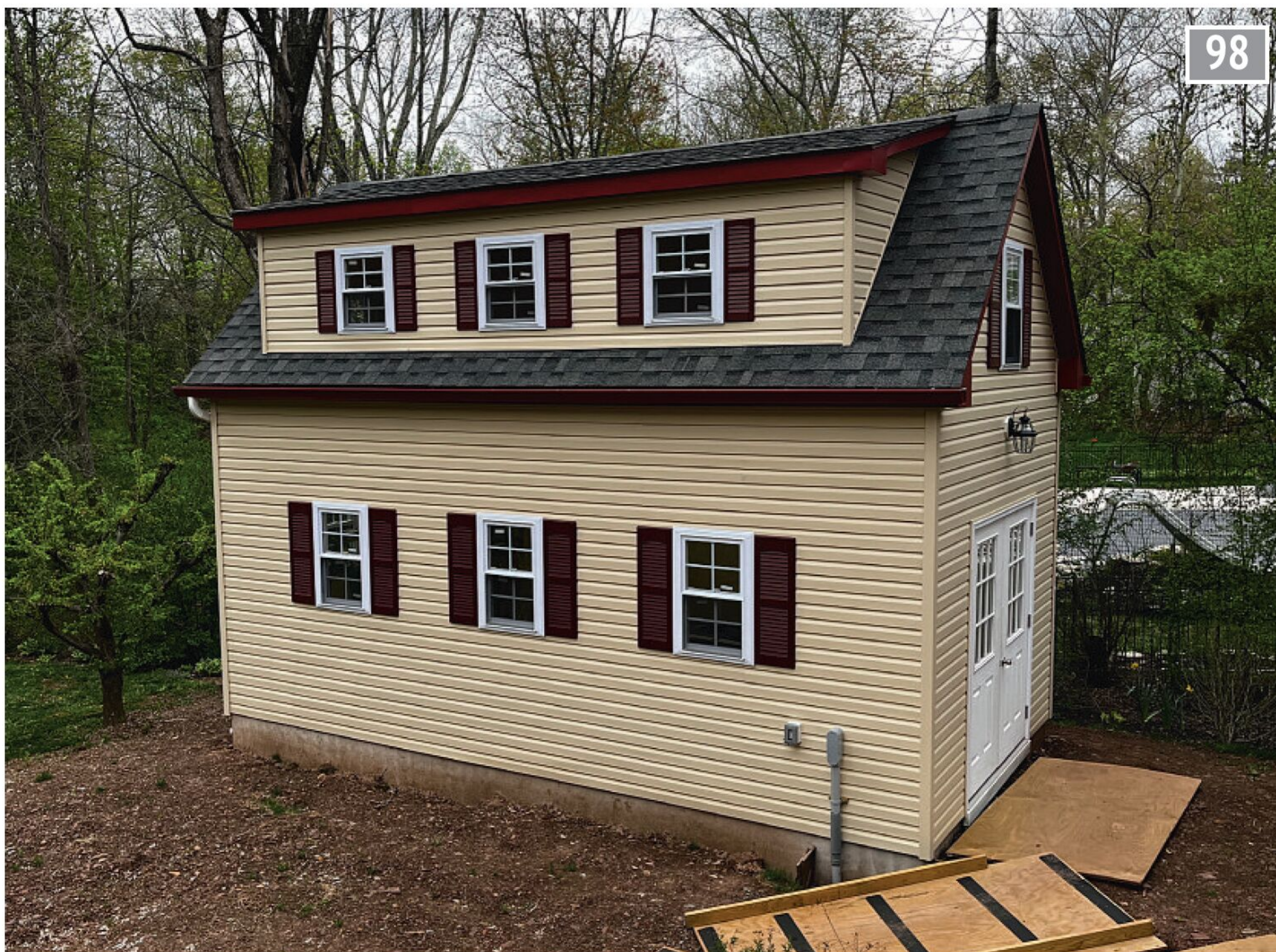
Although depicted a few months later with the electrical system by then installed, forty-eight hours after its November arrival the shed was externally complete!
