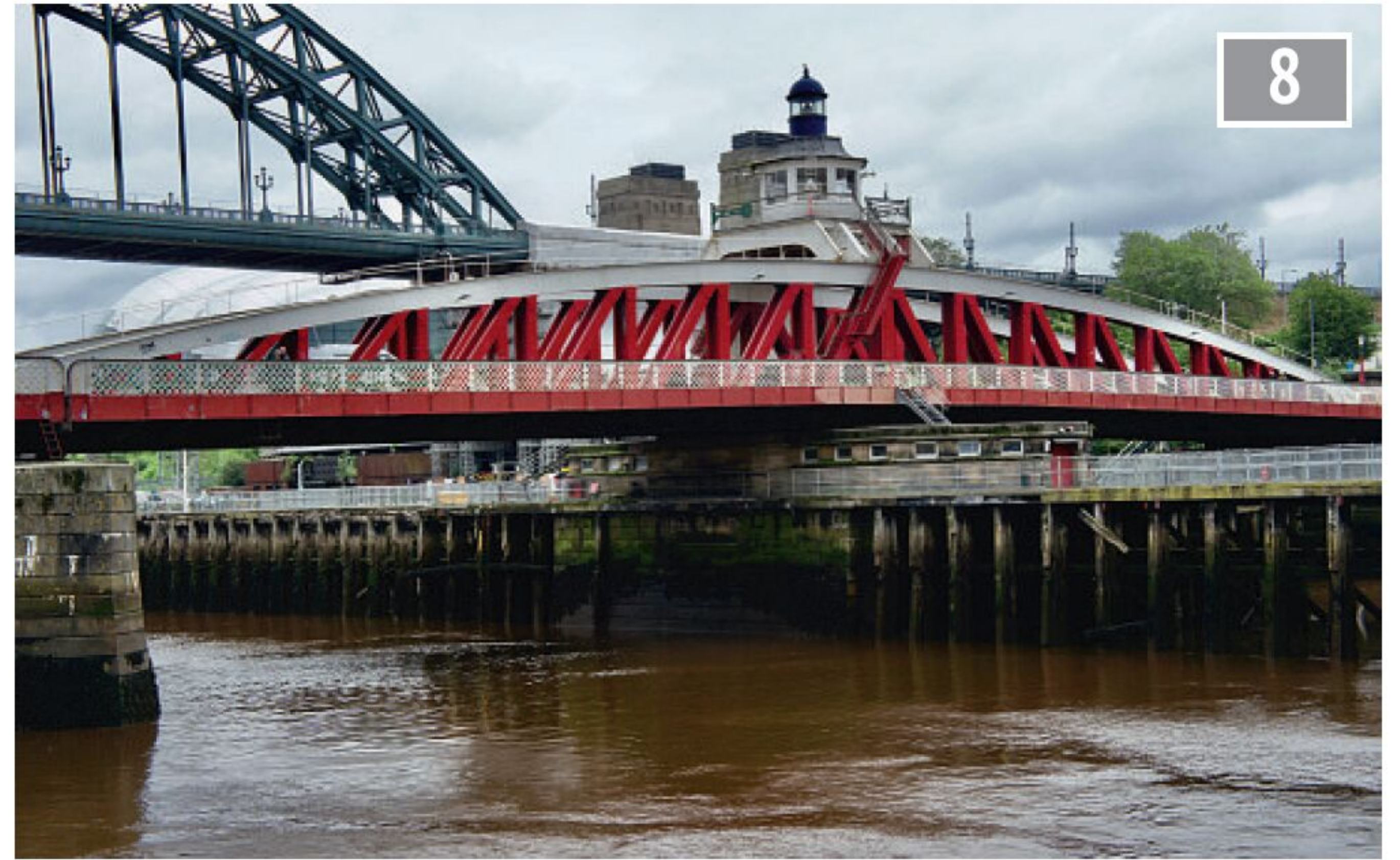
8 The Swing Bridge, opened in 1871, still uses the original Armstrong built hydraulic machinery.
