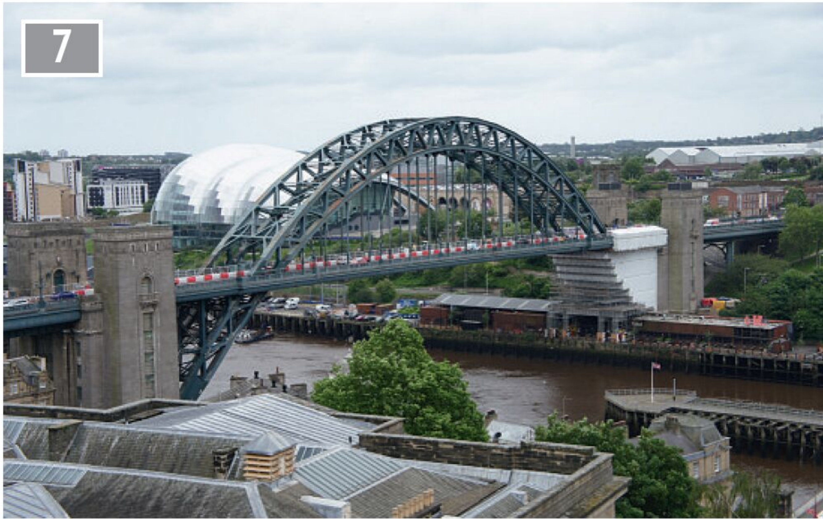
7 Tyne Bridge opened in 1928. Although not the prototype for Sydney Harbour Bridge it used the same construction techniques.
