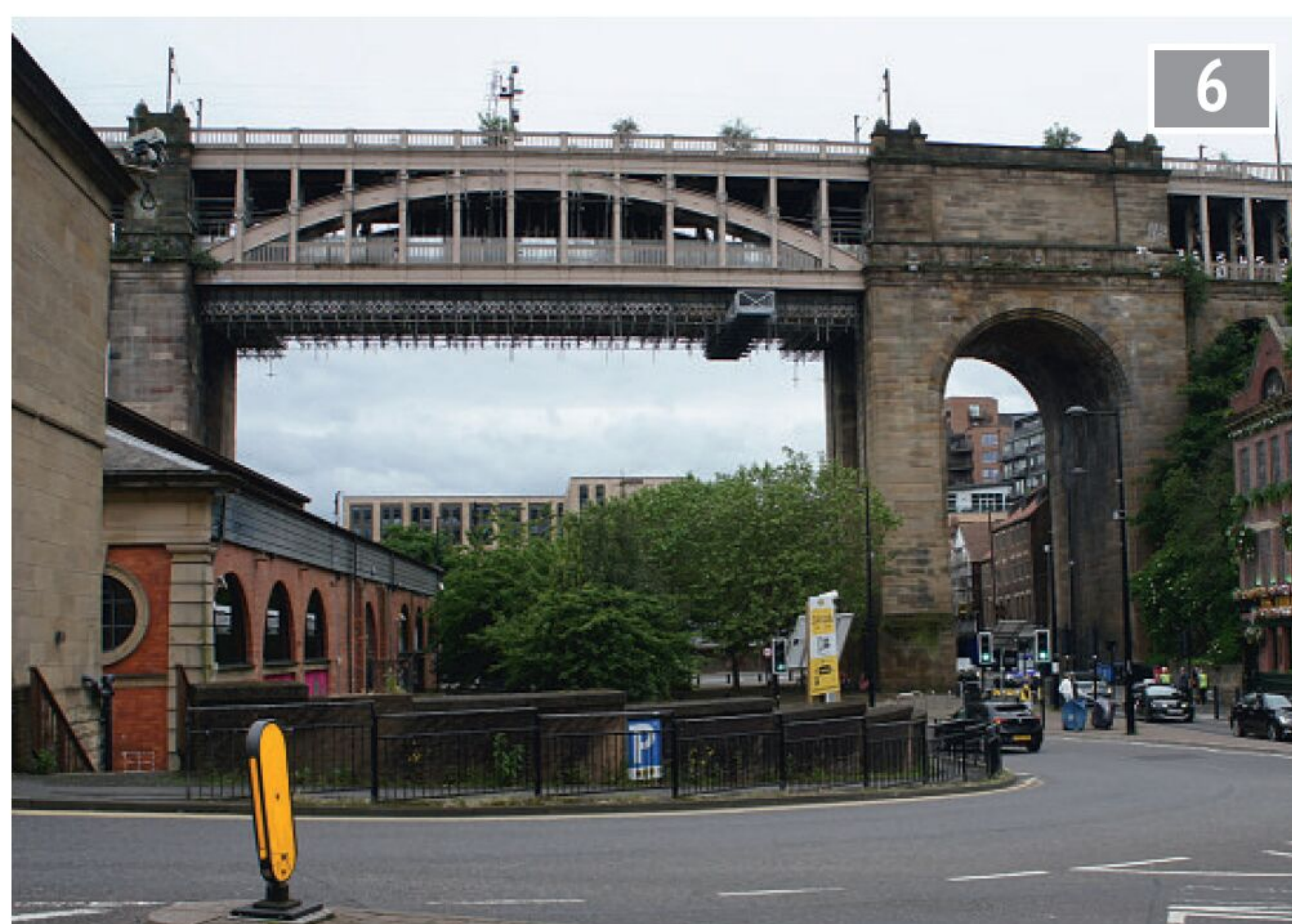
High Level Bridge span seen from the riverside Two decks carry road and rail traffic.
