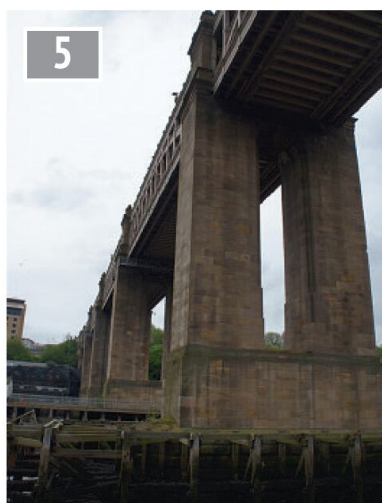
High Level Bridge pillars are hollow to save weight. They are made of ashlar built on wooden piles driven into the river bed.
