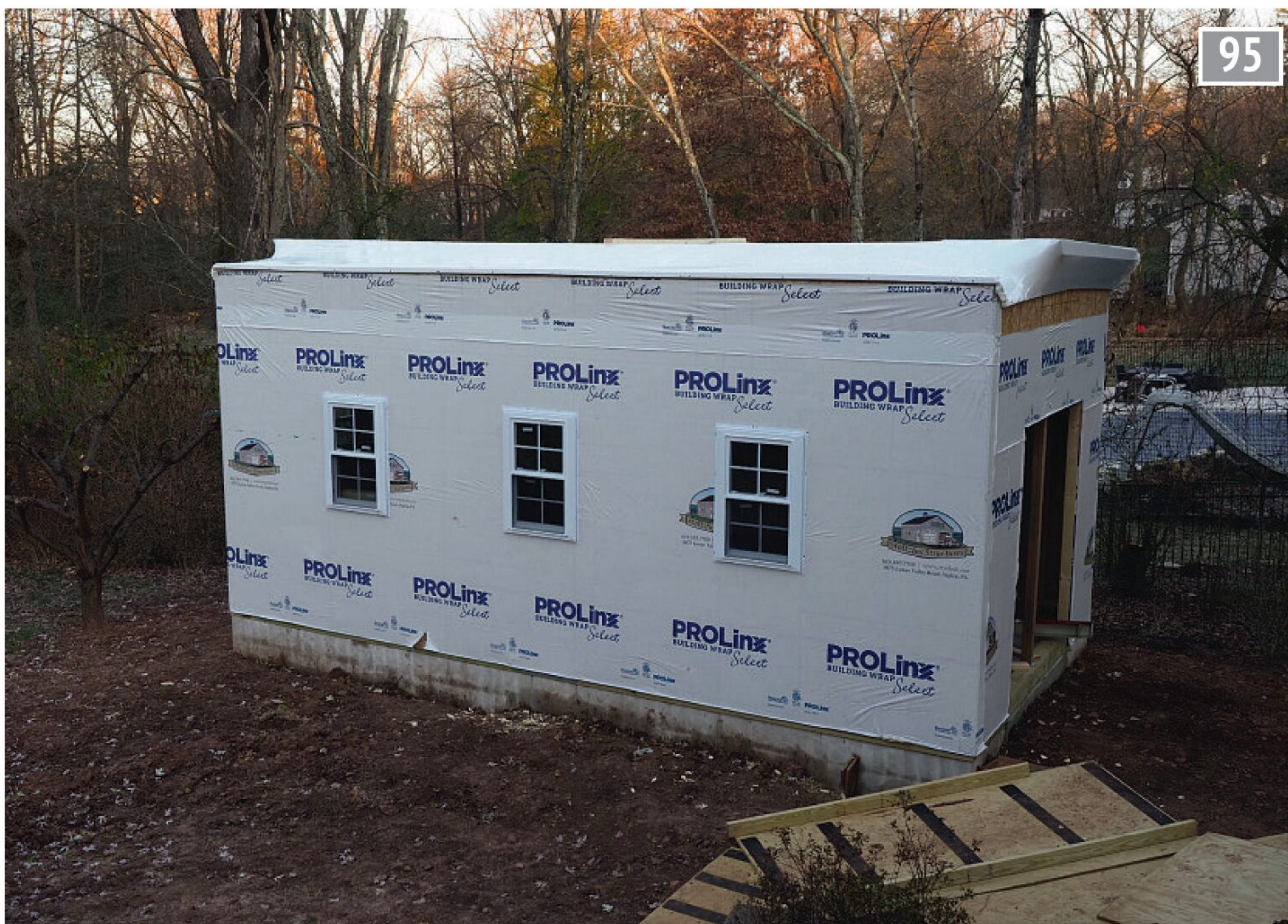
The newly arrived shed, bearing a disturbingly single-storey appearance.
