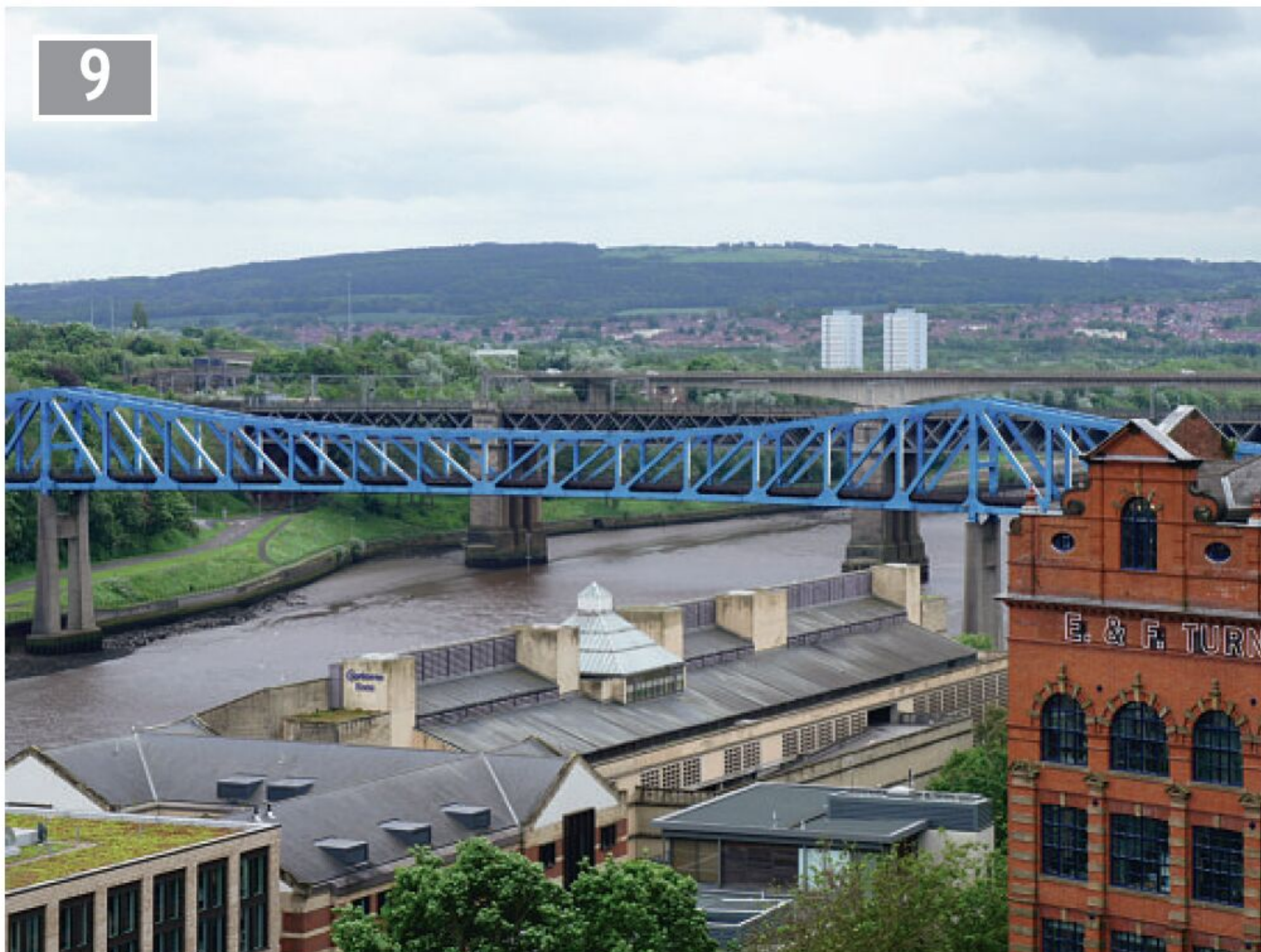
9 The Metro bridge seen from the castle keep with the King Edward VII rail bridge and Redheugh road bridge just beyond.
