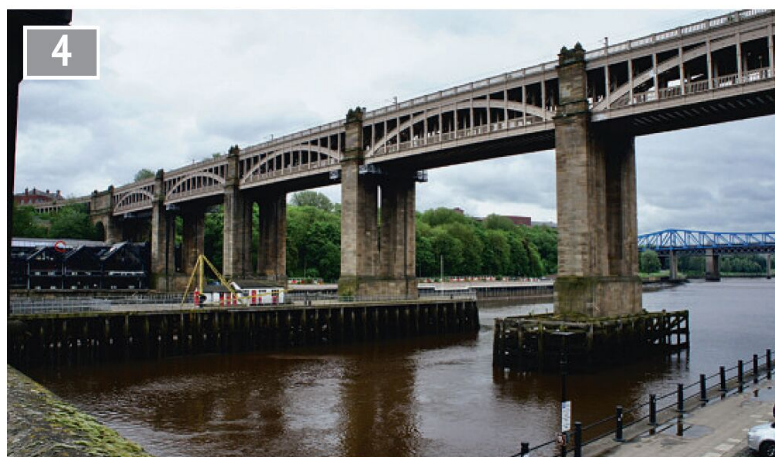
Robert Stephenson's remarkable High Level Bridge seen from the riverside.
