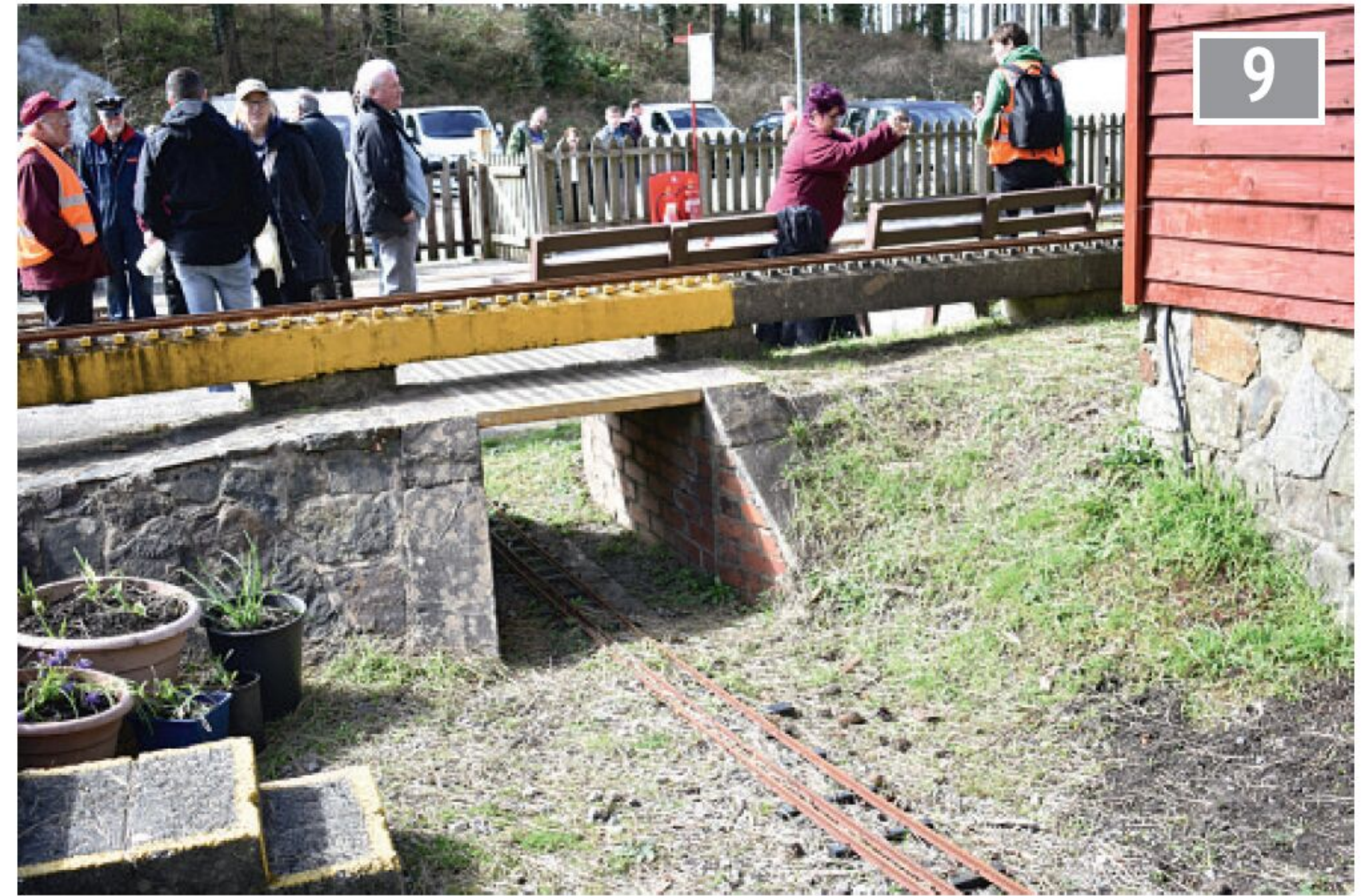
The short tunnel under the raised track for ground level access from the unloading area.
