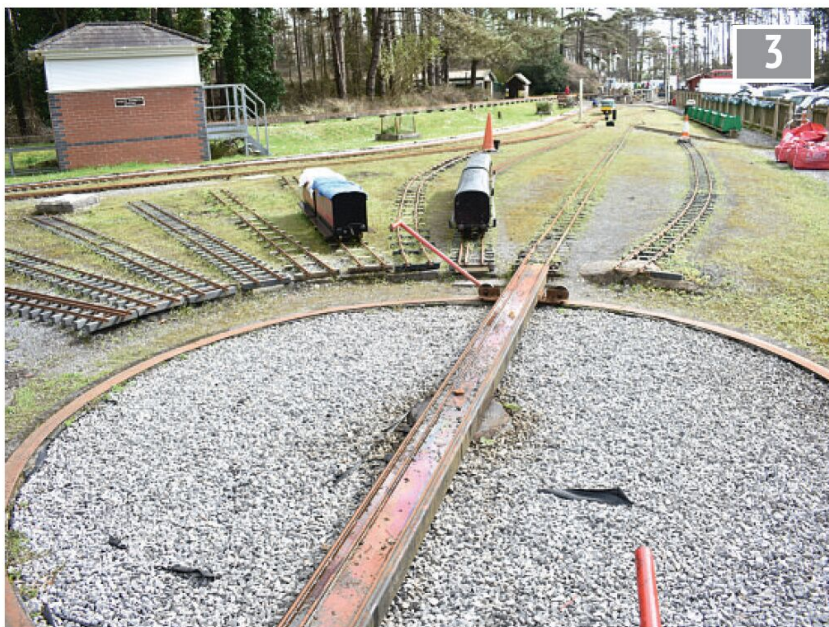
The access line from the turntable to the main station.
