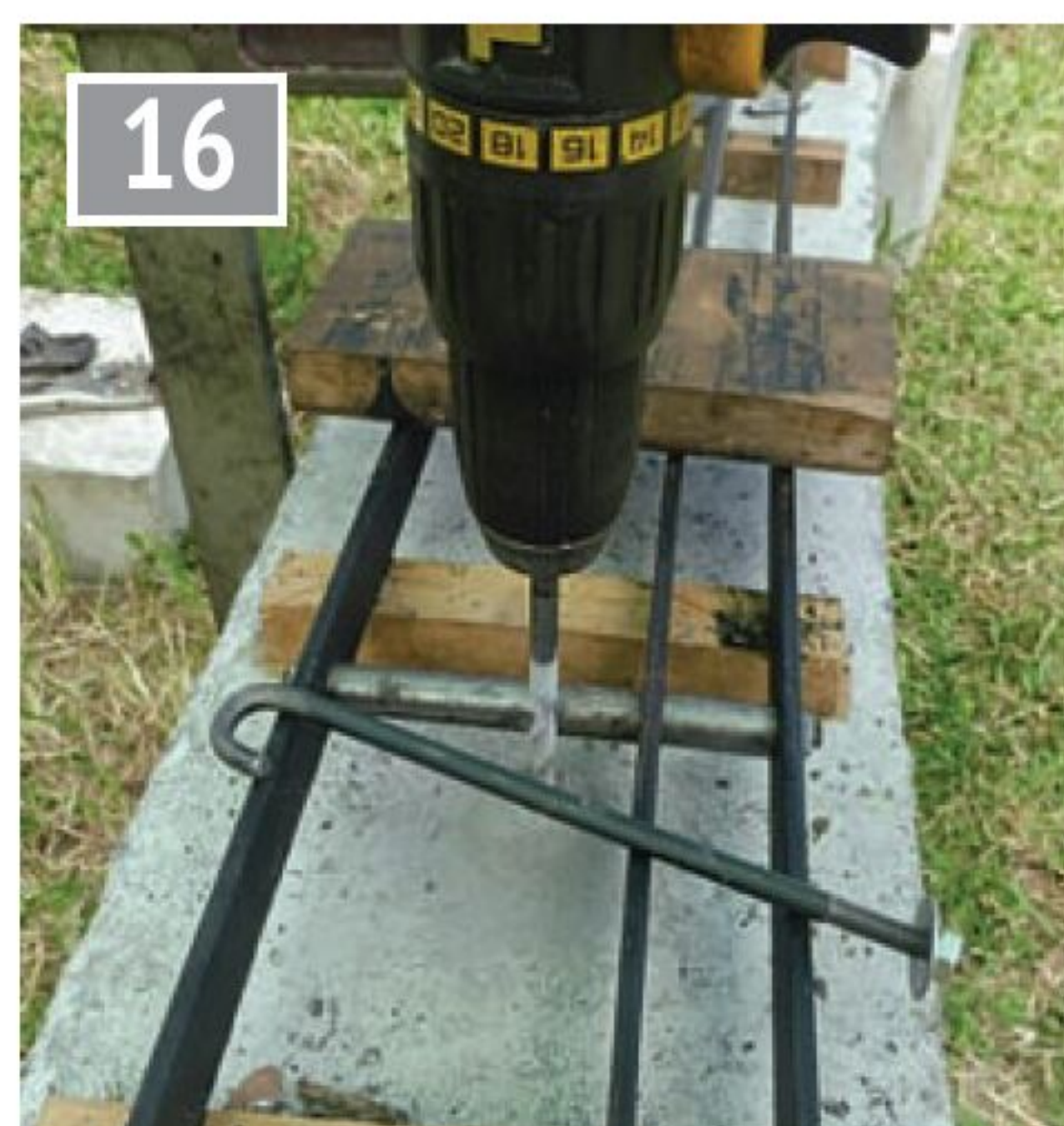
Drilling for the hook bolts.
