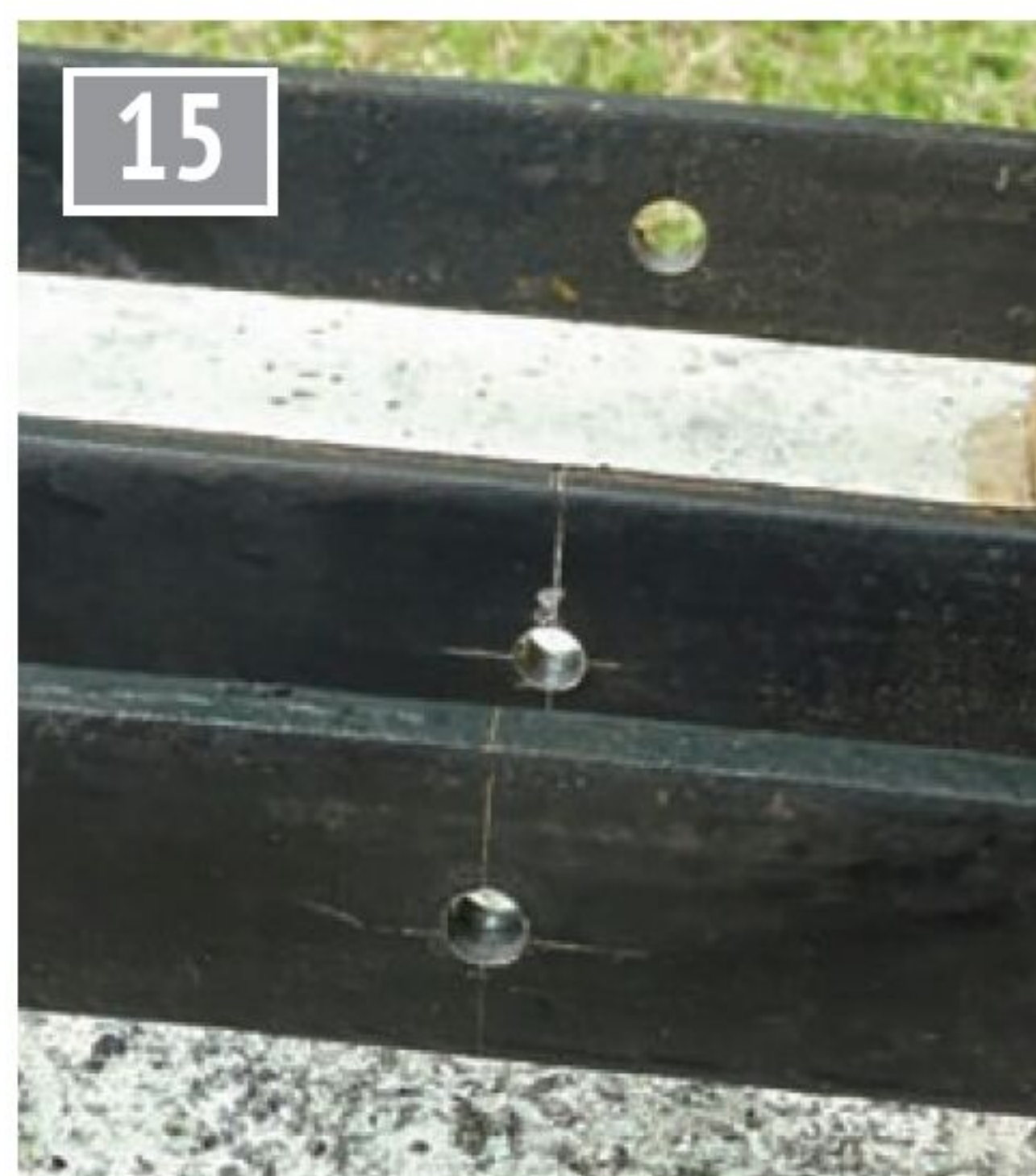
Tie bolt holes spotted and drilled through.
