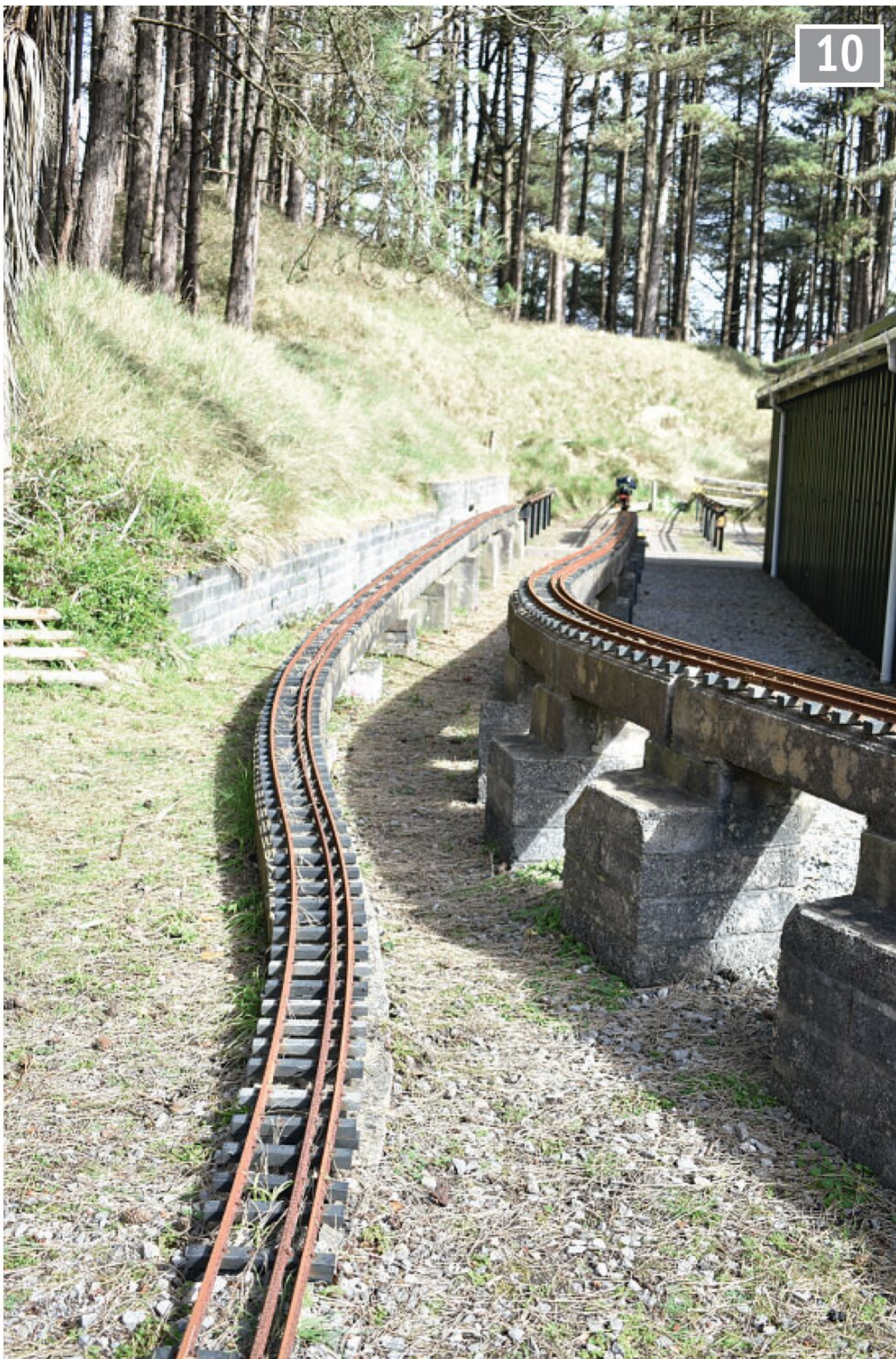
The access track to the raised track steaming bays with the main line access track alongside.
