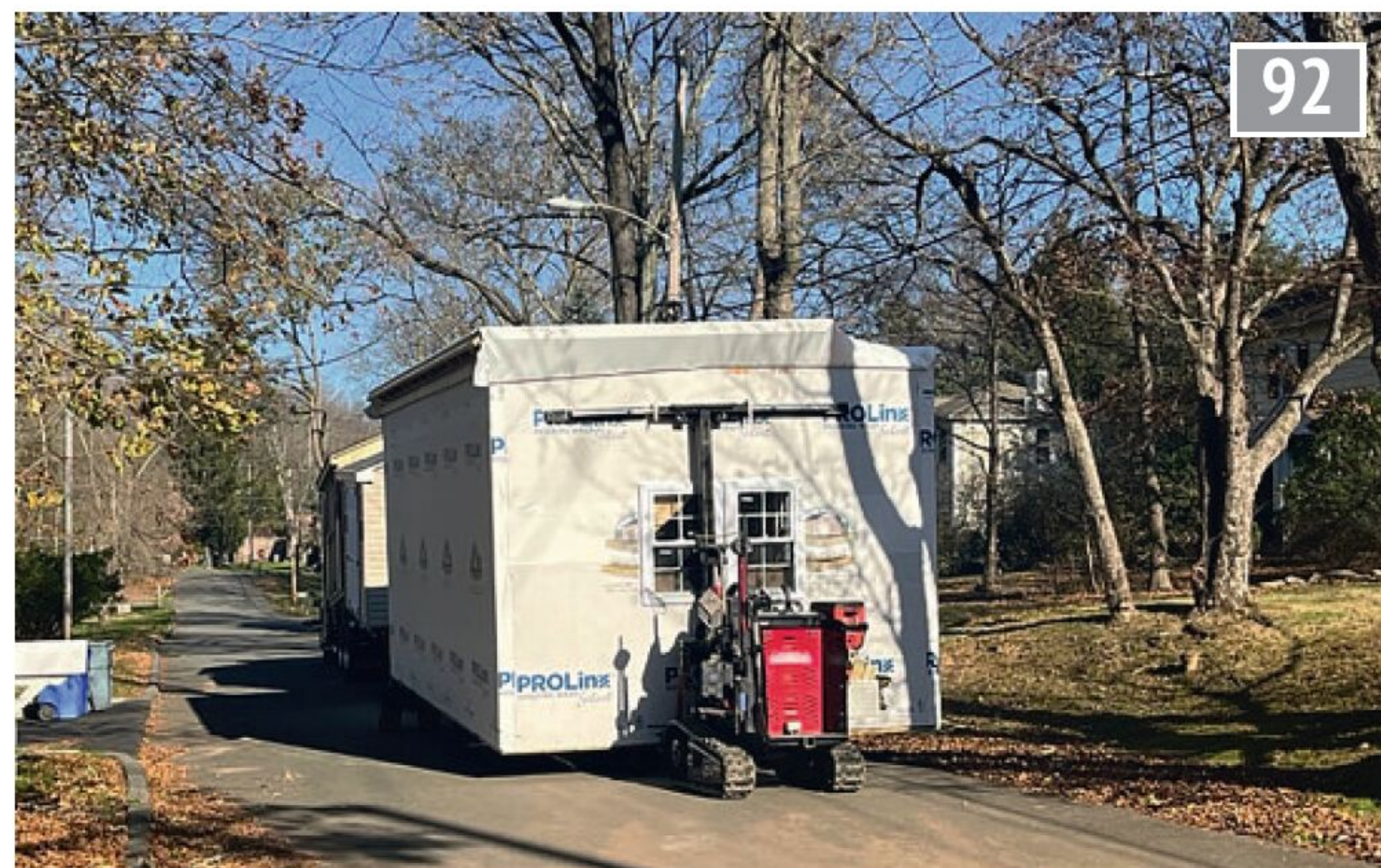
The mechanical mule draws the shed from its trailer, improbable antennae spread wide.
