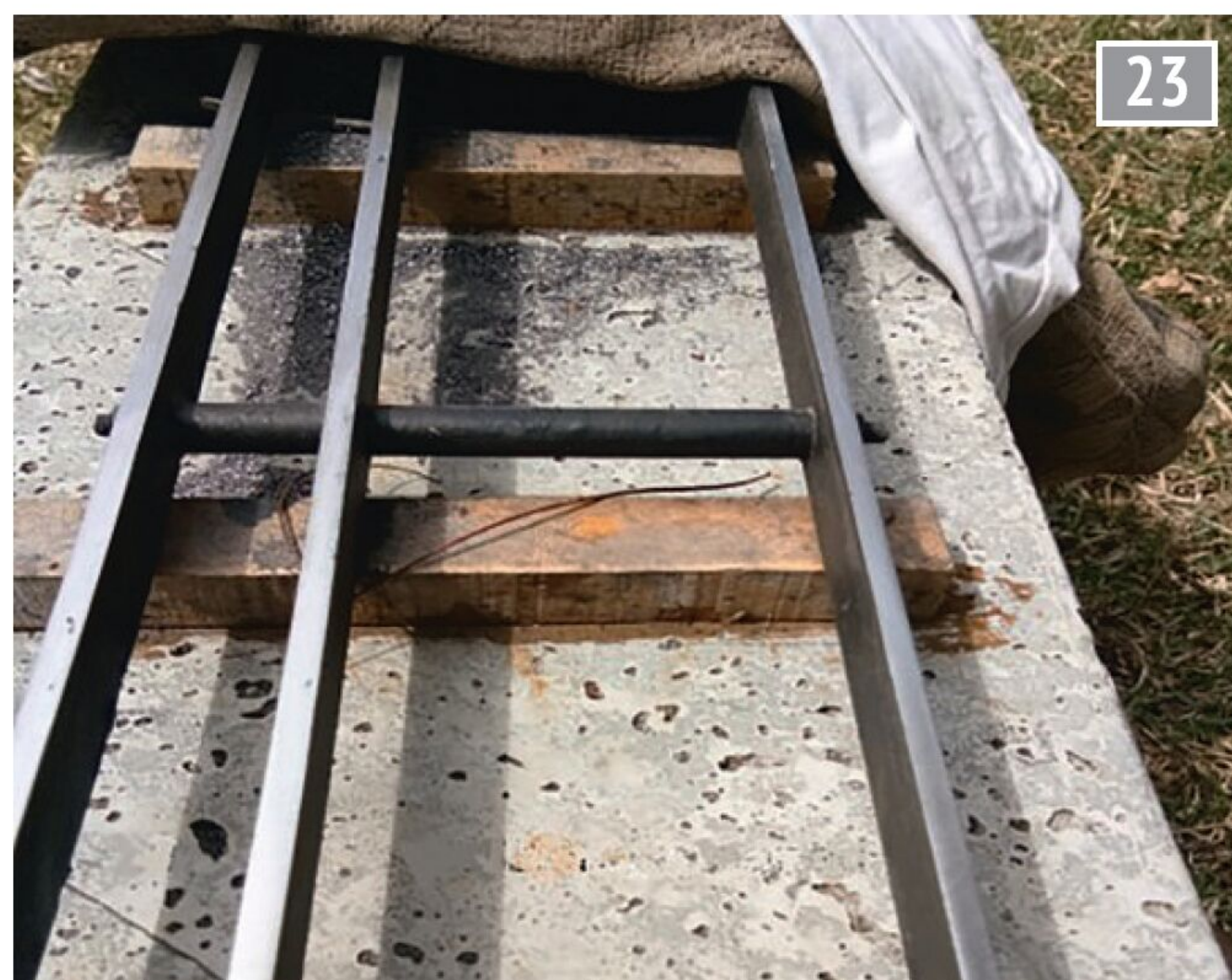
Railhead after cleaning.
