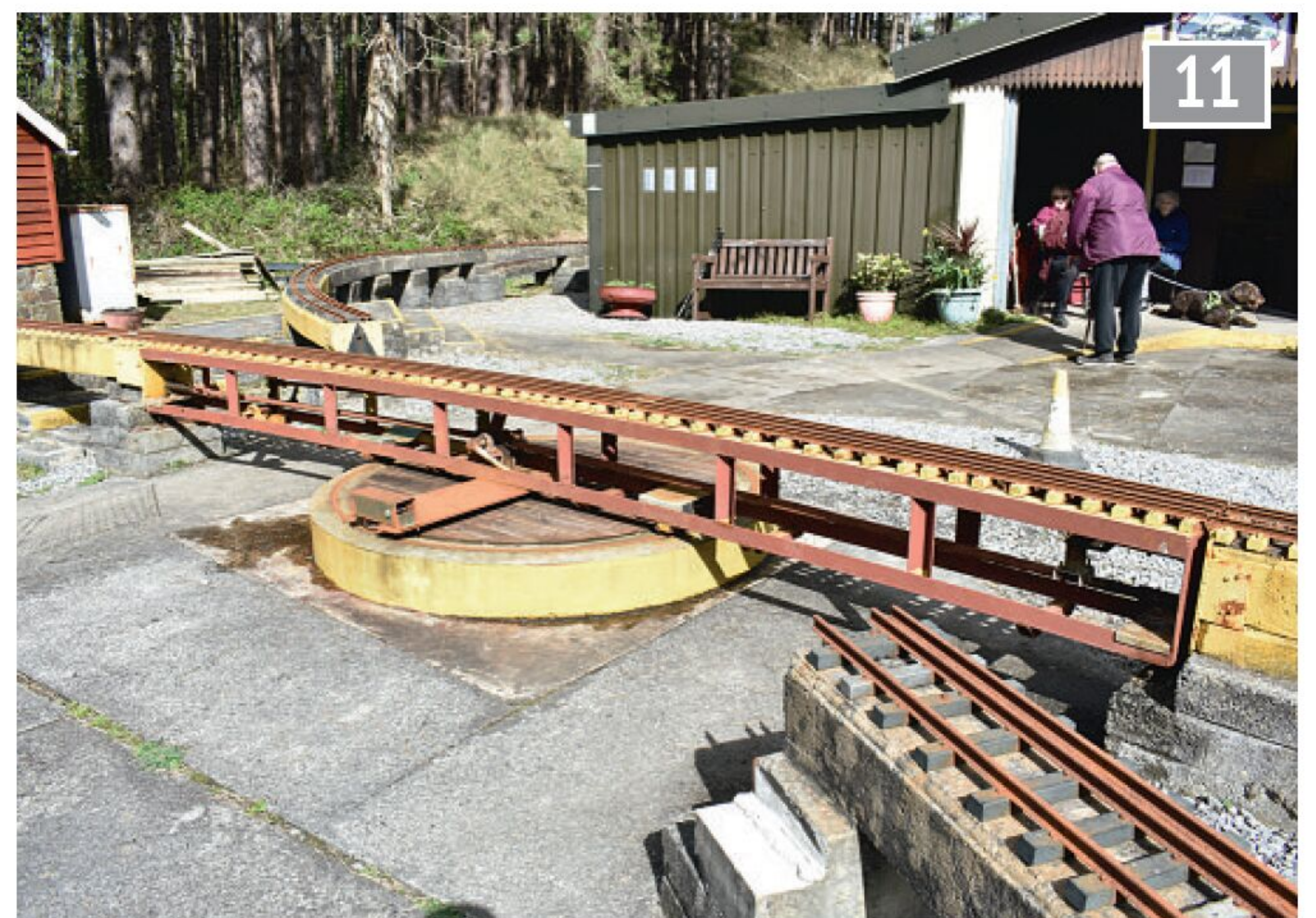
A view of the main raised track movable bridge which gives access to the clubhouse and raised track.
