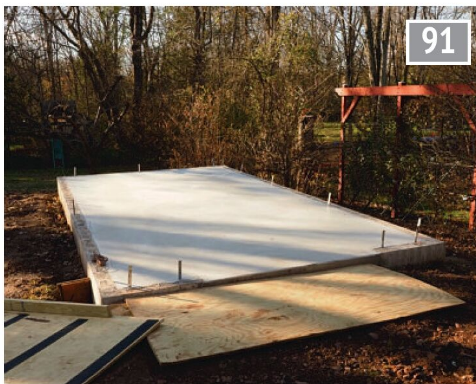
Two weeks later and the foundation is ready for the shed's imminent arrival.
