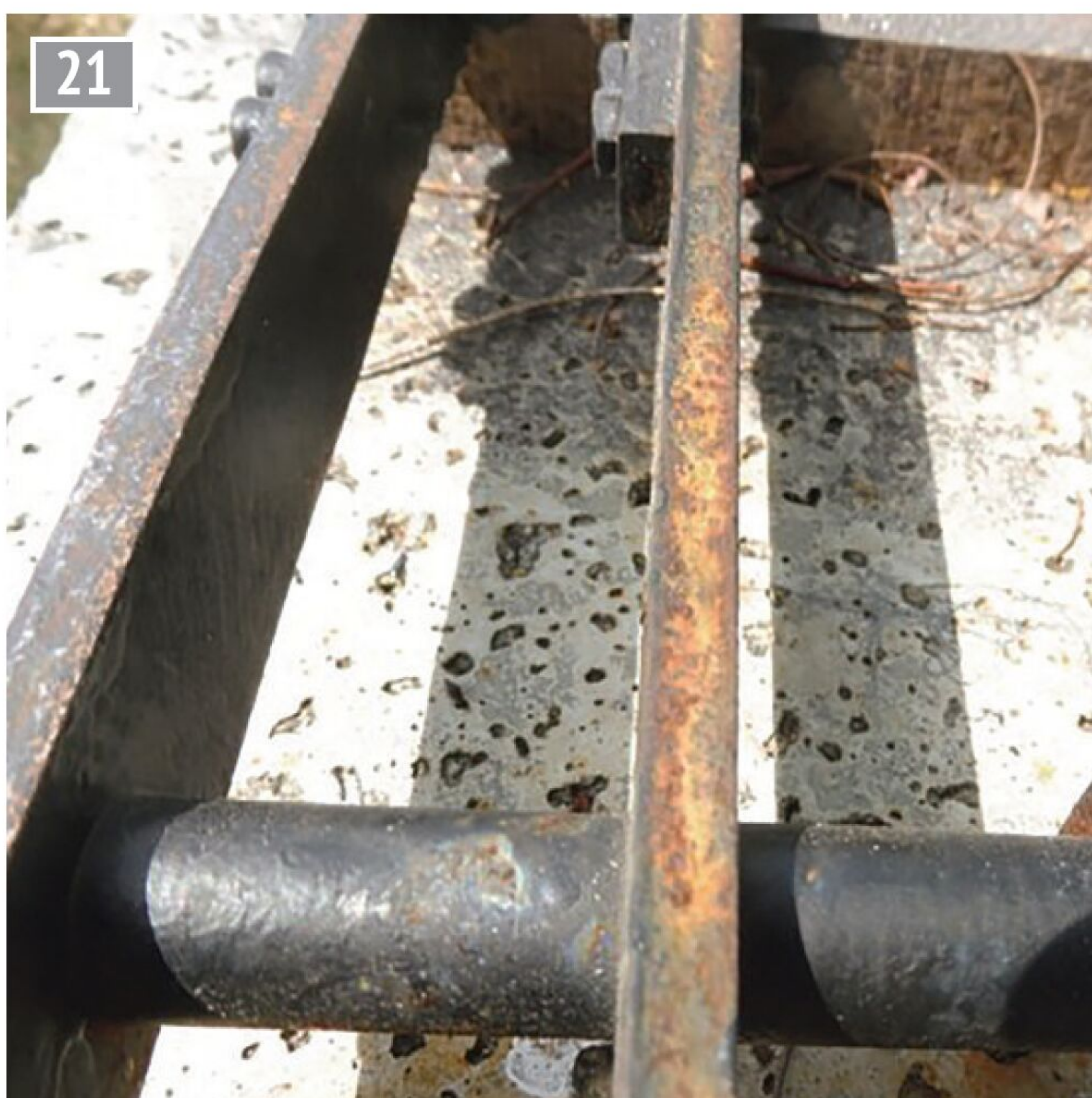
Railhead before linishing.
