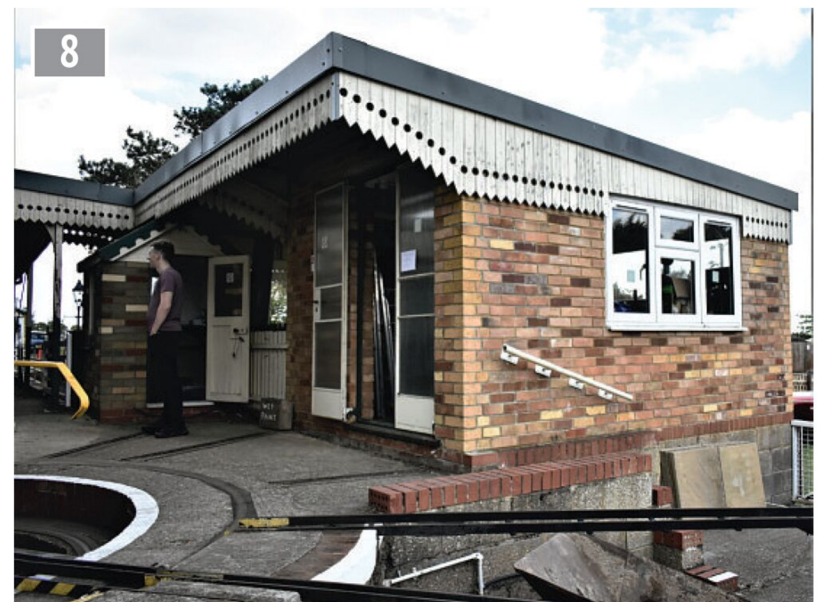
The Station Building at Hayes End.
