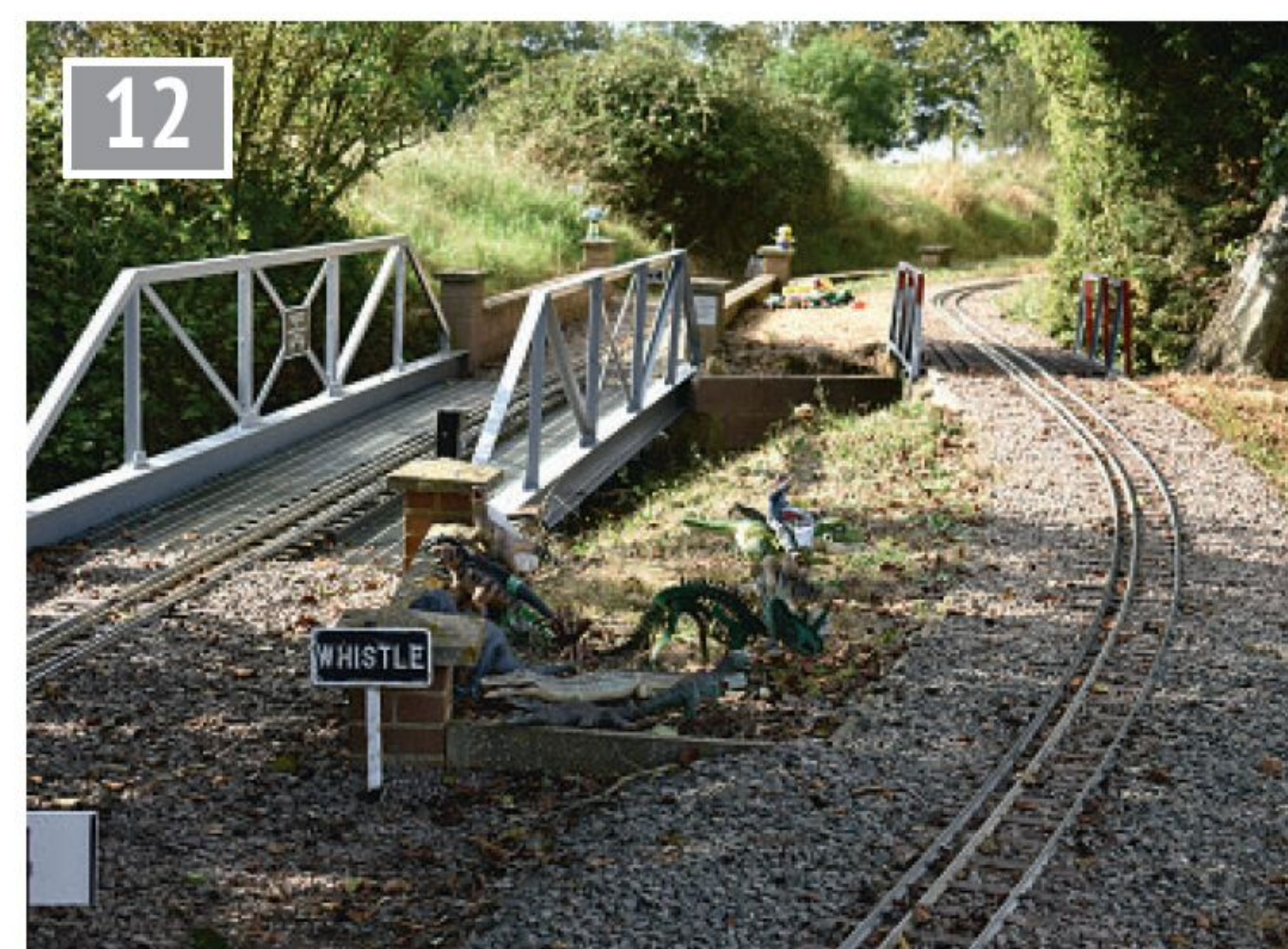
Both main lines with their arrangement of bridges.
