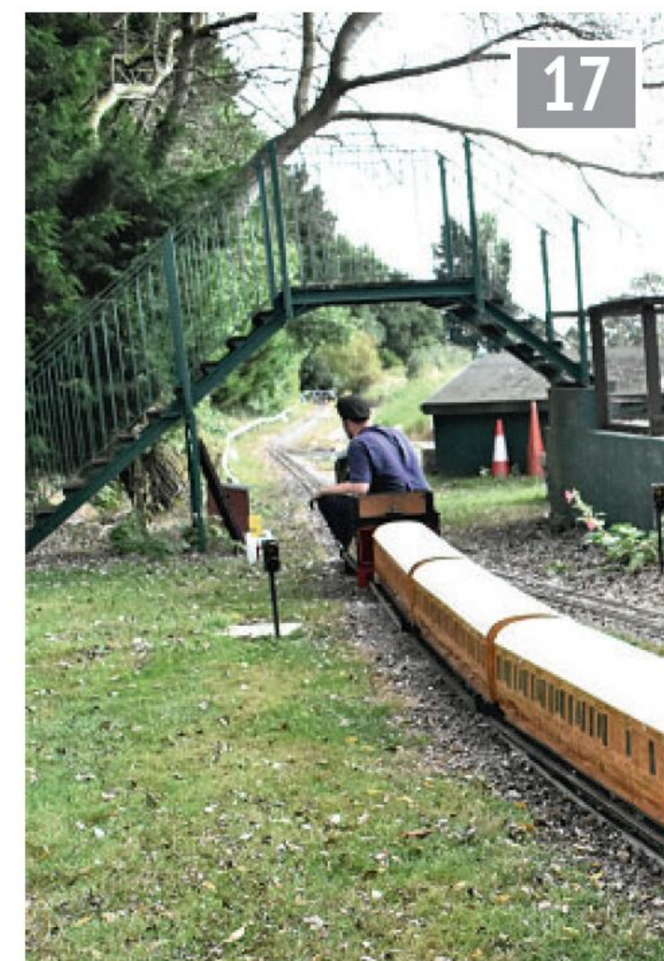
The small additional footbridge giving access to the ground level storage shed and viewing area.
