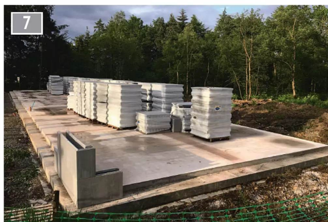
ICF construction was like building with lego.
