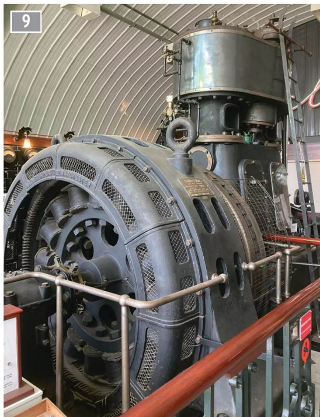
Three phase electrical generator.
