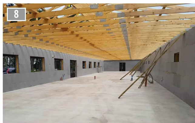
The building taking shape.
