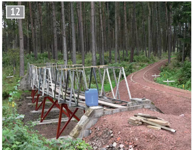
Bridges and embankments.
