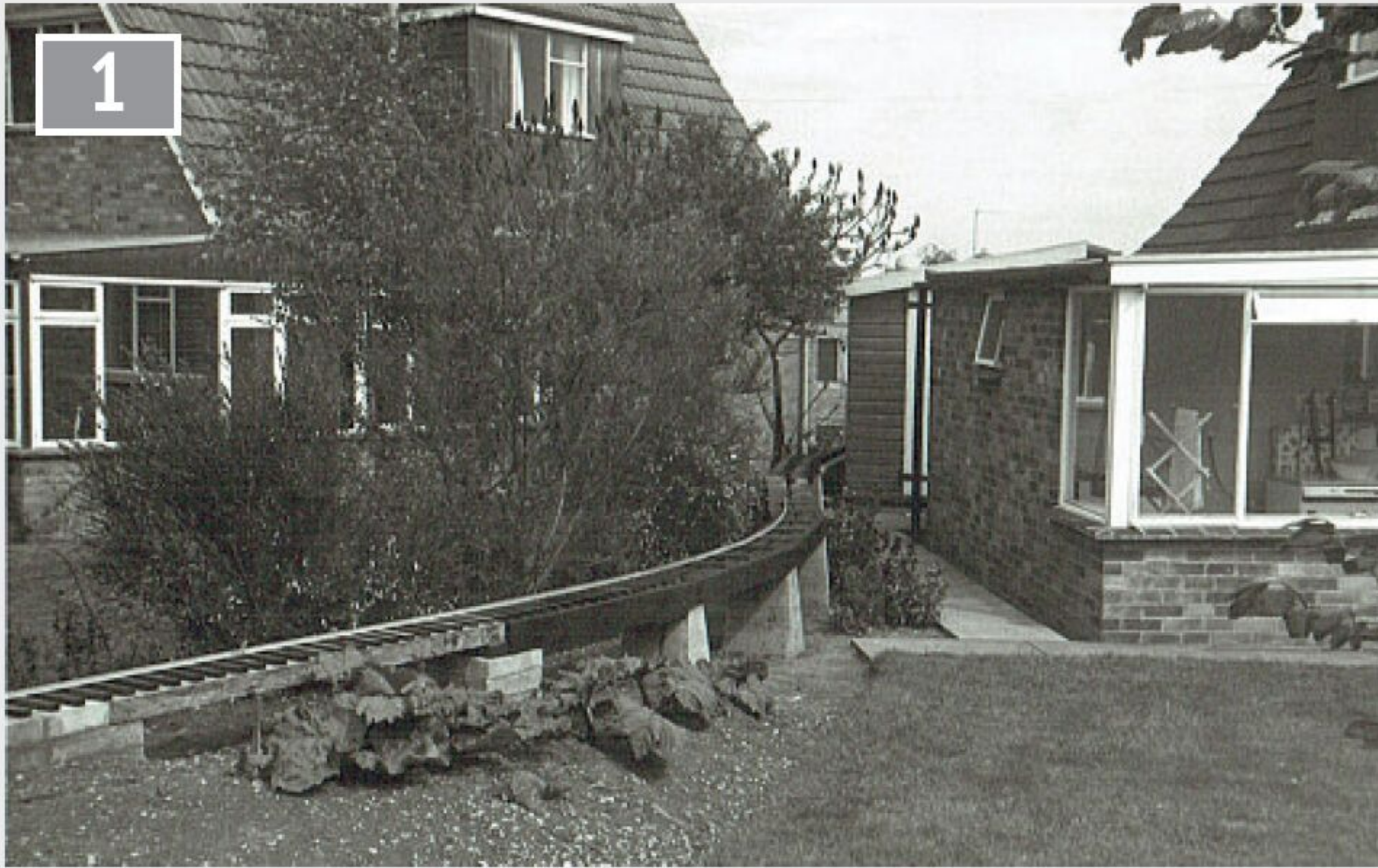
Two views of the lower end of the track leading to the workshop, where the track was laid on discarded house timbers.
