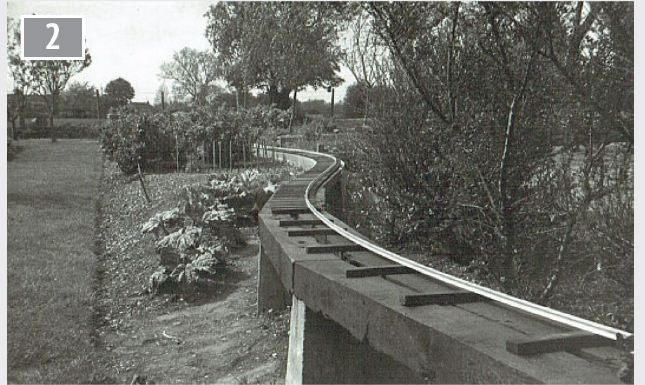
Two views of the lower end of the track leading to the workshop, where the track was laid on discarded house timbers.
