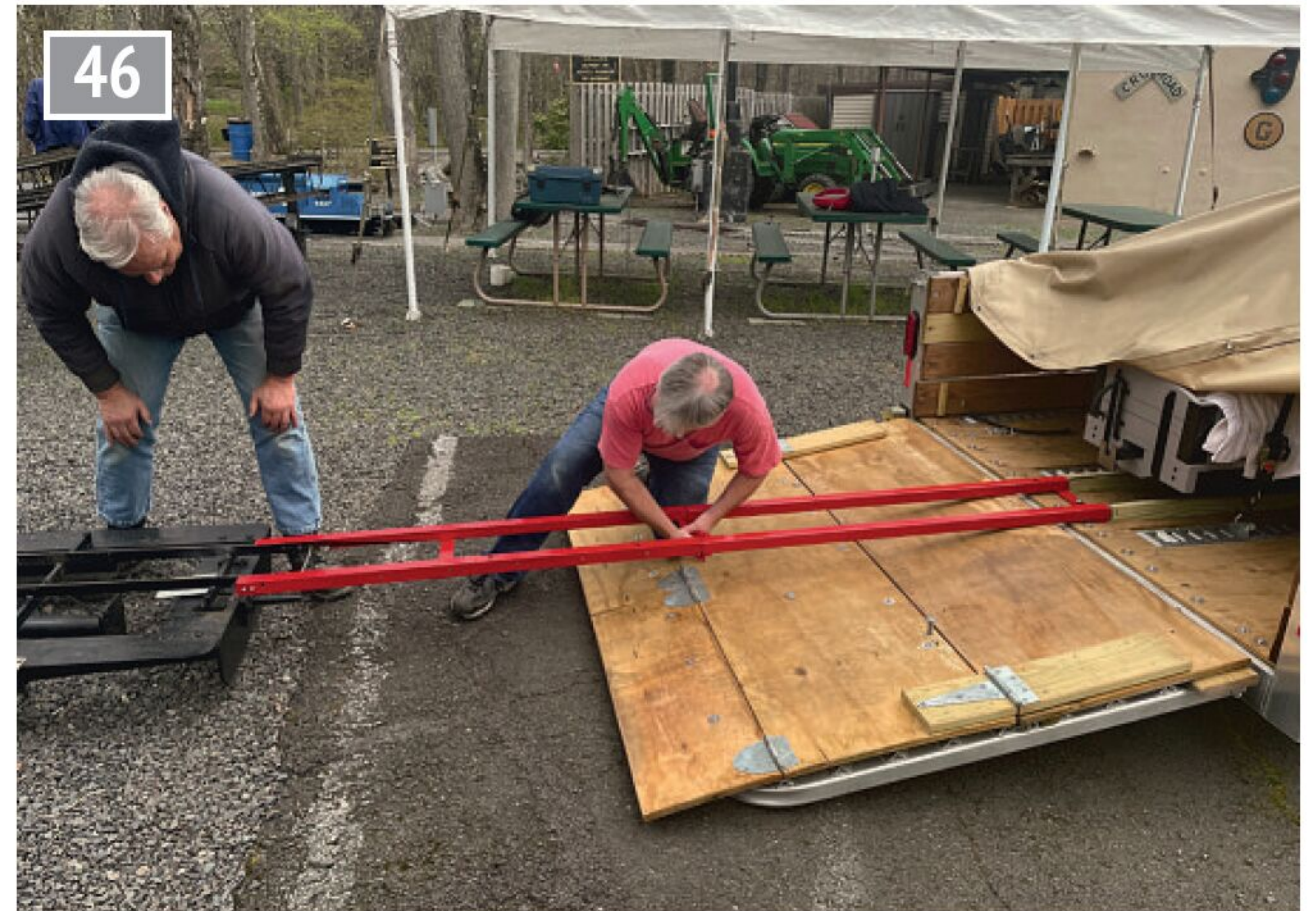
46 With the trailer positioned the correct distance from the turntable thanks to the tell-tale pole, the assembled railway bridge is laid in place (photo: Helen Munro).
