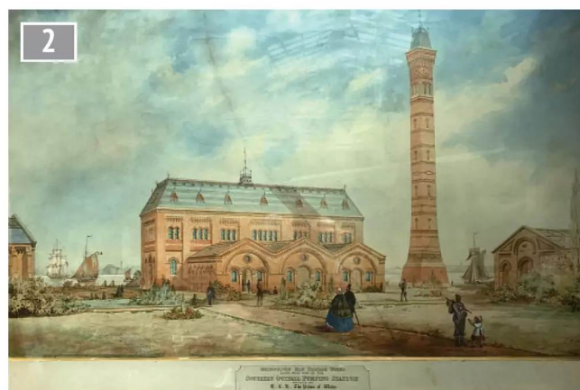
Contemporary view of the pumping station.
