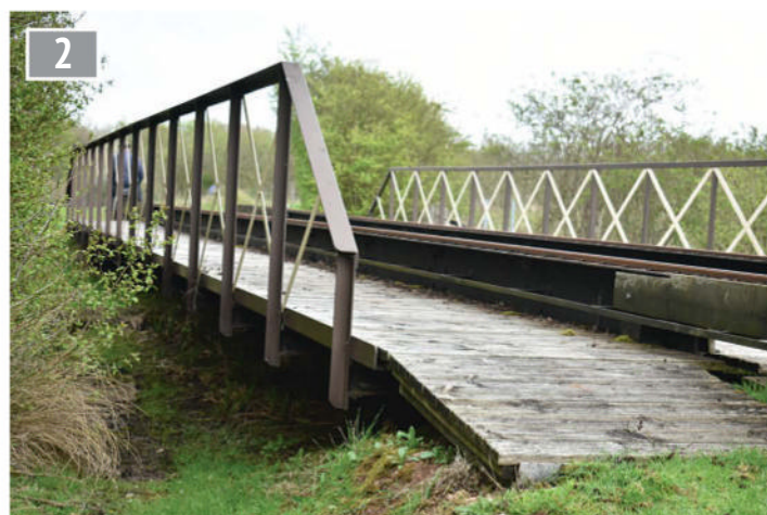
A view of the substantial construction of the girder bridge.
