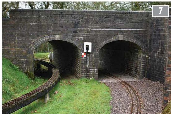
The twin tunnels.
