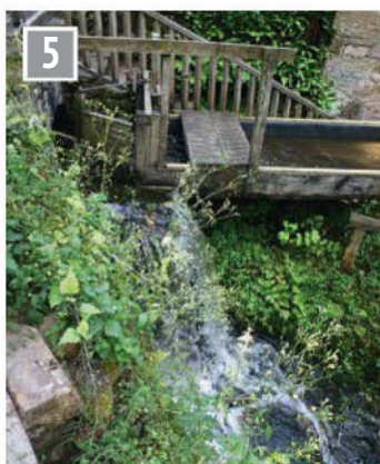
Water flows from the headrace to the launder feeding the mill wheel to the right. The overflow rejoins the Crowdundle Beck.
