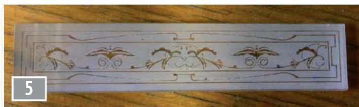
The clerestory windows were laser etched.
