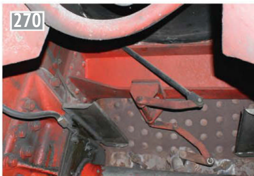
Operating linkage for the blow down valve.
