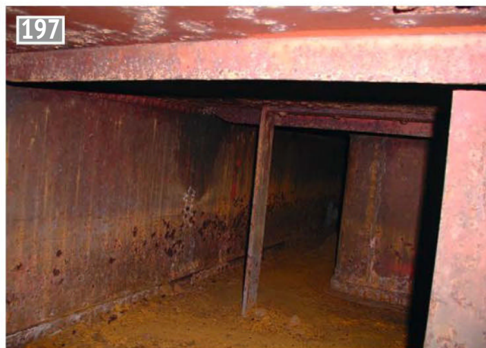
A very rare photograph of the inside of the tender tank; notice the wheel cut-outs to the left of the tank leg.
