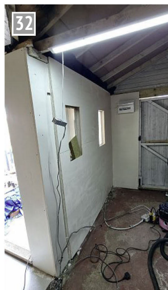
The first section of panelling is complete.
