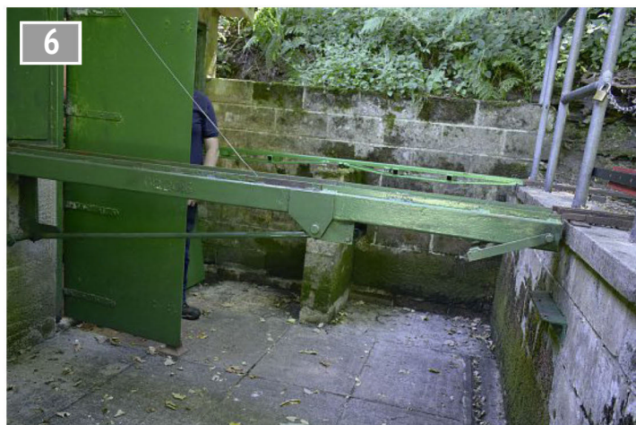
The unique bridge from the storage shed, fully extended and secure for access into the shed.
