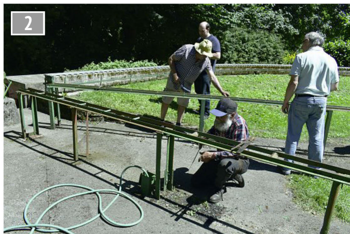
Members busy renovating the raised track steaming bays.
