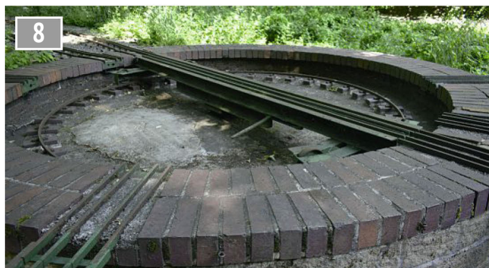
A substantial structure for the ground level turntable.
