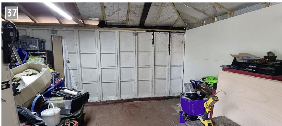
The longest wall is prepared for panelling.
