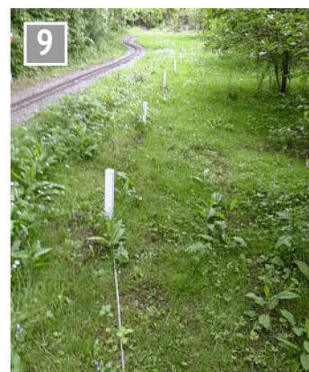
The new raised 3 1/2 and 5 inch track is staked out in the northern extension.
